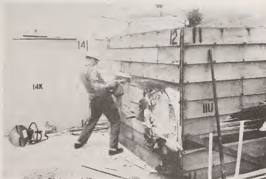
Figure 102. Cutting with Hubless Saw; Test 12
