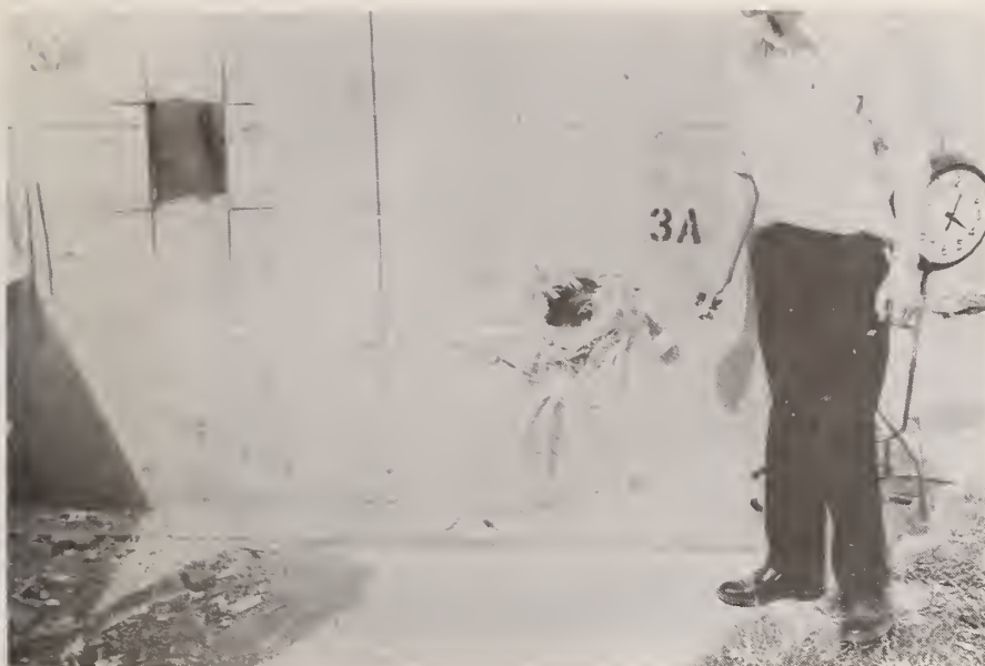
Figure 25. Opening Produced by 6-lb. Chopping Maul; Test 3A
