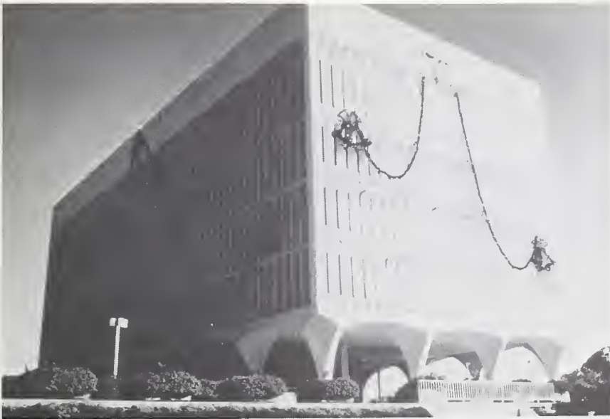
Figure 23-1 Shear wall-frame building with little exterior damage, Edificio Administrativo ENALUF.
