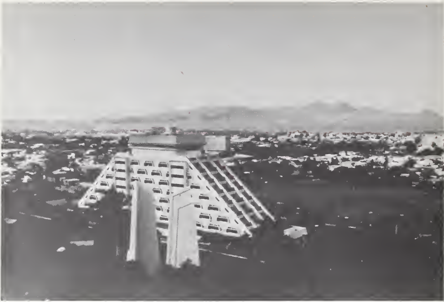
Figure 42-1 General view of Hotel Intercontinental.
