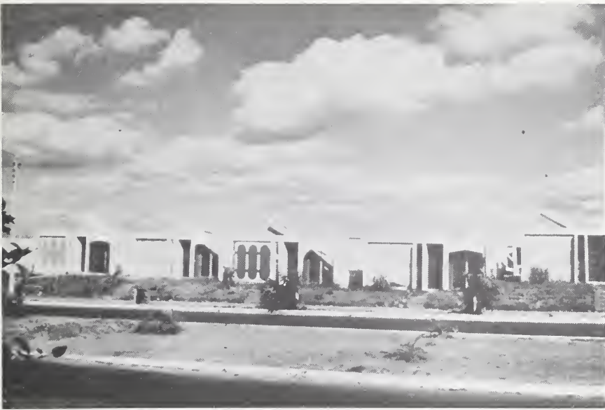
Figure 24-1 The tilted precast roof channels have slid off walls, Bello Horizonte.
