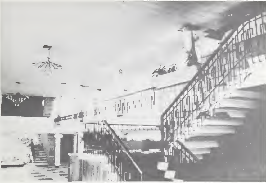
Figure 73-1 Severe structural damage in main building of the Country Club Tejapa.
