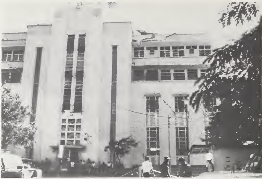
Figure 5-1 Front of the Palacio de Comunicaciones, limited damage except at fourth floor.
