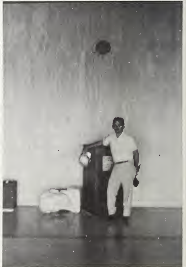
Figure 41-4 Fallen bust of Ruben Dario, Ing. Raul Amador of Nicaraguan Ministry of Public Works, Teatro Ruben Dario.
