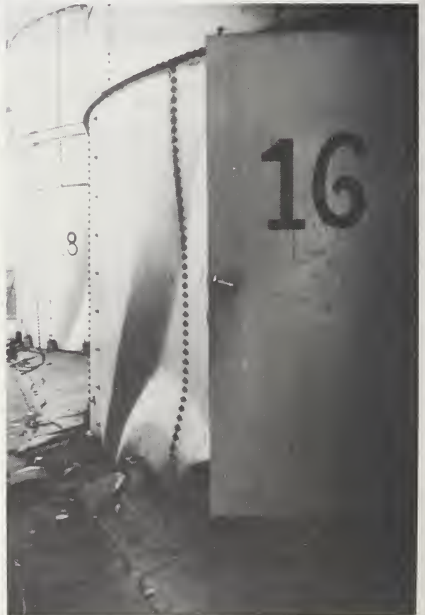
Figure 16-6 Compressive buckling at base of INCEI elevators.
