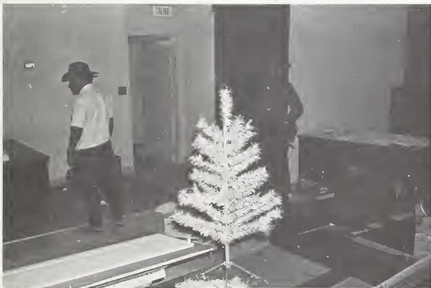
Figure 54-2 Good condition of interior due to control of drift, Banco de America.
