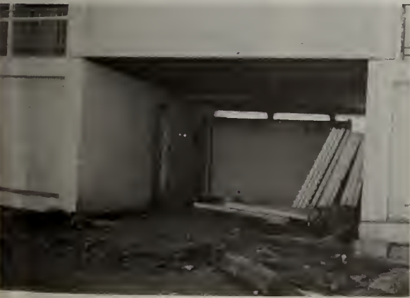
FIGURE 8. Detail of stacking of modules.
