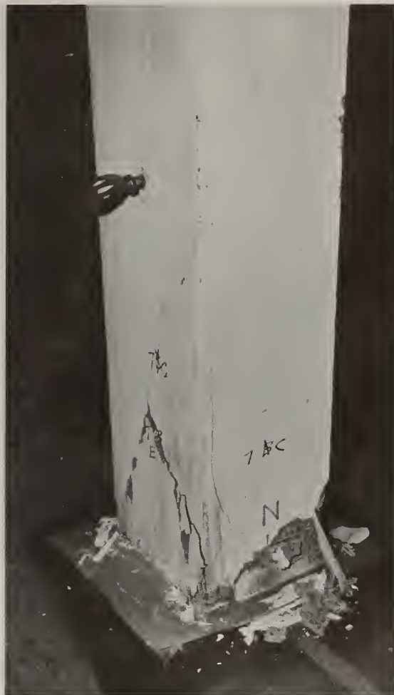
FIGURE 15. Failure of connection with neoprene pads and low friction material.
