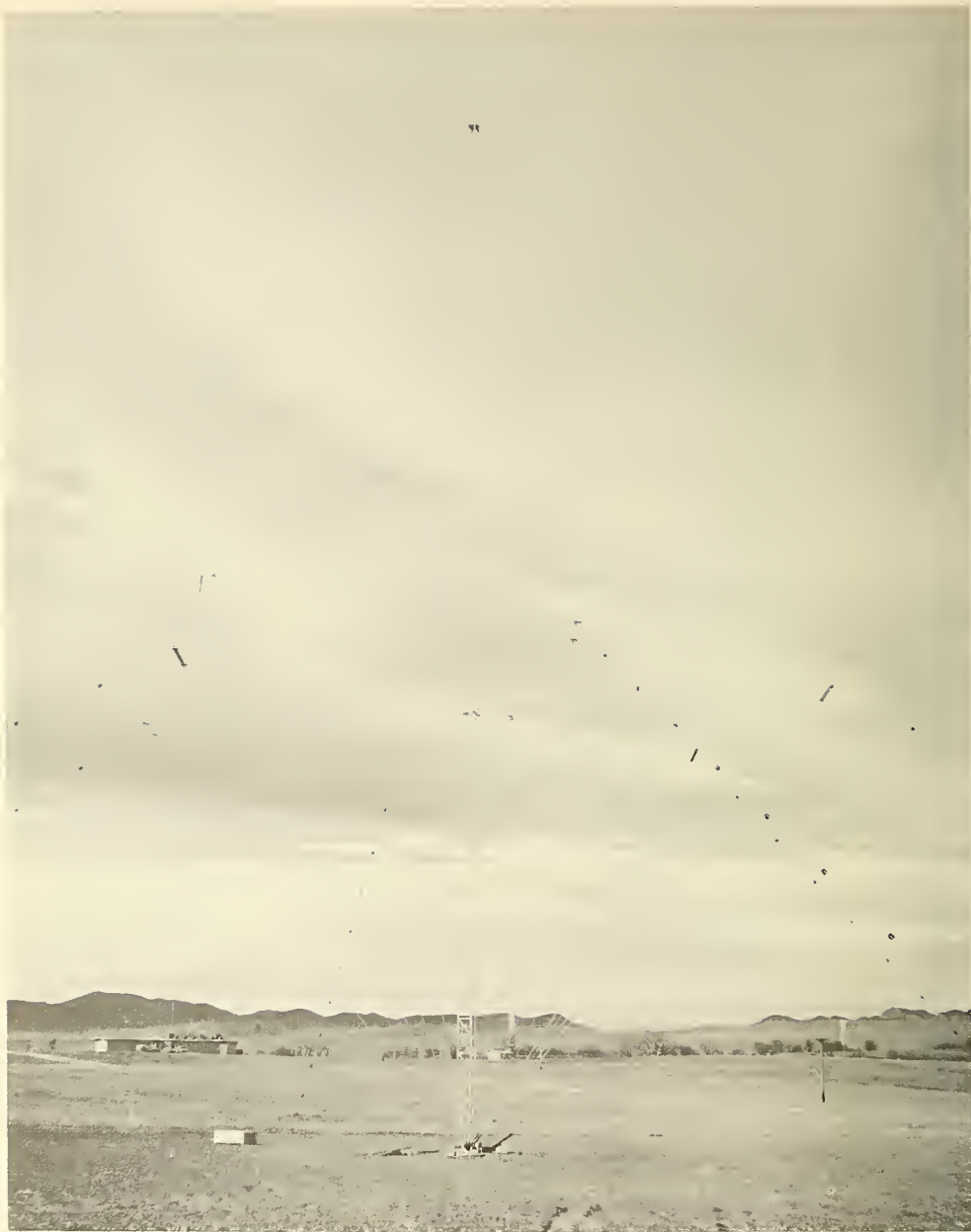
Figure 13. A view of one of the 2.5 - 25 MHz standby antennas.
