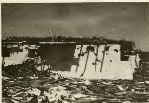
Photograph 56—Damage to a house constructed with stucco-wood frame and roofed with rounded clay tiles. Note bombardment of walls by debris. (Location 31)
