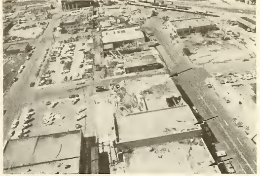
Photograph 36—Roof damage to light industrial buildings. View looking north. (Location 20)
