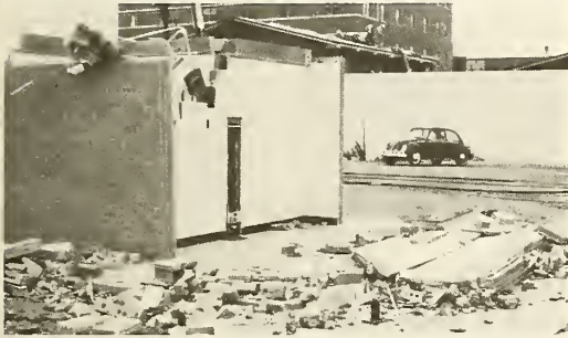
Photograph 16—Small office building for dealer in used automobiles. Roof structure completely removed and non-reinforced masonry walls badly damaged. (Location 9)
