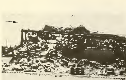
Photograph 41—Destruction of a soft-drink warehouse. View looking west. (Location 24)
