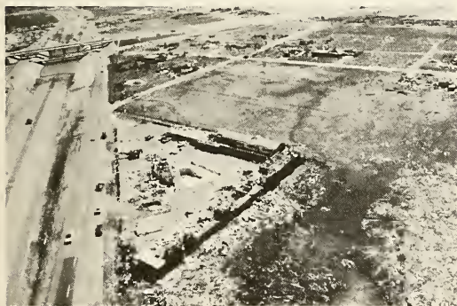
Photograph 44—View looking south over the destroyed two-story Ramada Inn Motel. (Location 27)
