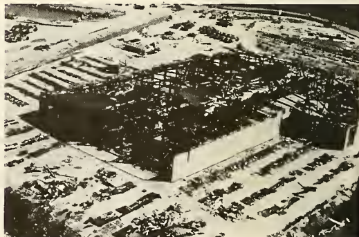
Photograph 43—Clark Equipment Company workshop with stripping of corrugated metal roofing and distortion of the structural steel frame. View looking south. (Location 26)
