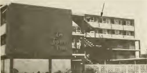
Photograph 27—South elevation of five-story motel with damage to glazing in upper floors. (Location 14)
