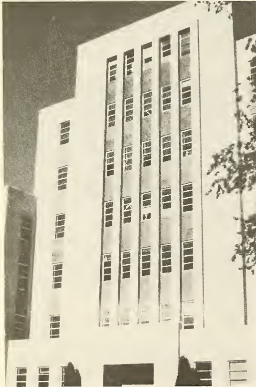
Photograph 33—West elevation of County Court Building suffered only slight glazing damage. (Location 18)
