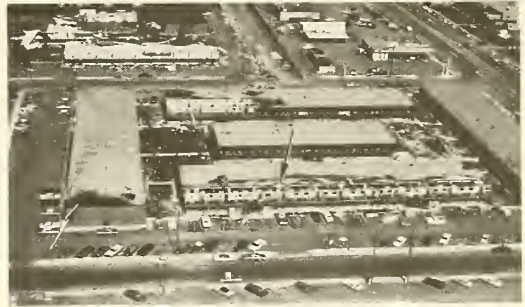
Photograph 2—Apartment complex with “peel-back” of roof membrane and loss of roof overhanging a balcony. View looking east. (Location 2)
