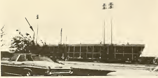
Photograph 3—Jones Stadium of Texas Technological University with bent and collapsed floodlight standards. View looking west. (Location 2)
