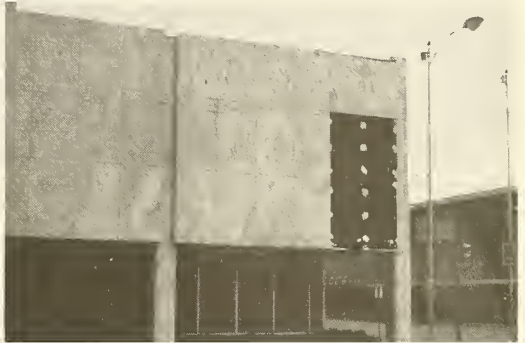
Photograph 19—West elevation of store with loss of marble veneer. (Location 12)
