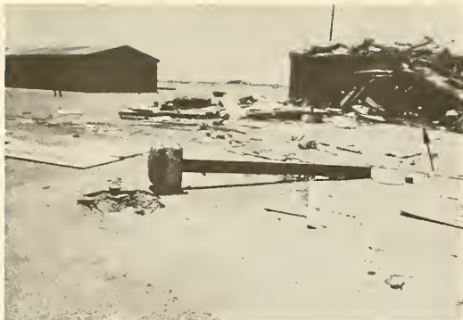
Photograph 61—An overturned steel column is all that remains of several private airplane hangars on the east side of Lubbock Municipal Airport. (Location 33)
