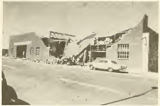
Photograph 18—Maintenance shops of Texas, New Mexico and Oklahoma Coach Company. View looking southwest. (Location 11)
