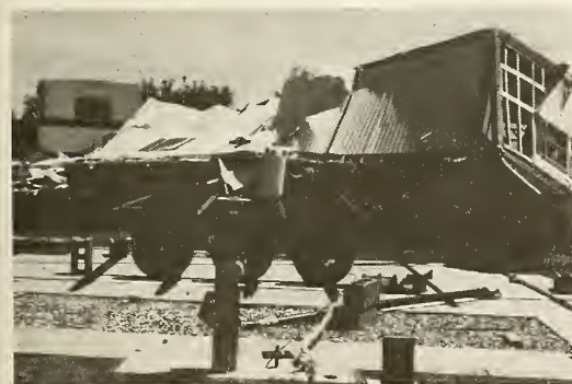
Photograph 58—Mobile home park at Purdue Street with one unit dislodged from its chassis and partly overturned. (Location 32)
