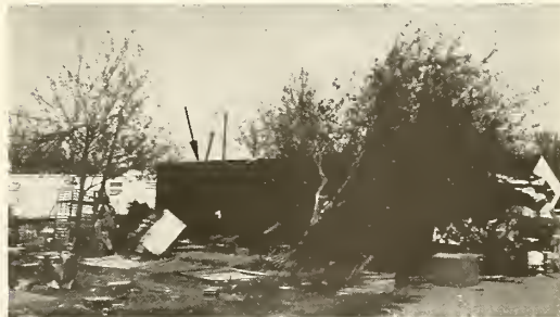
Photograph 52—Several unanchored mobile homes overturned. (Location 30)
