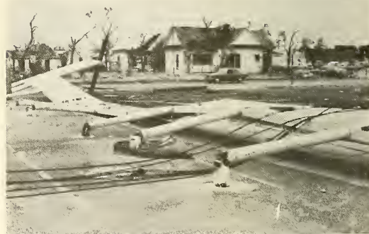
Photograph 14—Damage to sign with tubular steel posts. View looking north. (Location 9)
