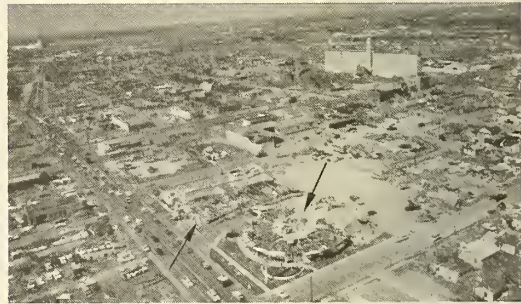
Photograph 6—View looking northeast from center of city. Note destruction of Newsom's Living Center and neighboring buildings in the foreground. (Location 5)
