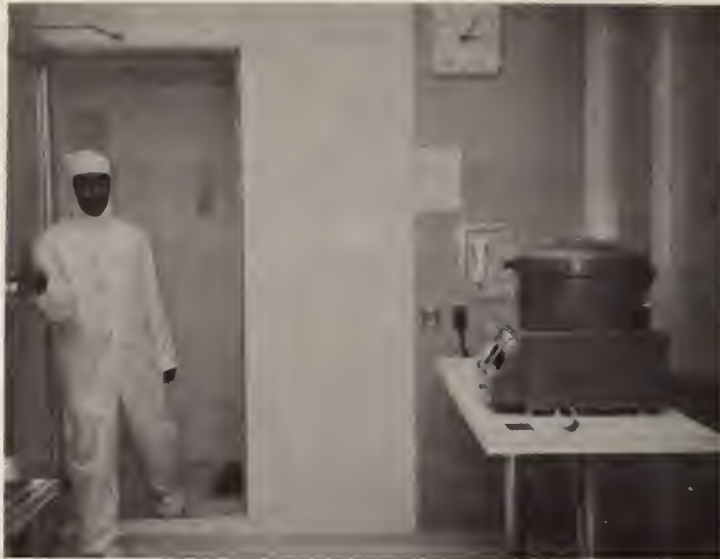
Figure 22. Entrance from the air shower into the class 1000 area.
