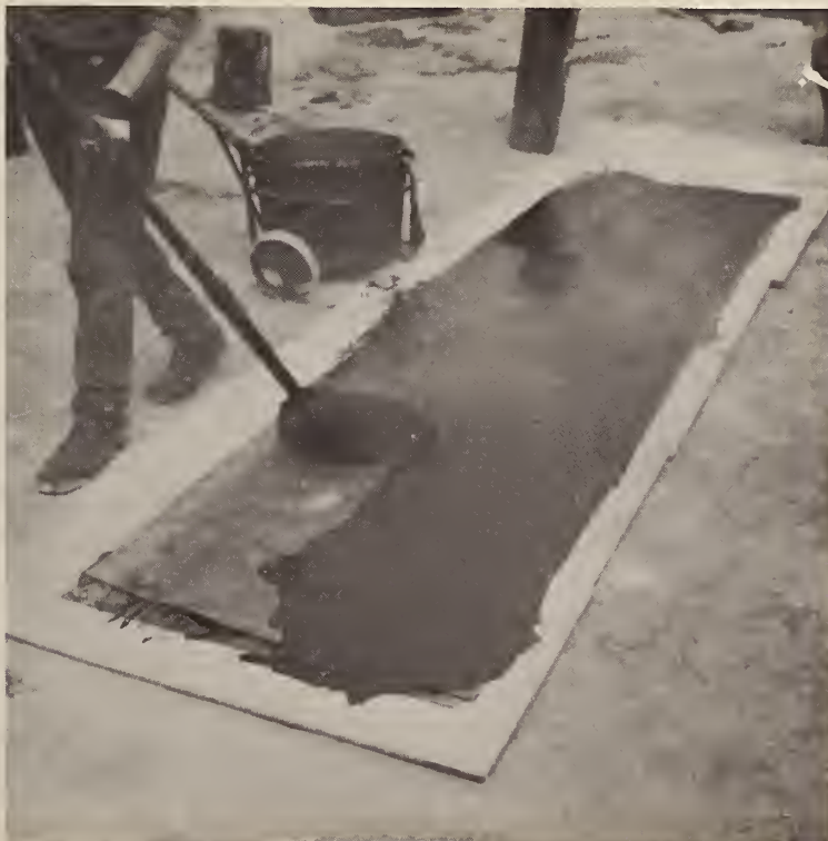
FIGURE 2. Application of hot asphalt to felt.
