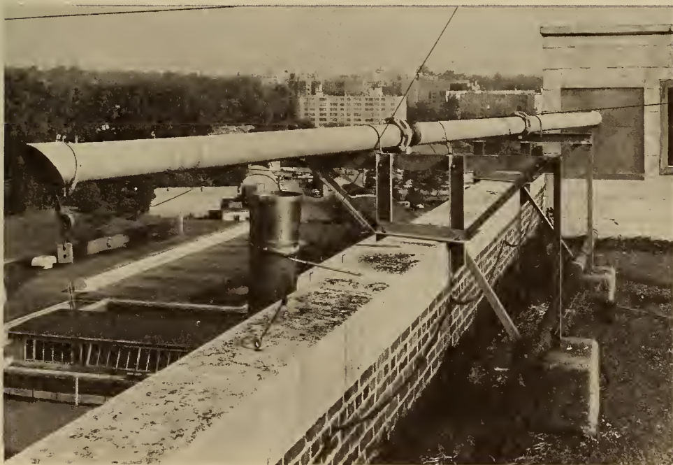
Figure 4B A CLOSE-UP VIEW OF THE BAFFLING TUBE- The front of the tube is covered with a removable protective shield.
