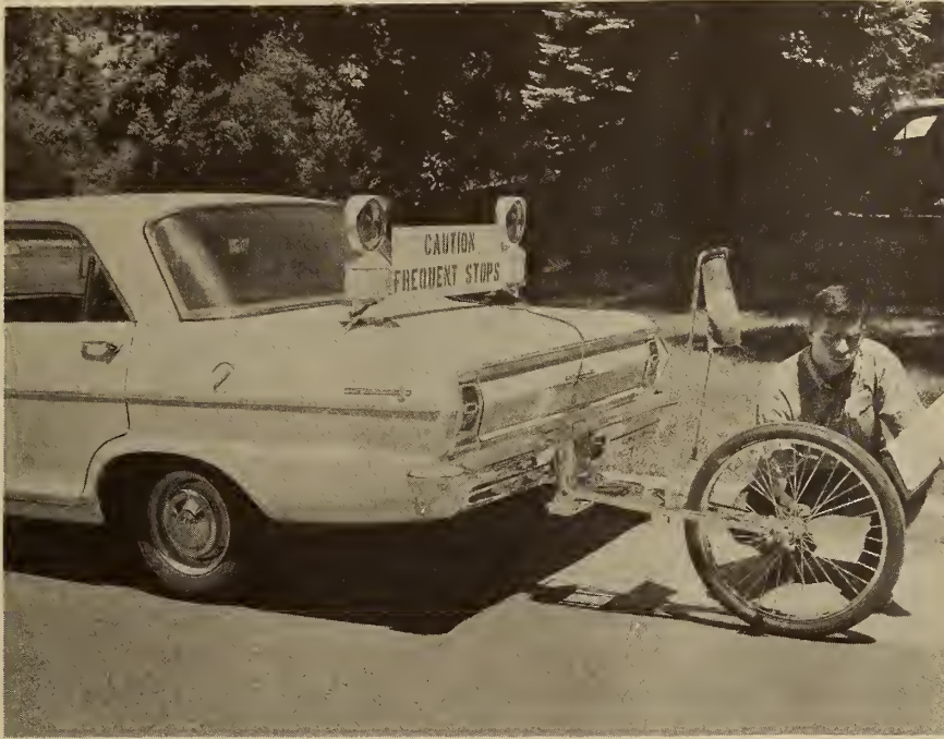
Figure 1. Fifth Wheel in Test Position
