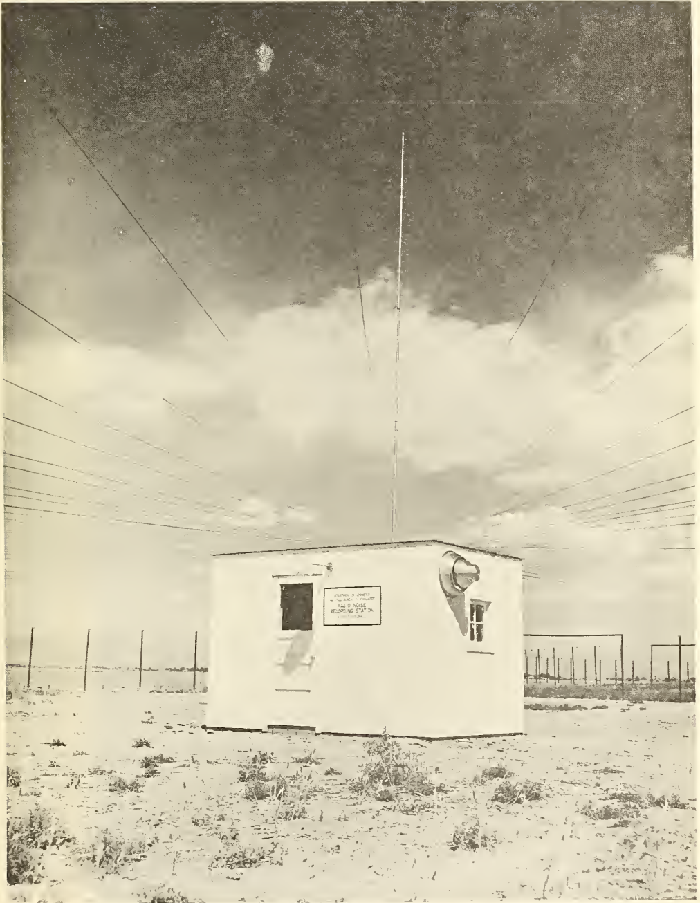
Radio Noise Recording Station
