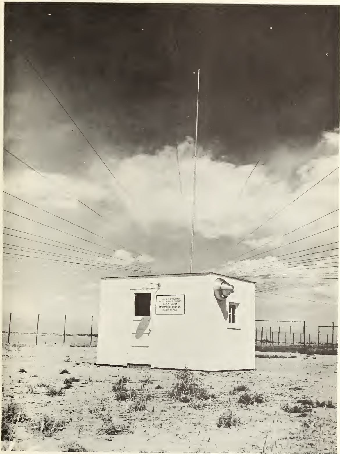
Radio Noise Recording Station
