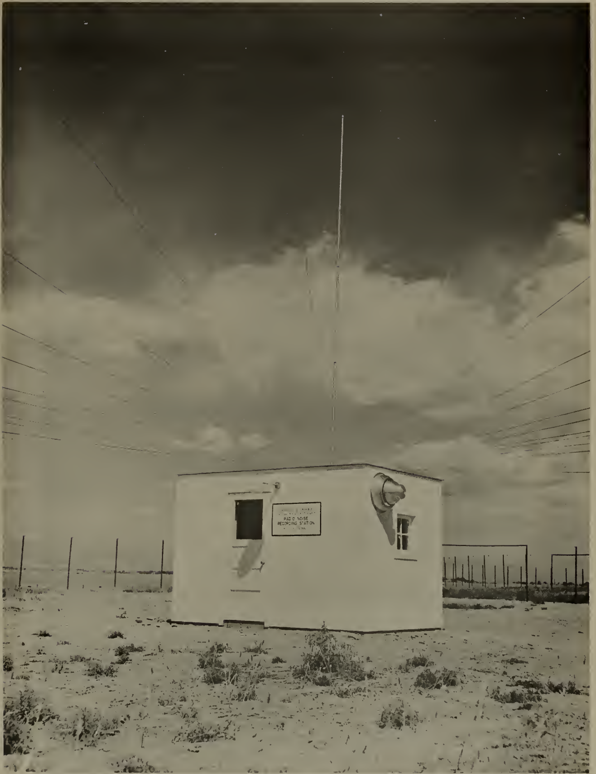
Radio Noise Recording Station
