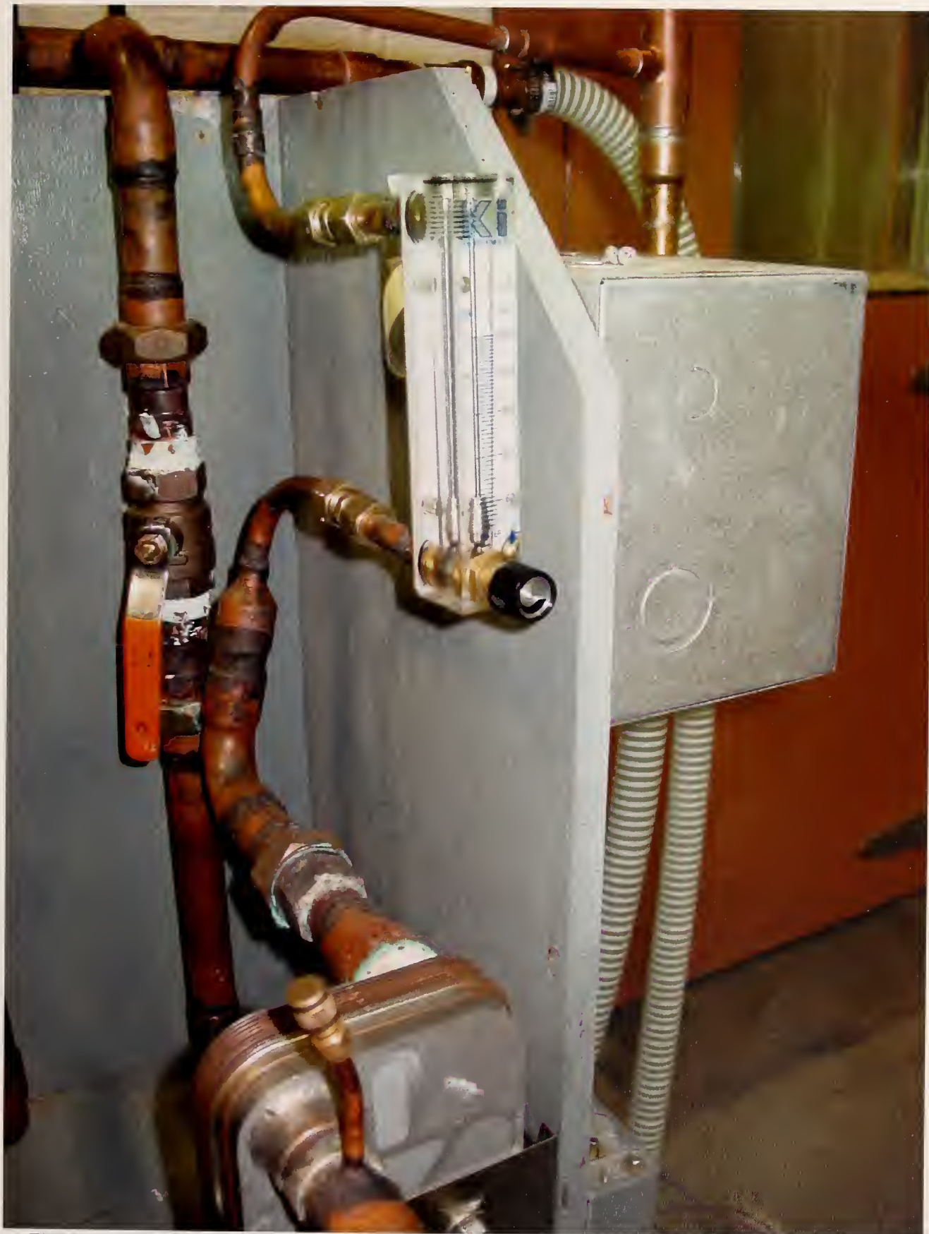
Figure B4: Rotameter/flowmeter used to adjust water flow to subcooler heat exchanger
