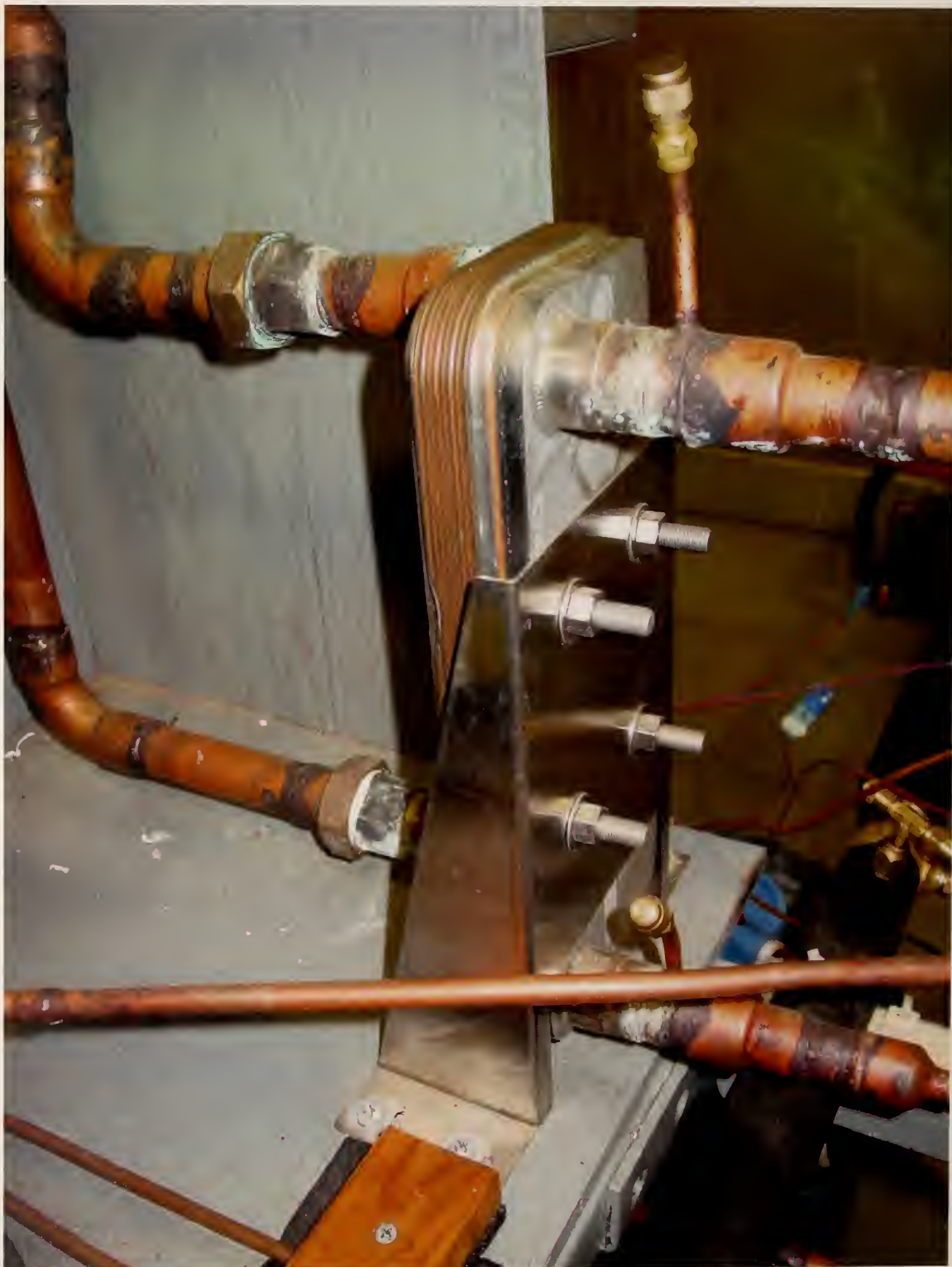
Figure B7: Brazed plate subcooler heat exchanger
