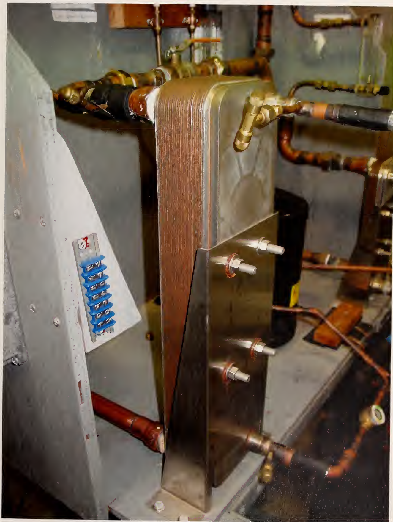
Figure B6: Brazed plate condenser heat exchanger
