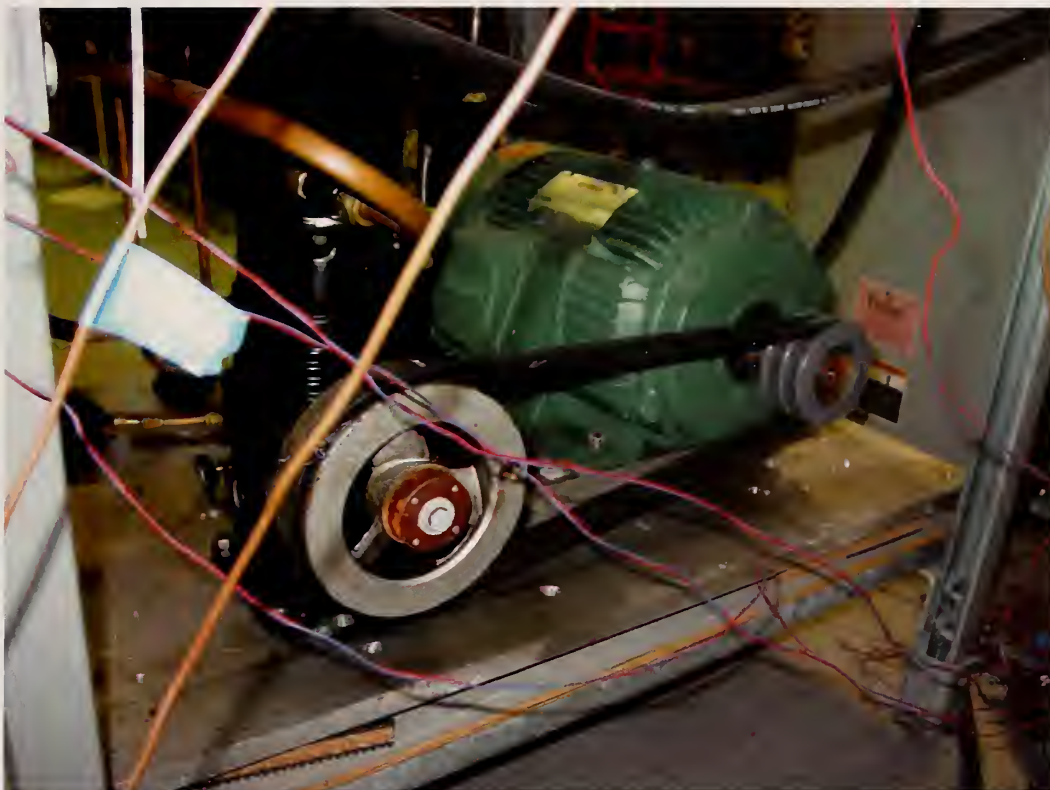
Figure B8: Compressor and motor for water-cooled condensing unit (guard removed)
