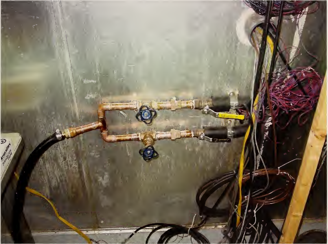
Figure C8: Hot and cold house water mixed before going to water-heated evaporator unit
