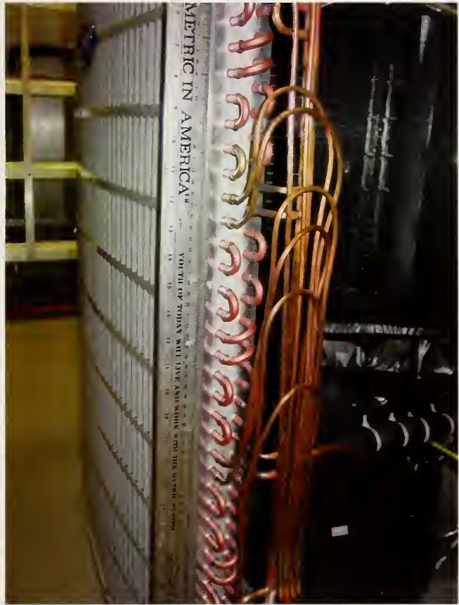
Figure A12: Matched condensing unit coil pictures
