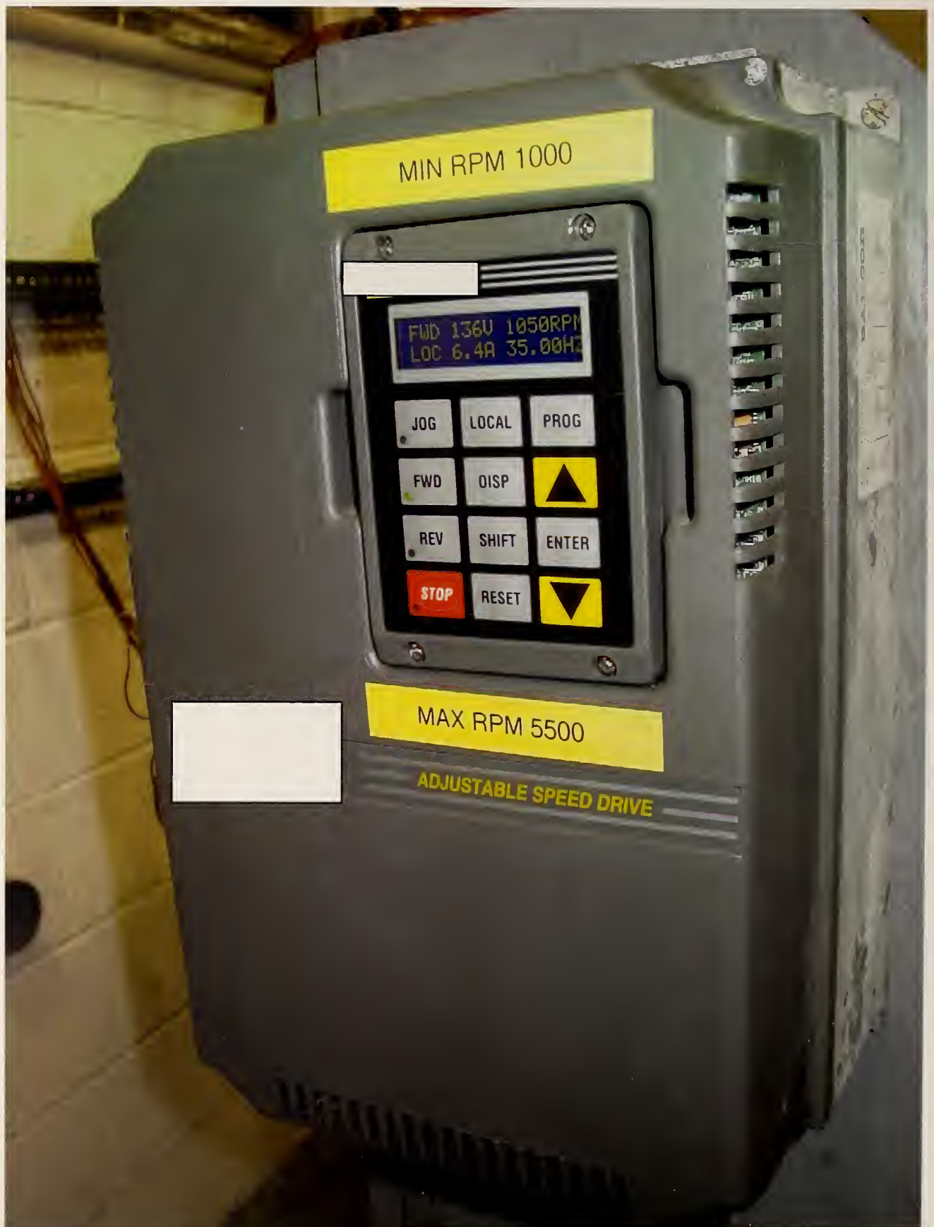
Figure B10: Variable speed drive for water-cooled condensing unit
