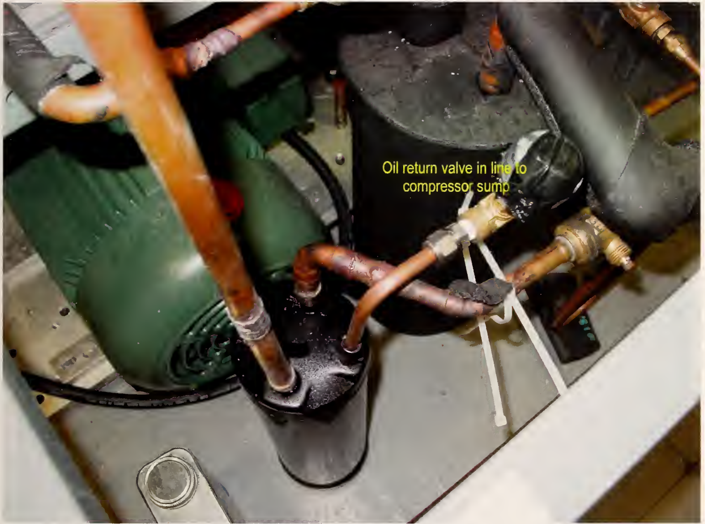
Figure B2: Oil separator arrangement
