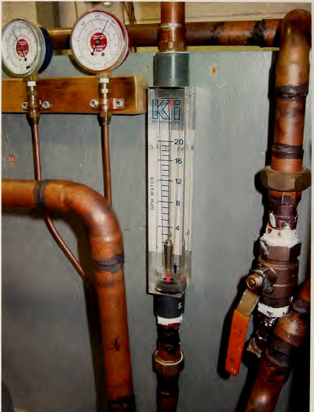
Figure B3: Rotameter/flowmeter used to adjust water flowrate to condenser heat exchanger
