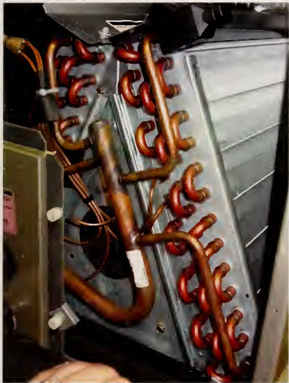
Figure A6: Mixed coil #1 side view
