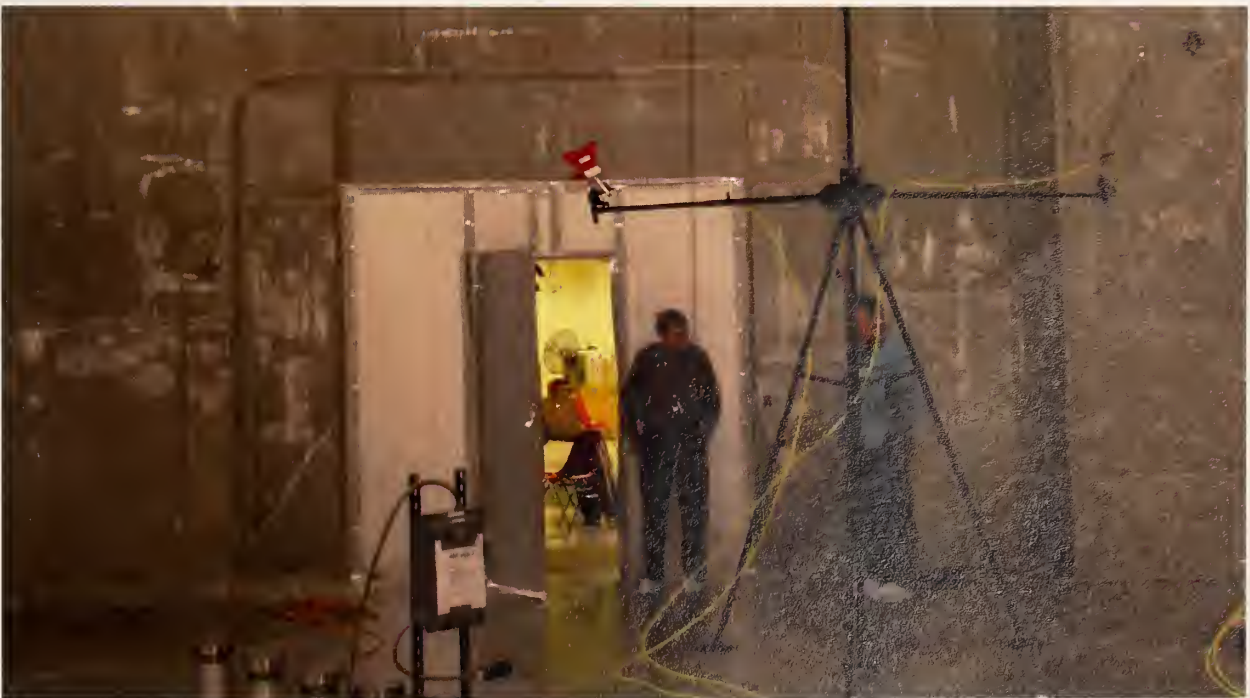
Figure 90. Personnel door made of foil-covered polystyrene foam.
