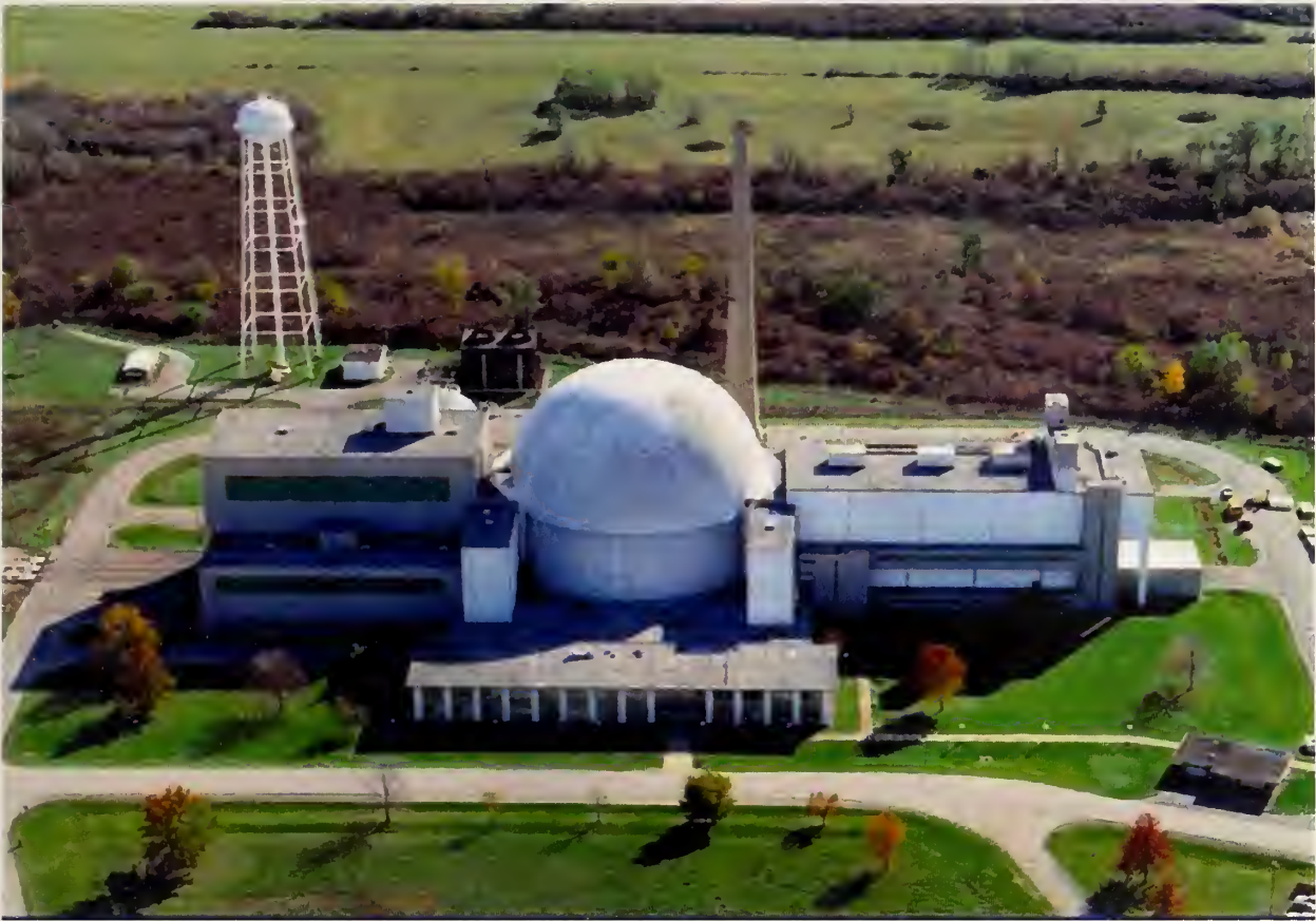
Figure 1. Aerial view of NASA Space Power Facility located at the Plum Brook Station near Sandusky, Ohio. (Photo courtesy of NASA)
