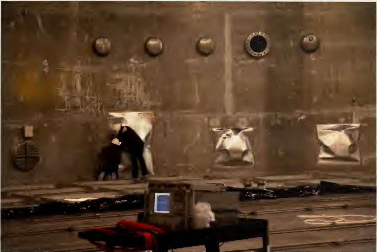
Figure 89. Covering probable leakage points.
