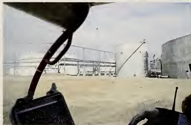
Figure 5.2-3: NIST staff collecting measurement data while driving around the perimeter of the facility among the large storage tanks.
