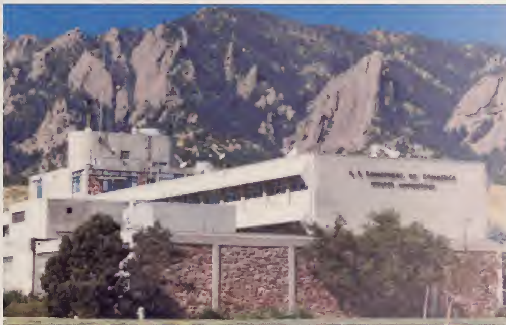
Figure 43. NIST main building (the Radio Building) in Boulder, CO.
