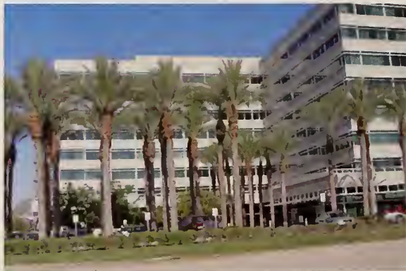
Figure 12. The office building in Phoenix, AZ.
