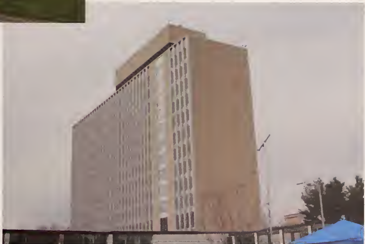
Figure 21. The NIST office building in Gaithersburg, MD.
