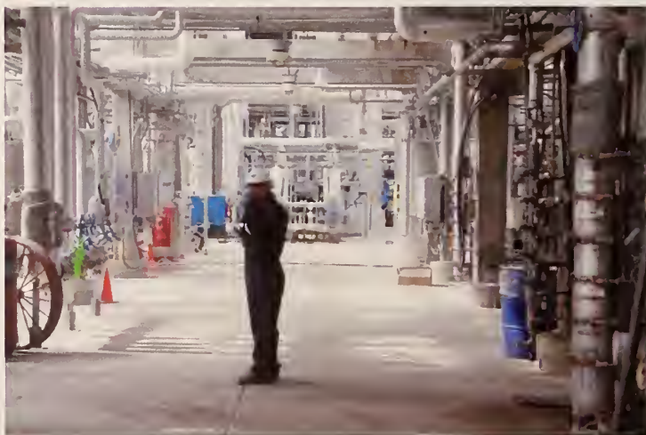
Figure 40. Inside the SUNCOR oil refinery in Commerce City, CO.
