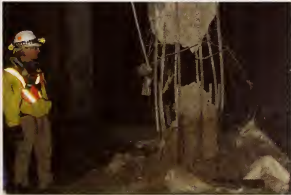
Figure 3. Pre-implosion preparation inside the convention center.
