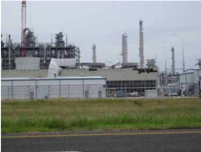
Figure 4-83 Cooling tower failures at the BASF Fina Plant in Port Arthur/Groves, Texas (photo credit: Christopher Letchford, Texas Tech University)
