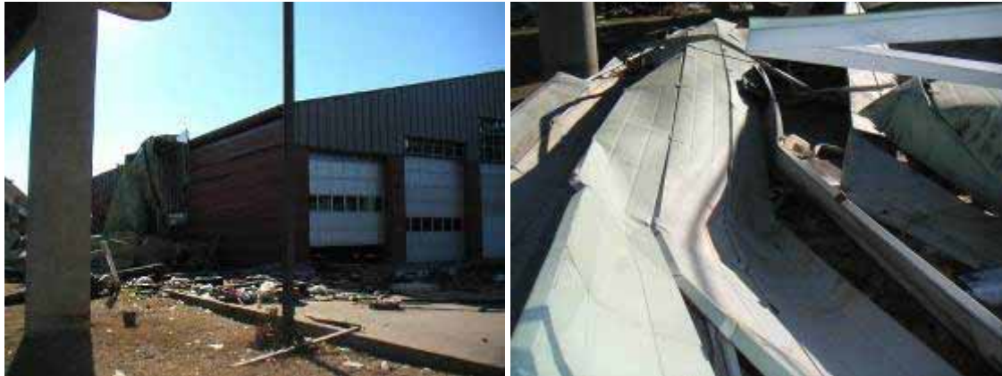
(a) (b) Figure 3-38 New Orleans Third District Fire Headquarters. (a): roof damage. (b): apparent lack of fasteners (Photo credit: Keith Porter, Scawthorn Porter Associates).
