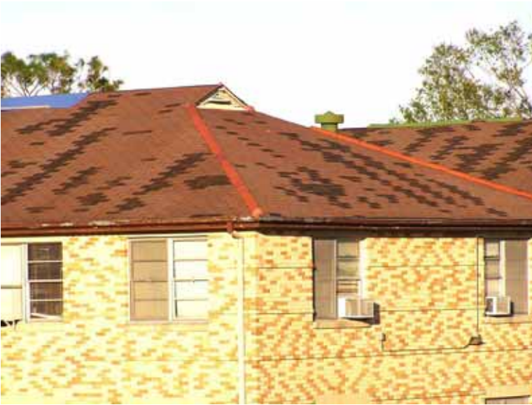
Figure 5-22 Damage to older three-tab asphalt shingles wherein approximately 40 percent to 50 percent of the shingles were blown off the front side of the home in New Orleans. Note the vertical strips of blown-off shingles. This failure pattern is associated with applying the shingles in a process known as “racking” in which shingle are applied vertically or straight up the roof. Racked–applied shingles are susceptible to blow-off as illustrated here, and the process should not be carried out in regions susceptible to high winds. (Photo credit: Robb Smith, Amtech Roofing Consultants)
