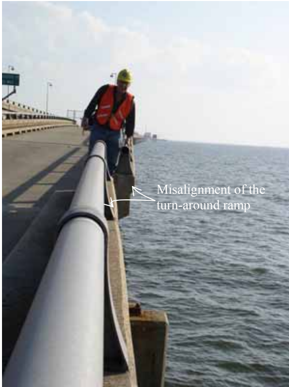
Figure 4-35 Misaligned spans of the Toll Causeway's turn around ramp (photo credit: Ron T. Eguchi, ImageCat).
