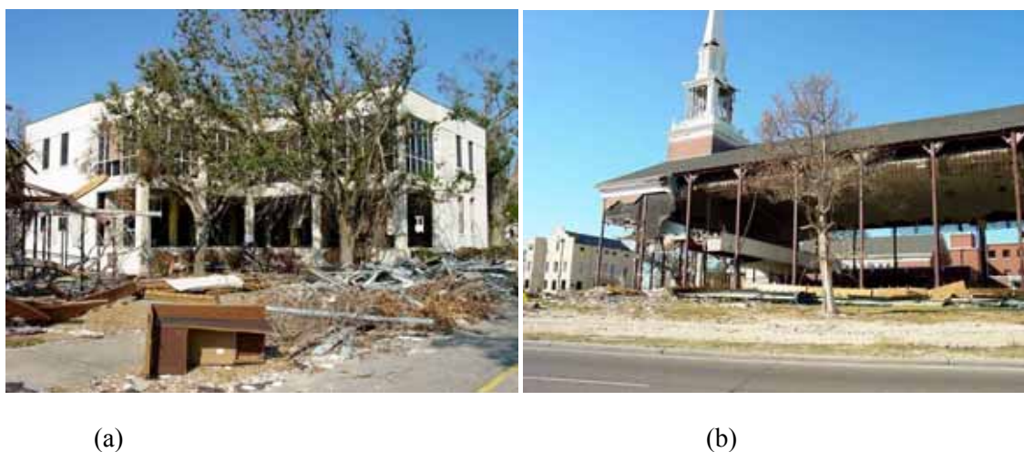
Figure 3-6 Damage due to storm surge at (a) the Department of Veterans Affairs hospital, and (b) First Baptist Church, in Gulfport, MS (Photo credit: (a) Habib Rahman, National Research Council of Canada, (b) Jack Hayes, USACE).
