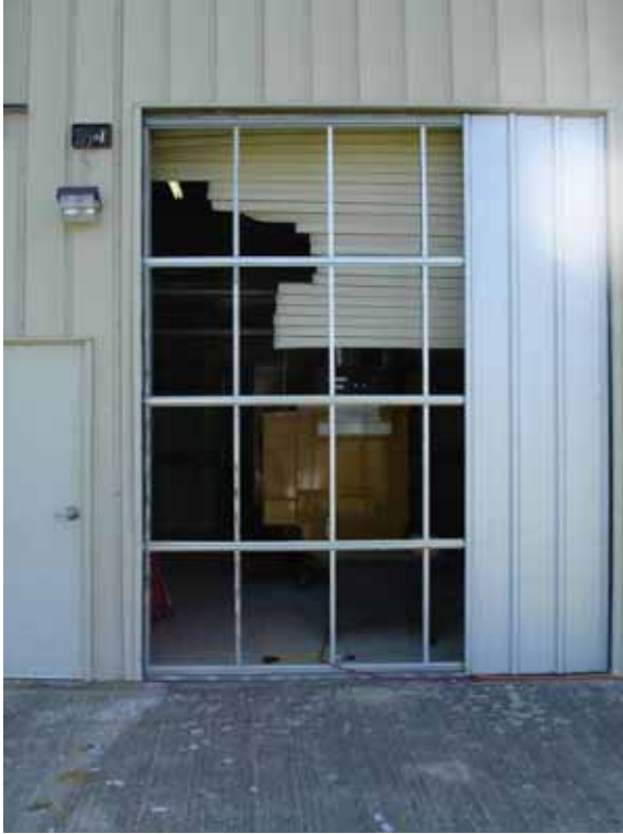
Figure 4-73 Roller door failure (with temporary framing and cladding) that led to auxiliary generator shutdown at Central Water Treatment Plant in Beaumont, Texas (photo credit: Christopher Letchford, Texas Tech University)
