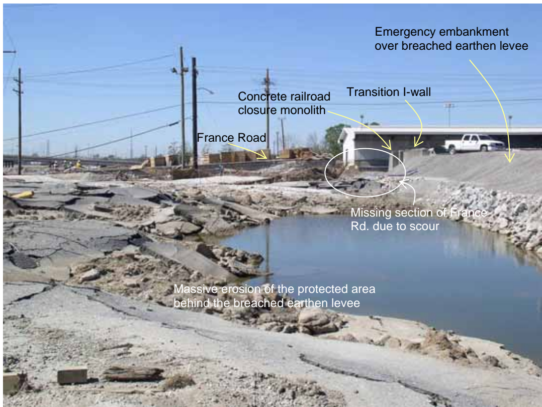
Figure 4-21 Erosion behind breached earthen levee. The breach occurred at the transition between the earthen levee and the transition I-wall (photo credit: NIST)
