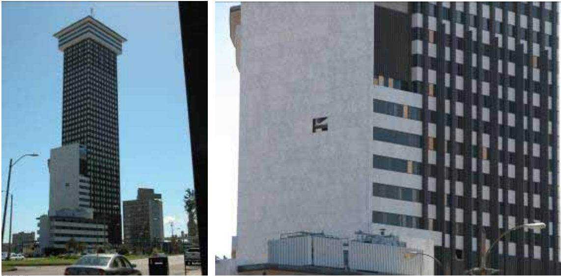
Figure 3-51 Unusual instance of damage to stone cladding due to wind pressure (Photo credit: Keith Porter, Scawthorn Porter Associates).
