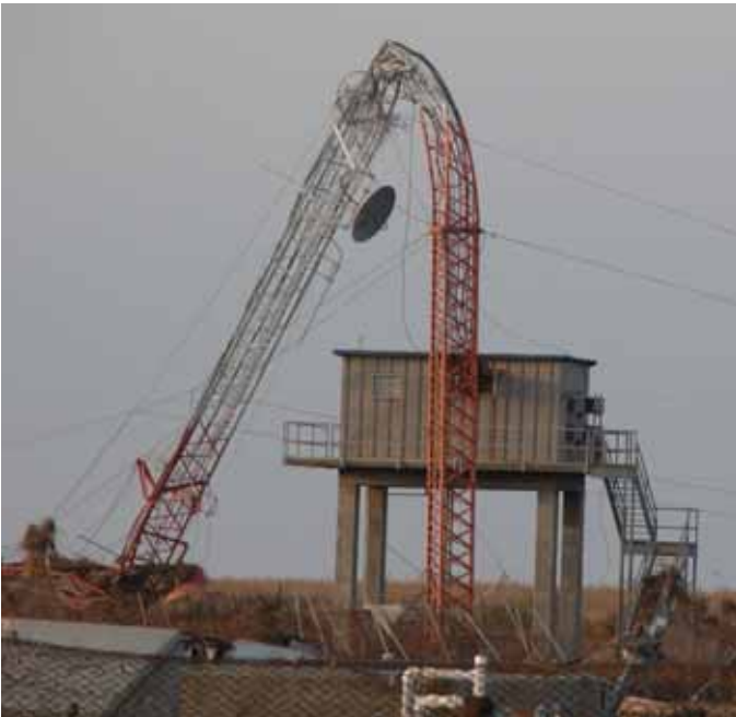
Figure 4-77 Downed communications tower on US Route 82 near Holly Beach Louisiana following Hurricane Rita (photo credit: Christopher Letchford, Texas Tech University)
