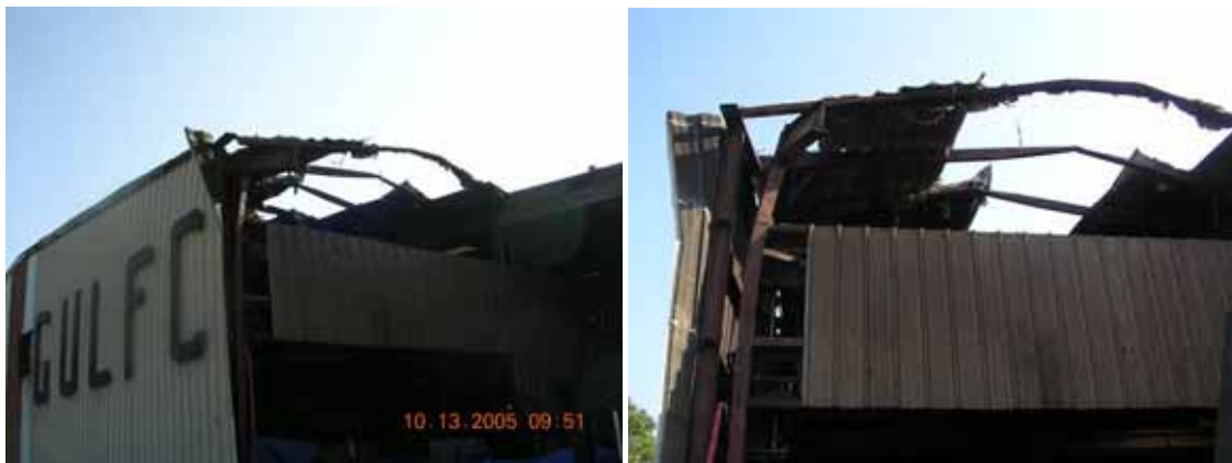
Figure 3-16 Buckled purlins and collapse of a portion of the end bay of a steel-frame warehouse from wind pressure in Beaumont, TX (Photo credit: NIST).
