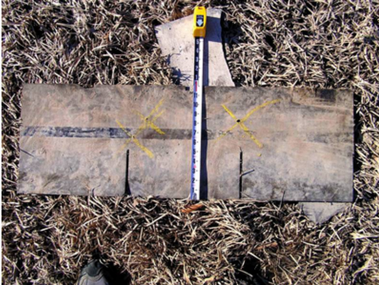
Figure 5-24 Example of a blown-off three-tab asphalt shingle that was clearly misapplied. The yellow Xs mark locations where the shingle was nailed in place. (Photo credit: Robb Smith, Amtech Roofing Consultants)
