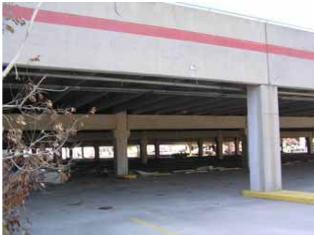
Figure 3-2 Successful performance of a single-story parking structure in Biloxi, MS (Photo credit: NIST).
