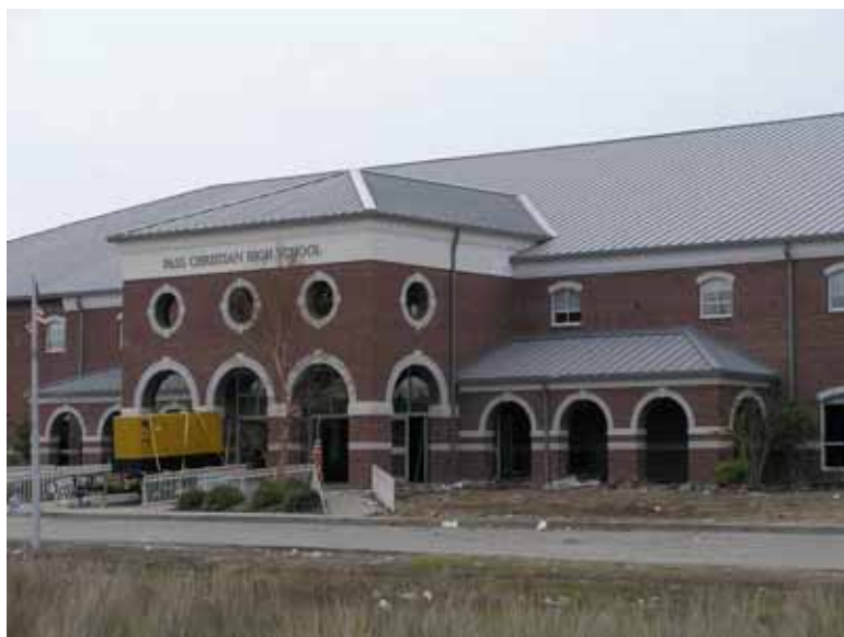
Figure 3-33 Standing seam metal roof in the coastal region of Pass Christian, MS, that sustained Hurricane Katrina without damage (Photo credit: NIST).
