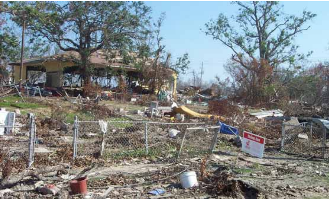
Figure 5-3 Residential damage in Biloxi, Mississippi. Masonry components survived. (Photo credit: Thomas B. Rodino, Shiner Moseley and Associates, Inc.)
