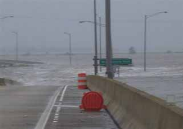
Figure 4-50 Surge waters overtopped US I-10 bridge ramp over Mobile Bay. View is eastbound, taken on the same day Hurricane Katrina hit (8/29/06). (Photo credit: George Conner, MSDOT)
