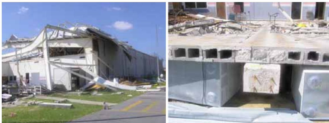
Figure 3-10 Damage to Gaston Hewes Recreation Center in Gulfport, Mississippi (Photo credit: NIST).
