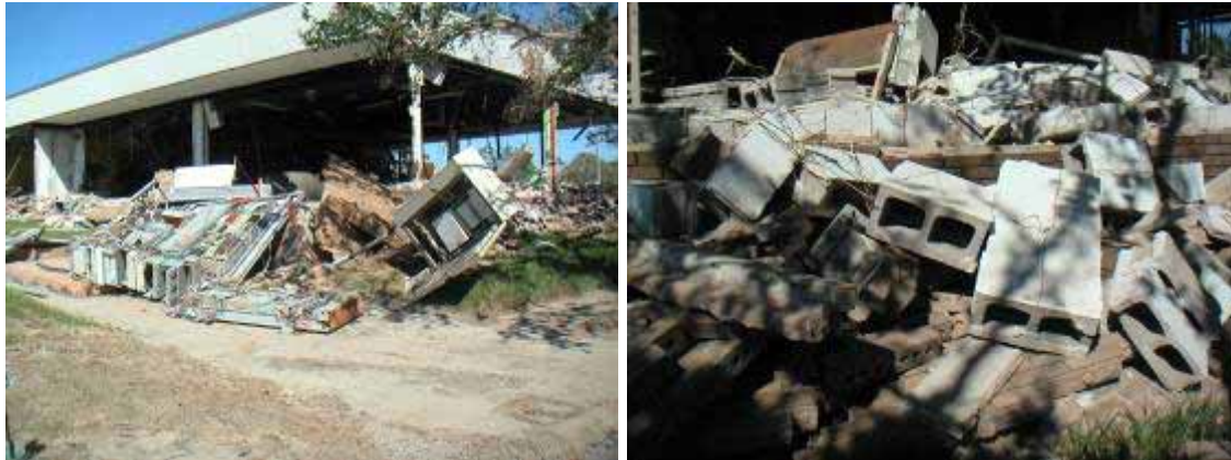
Figure 3-4 Storm-surge-induced collapse of CMU walls at the Venetian Isles Fire Station in New Orleans (Photo credit: Keith Porter, Scawthorn Porter Associates).
