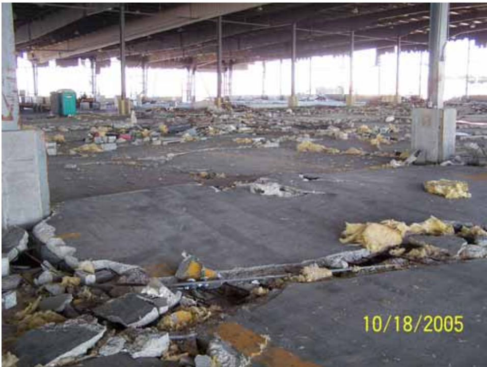
Figure 4-63 East Pier, showing damage to cargo shed deck and sheet metal siding (photo credit: Thomas B. Rodino, Shiner Moseley and Associates, Inc.)
