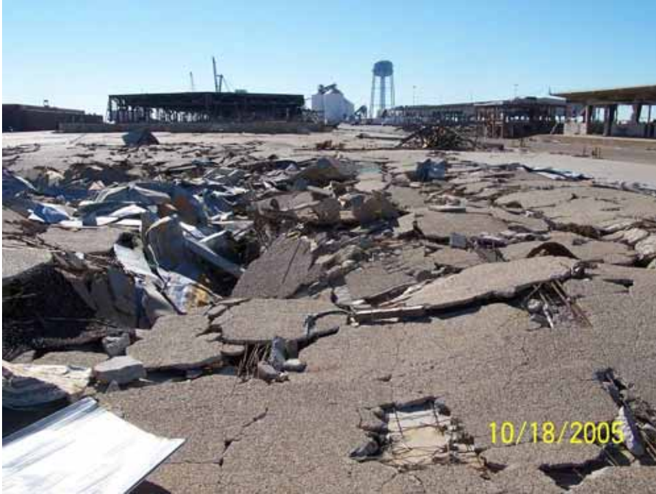
Figure 4-62 West Pier, showing collapse of wharf structure due to pile failure (photo credit: Thomas B. Rodino, Shiner Moseley and Associates, Inc.)
