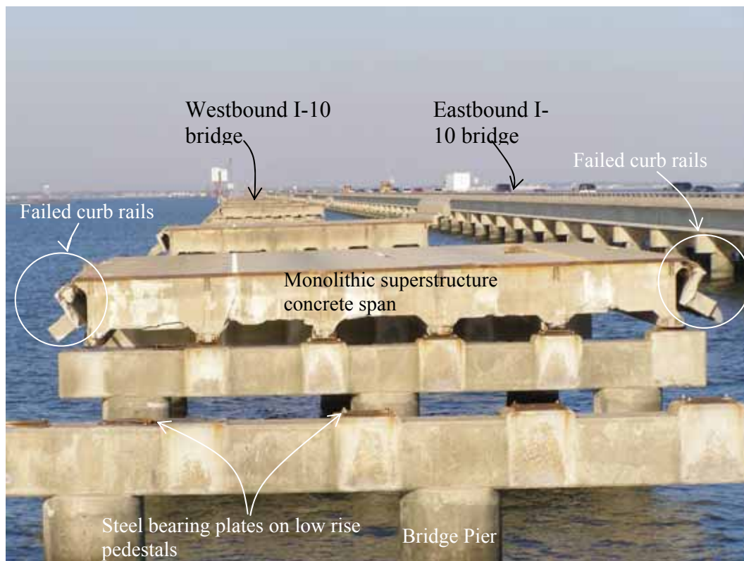
Figure 4-31 View looking north from west abutment of I-10 twin span bridges over Lake Pontchartrain (photo credit: NIST).
