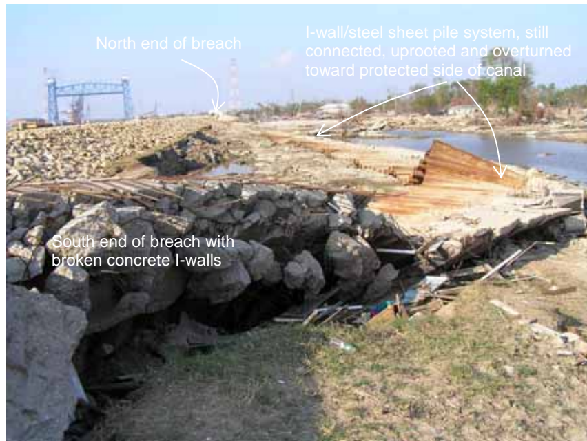
Figure 4-26 Overturned and uprooted floodwall at the IHNC Lower Ninth Ward South breach, with the I-walls remained connected to the sheet piles (photo credit: NIST)
