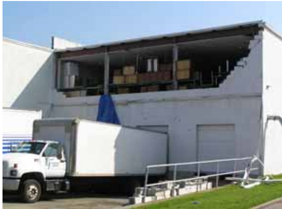
Figure 3-9 Failure of a non-load bearing masonry wall in Beaumont, TX (Photo credit: NIST).
