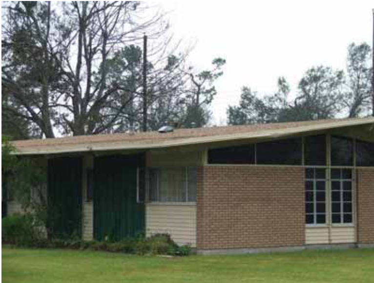
Figure 5-26 A small number of single-family, single-story homes having built-up bituminous membrane roofing (BUR) were seen. Those observed were undamaged as was the case for this house in Orange, Texas. (Photo credit: Dominic Sims, International Code Council)
