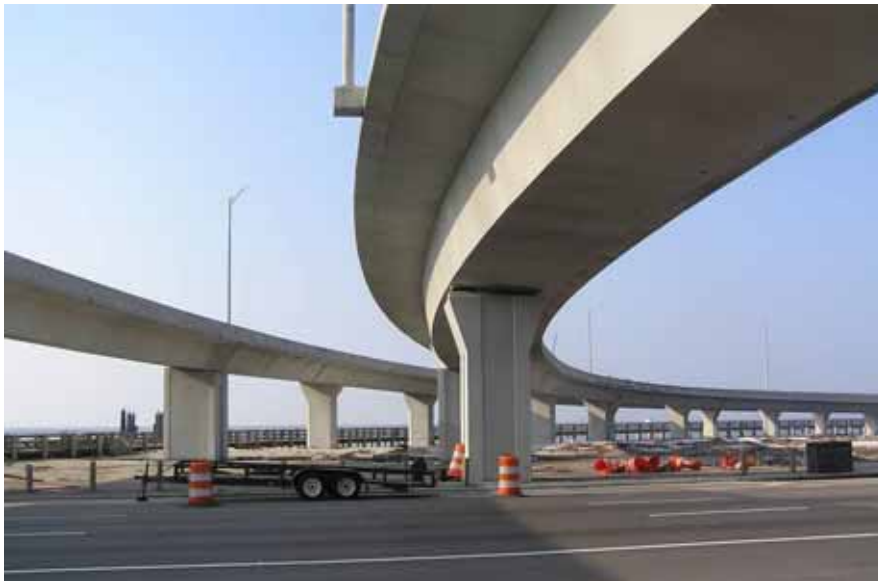
Figure 4-45 I-110 bridge ramps with cast-in-place, continuous box girder superstructure positively connected to bridge piers (photo credit: NIST)
