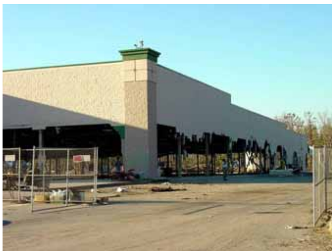
Figure 3-5 Storm-surge-induced collapse of the lower portions to a reinforced CMU wall in Gulfport, MS (Photo credit: Habib Rahman, National Research Council of Canada).
