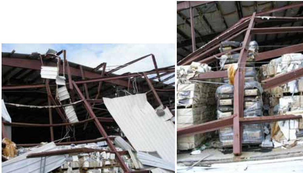
Figure 3-15 Collapse of the entire end bay of a steel-frame warehouse from wind pressure near Long Beach, MS (Photo credit: NIST).
