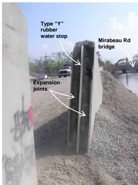
Figure 4-13 I-walls of failed floodwall section separated along water stop joint (photo credit: NIST)
