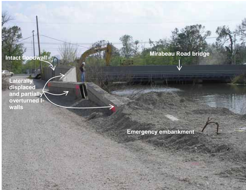
Figure 4-12 View looking south from the breach on the east bank of the London Avenue Outfall Canal toward Mirabeau Road bridge (photo credit: NIST)
