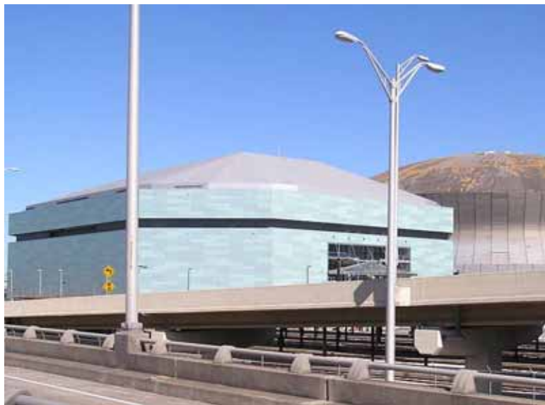
Figure 3-25 The New Orleans Arena, which has an SBS modified bitumen membrane, withstood the Hurricane Katrina winds without damage. (Photo credit: Robb Smith, Amtech Roofing Consultants).
