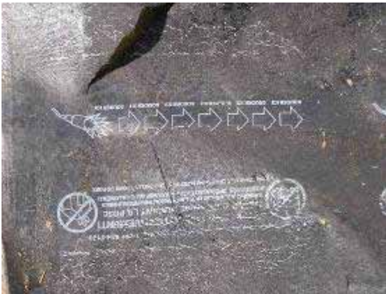
Figure 3-24 Had this failed heat bonded polymer-modified bitumen membrane been heated in accordance with acceptable practice, the plastic film and white markings would not be present (Photo credit: Robb Smith, Amtech Roofing Consultants).
