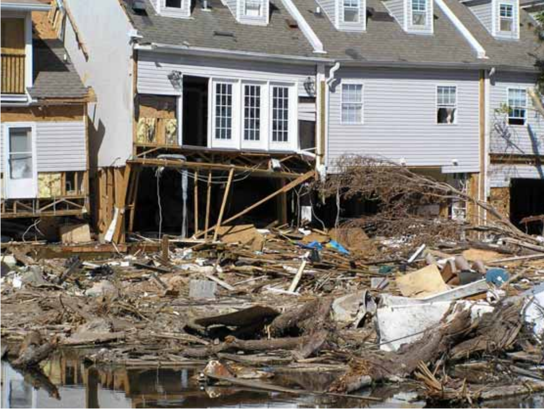
Figure 5-4 Severe damage and destruction to townhomes in Gulfport, Mississippi. (Photo credit: NIST)
