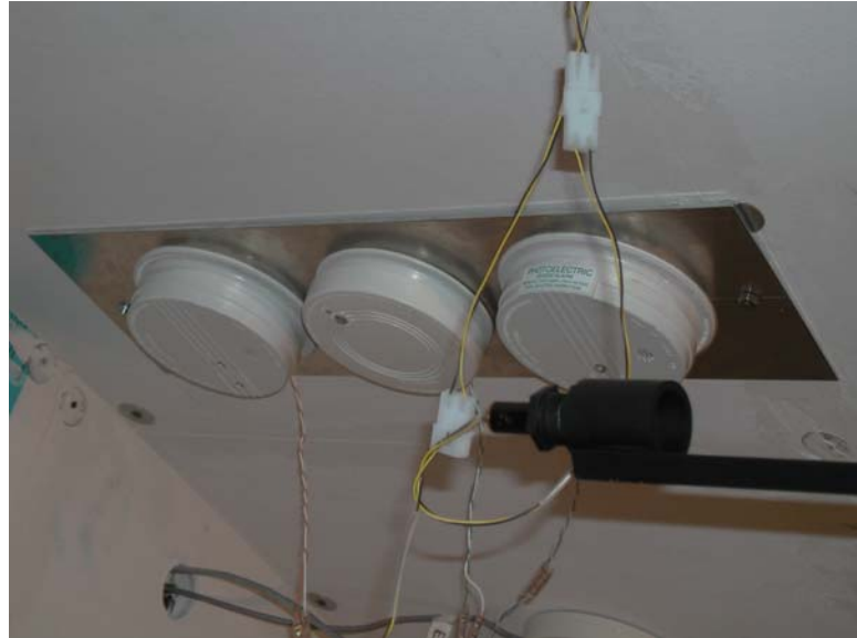
Figure 99. Measurement station showing unmodified smoke alarms arranged for testing
