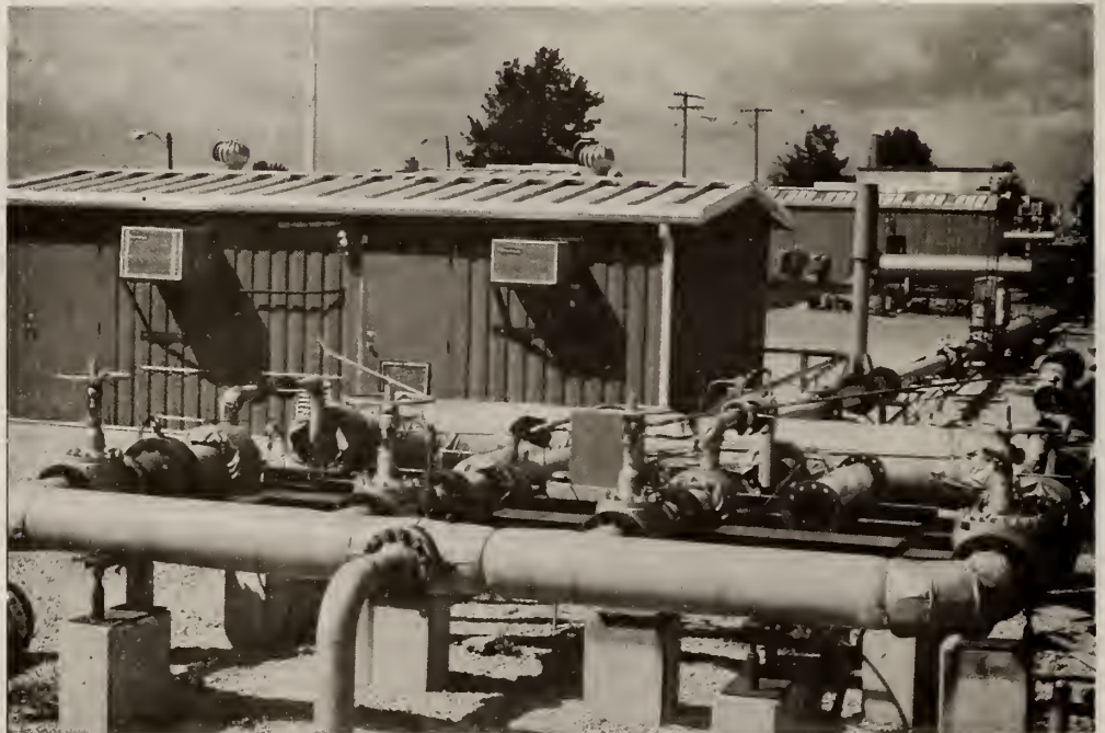
Photo No. 10 (1984 Piping Configuration)
