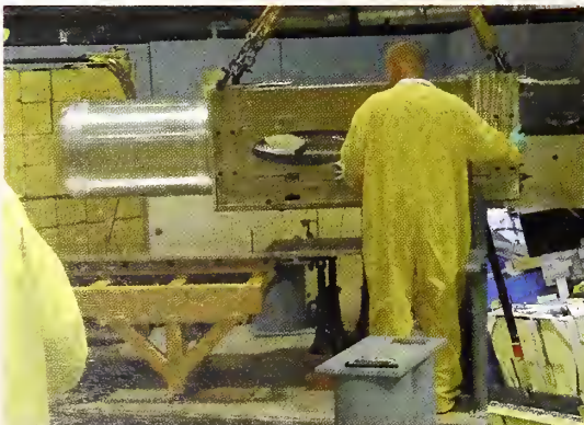
Unit 2, the new cold source assembly, is moved into place (above) and rides a track (right) into the cold source thimble.
