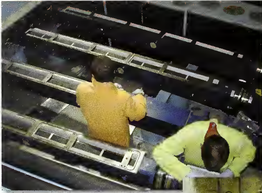
Biological shielding is removed and guides are disassembled prior to removing the Unit 1 cold source.
