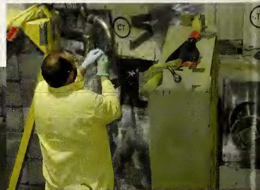
Connections to hydrogen condenser are welded into place.
