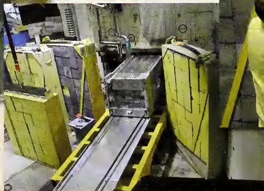
Unit 2, the new cold source assembly, is moved into place (above) and rides a track (right) into the cold source thimble.
