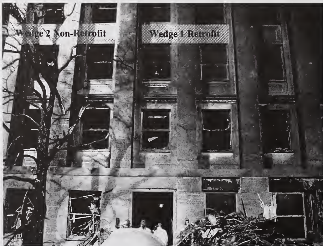
Figure 4. Exterior view of transition between Wedge 1 (on right, retrofit) and Wedge 2 (on left, non-retrofit). First floor non-retrofit window adjacent to transition may be High Hazard blast response. Second and 3 rd floor fire damage. Approximately 135 ft (44.2 m) North of plane impact point.
