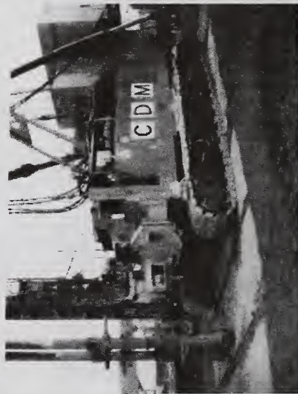
Photograph Improved ground by CDM (UCB & CDM Association)
