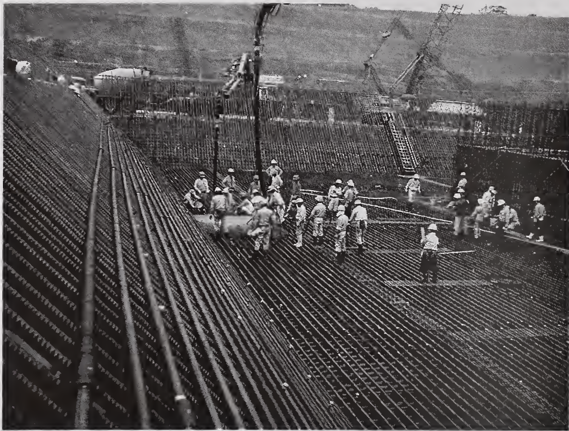
Fig. 4 First Concrete Casting for Shaking Table Foundation (June 20, 2000)
