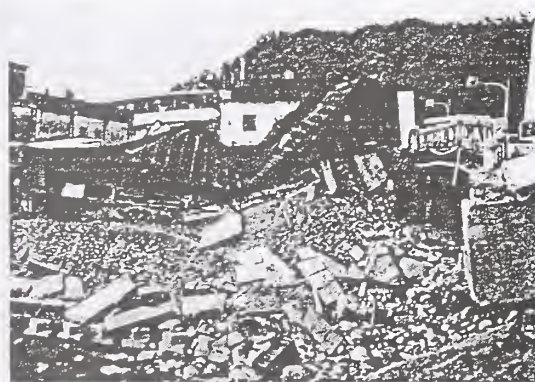
Photo 4 Building collapsed just above fault (Fengyuan City, Taichung County) Building of brick is perfectly destroyed
