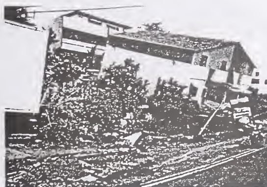
Photo 5 Building just above fault (Fengyuan City, Taichung County) The ground behind building is rised. The building in this vicinity got same damage
