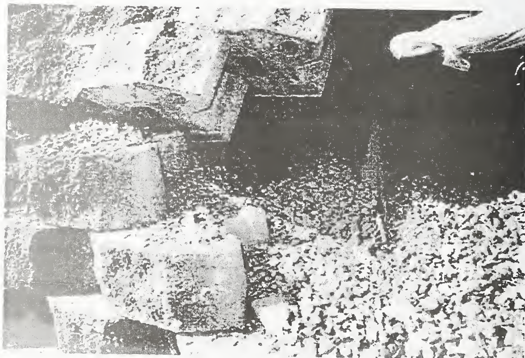
Photo.6 Close view of the collapsed segmental wall
