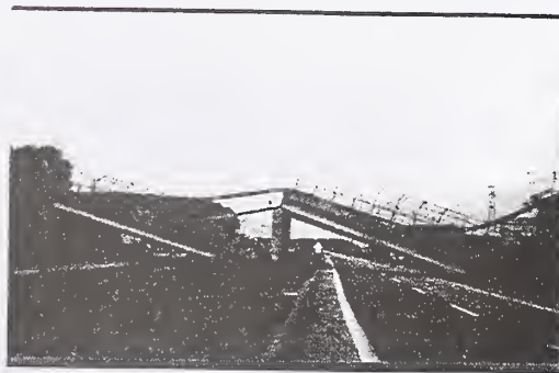
Photo 6 Collapse of Arifiye Bridge (Courtesy of H. Hoashi)
