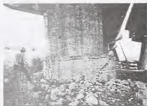
Photo 14 Failure of Caisson Foundation as a Direct Fault Movement, Wu-Shi Bridge (Courtesy of S. Iwata)
