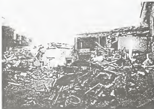
Photo 21 Damage of sundried brick structure (Tungshih, Taichung County)
