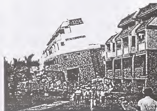
Photo 6 Building just above fault (Shihkang, Taichung County) RC multiple dwelling house of the new construction inclined by the fault. The pile is not used. The damage of the superstructure is very greatly nonexistent
