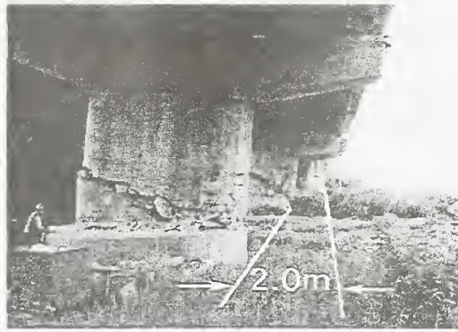
Photo 15 Lateral Movement of P1 and P2, Wu-Shi Bridge
