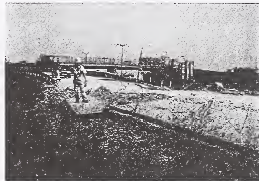
Photo 7 Minor Damage in an Overpass where the Fault Crossed the Overpass at Its Abutment
