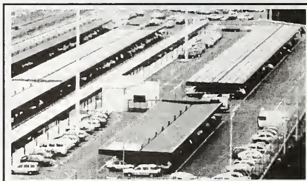
Fig. 41. PV Parking Structure near Rome
