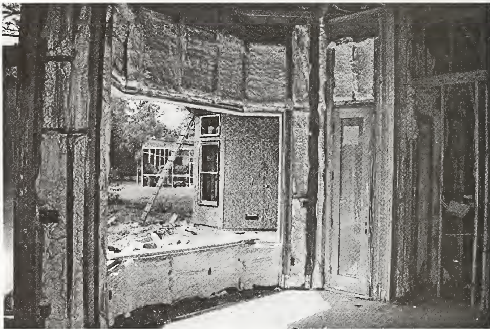
Foam is easy to apply in hard to insulate areas (Wall corners, window headers, etc.)
