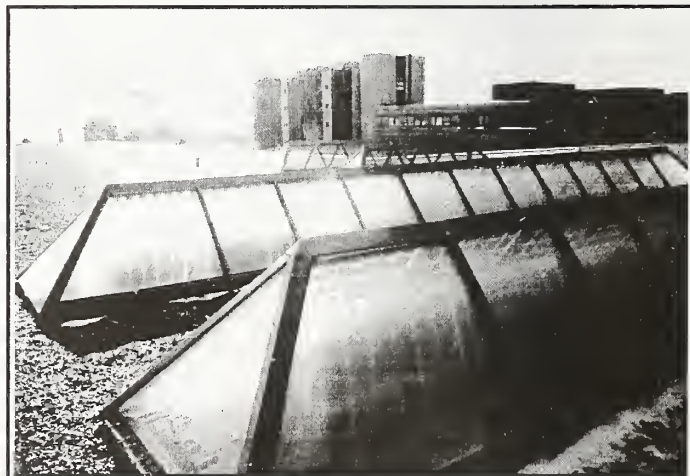
Fig. 15. Integral PV / Daylighting monitors at EPFL
