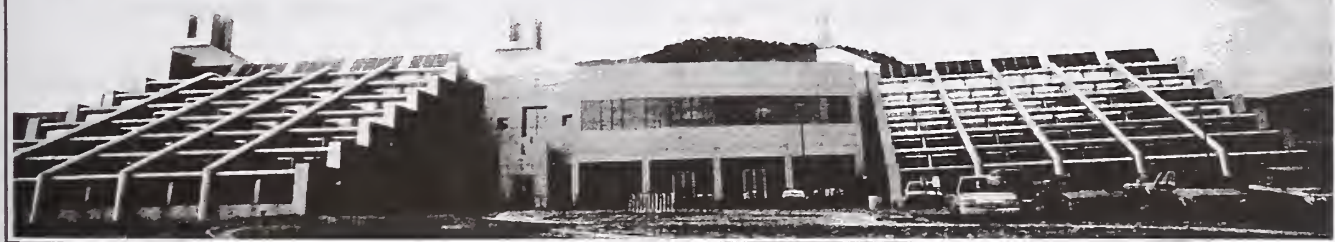
Fig. 34. The US National Renewable Energy Laboratory's new SERF building features a 15 kWp PV system
