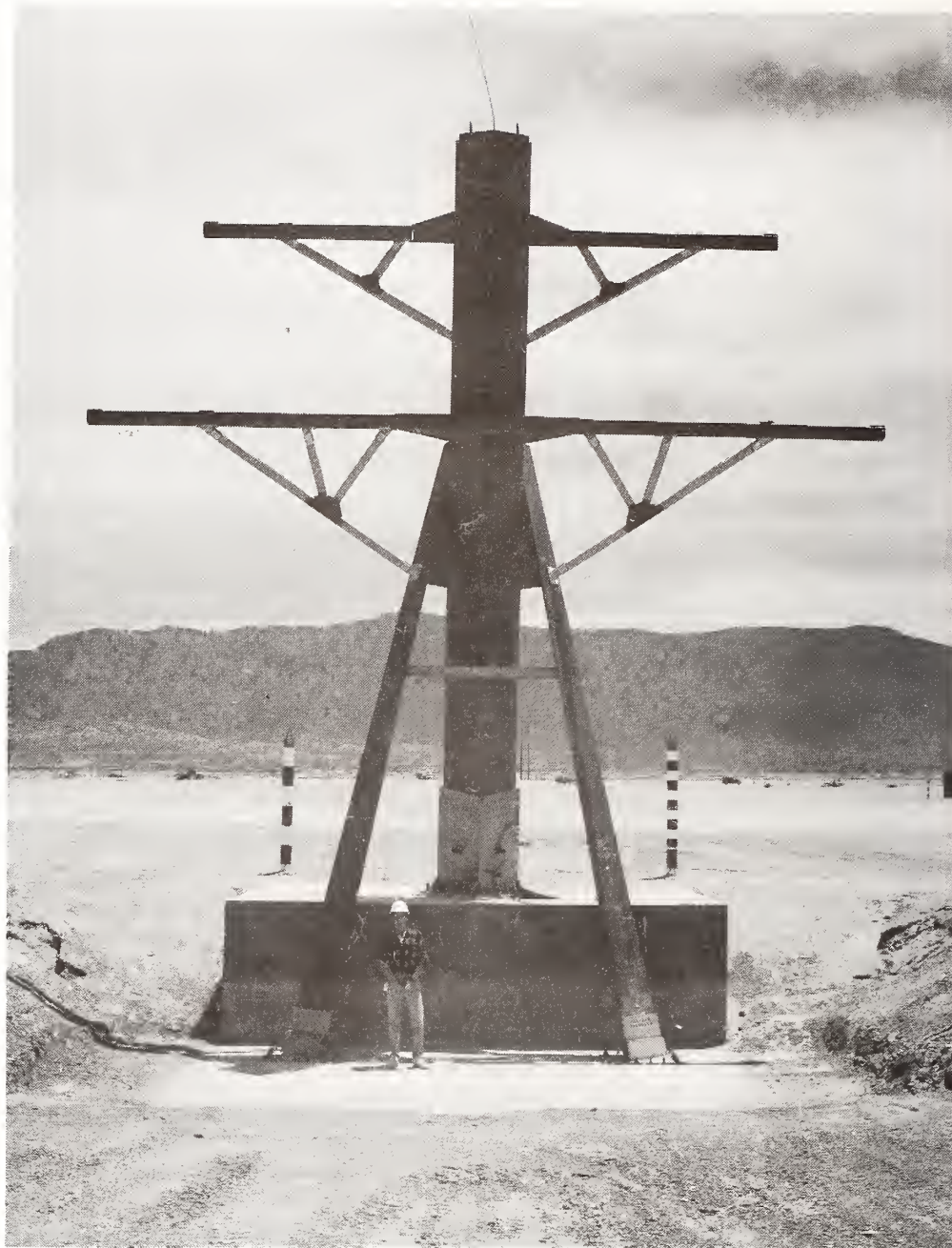
Figure 11. 1/2 - Scale Composite Ship Mast
