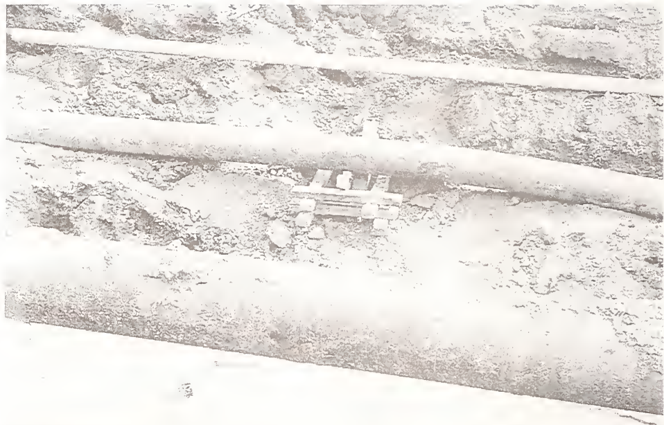
Figure 50 Some of the buried pipelines located near the intersection of Balboa Boulevard and Bircher Street--the potential hazard of co-location of lifeline systems. At this site are three water lines (two of them main lines); three gas lines; two sewers; one crude oil line; overhead power, telephone, and cable TV lines; the street lighting system; and the street itself.
