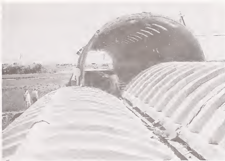
Photo 4.4 Collapse of A Snow Shelter (Okushiri Island)
