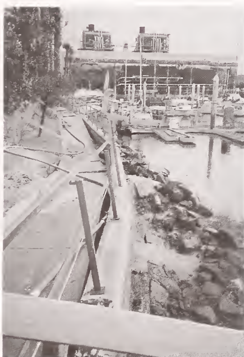
Photo 6.2 Displaced Bulkhead
