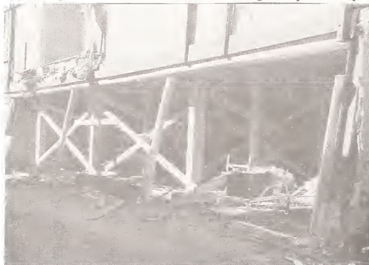
Photo 5.2 Damage of Northridge Meadows Apartment (First floor of the right side building was reinforced using wooden columns. Original posts were slender steel pipes)
