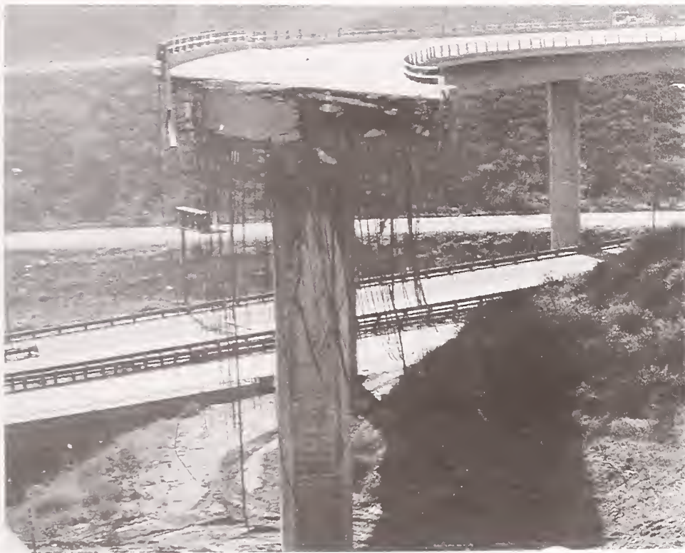
Figure 31 View of the flexural failure at Pier 3 of the SR14/I5 North Connector Overcrossing, looking to the south
