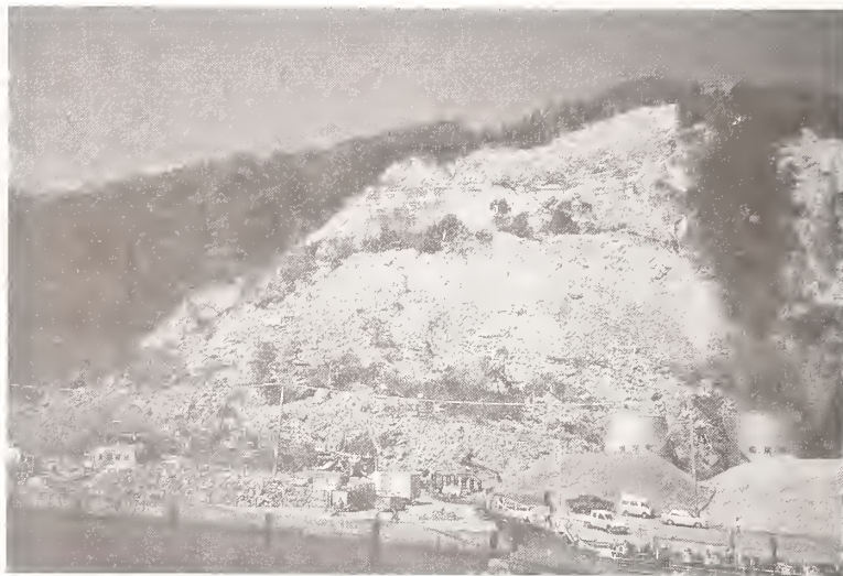
Photo 10.1 Slope Failure at Okushiri District
