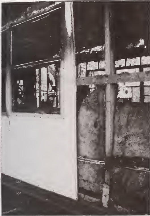
Photo 8.5 Structure of External Wall of a Mobile Home (Frame is of wood and siding is of hard board or aluminum panel)
