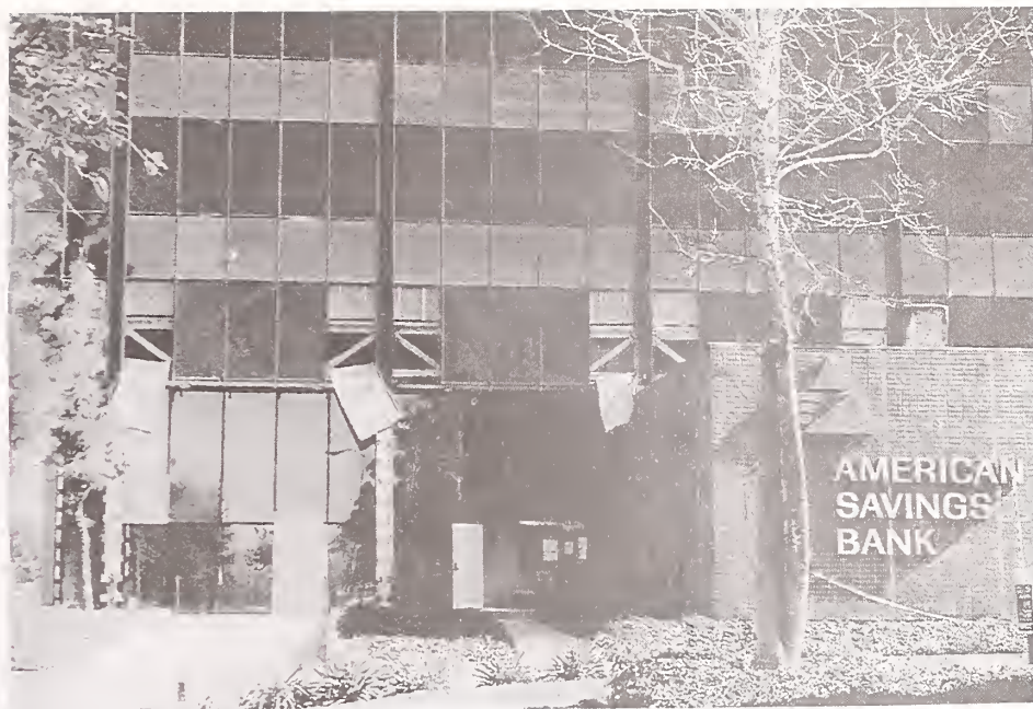
Figure 17 The first-story columns of the steel-framed building housing the American Savings Bank on Topanga Canyon Road in Canoga Park flexed during the quake and ended up slightly displaced from their original positions.
