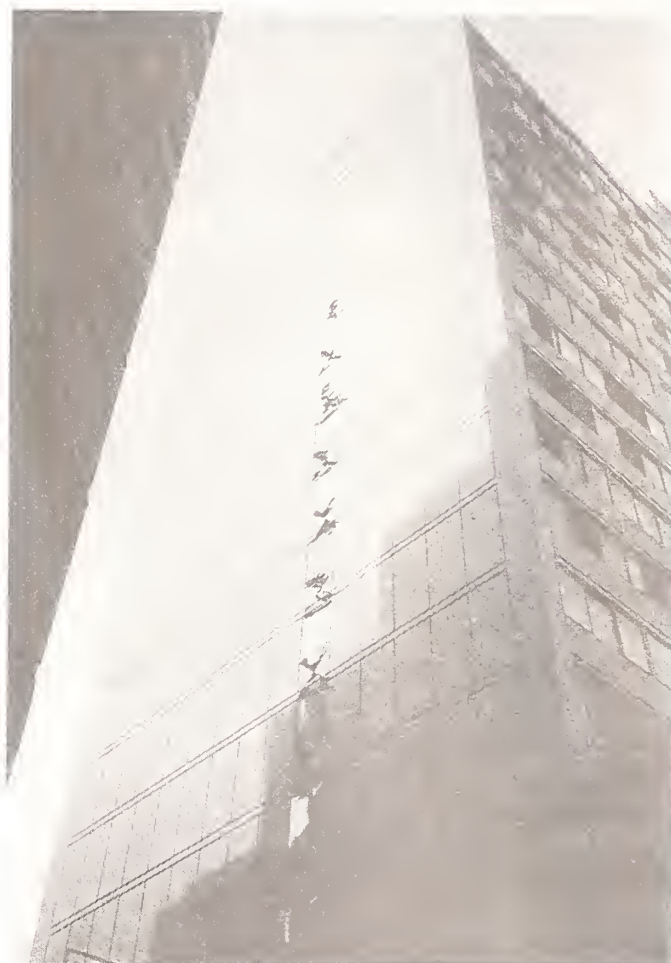
Figure 8 Champagne Towers apartment building in Santa Monica suffered a classic form of earthquake damage: shear failure of the coupling beams between linked shear walls at the transverse end of the building.
