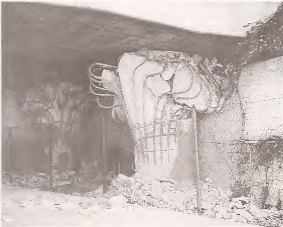
Figure 40 Piers of Bent 3 supporting eastbound lane of I10 at La Cienega Blvd.
