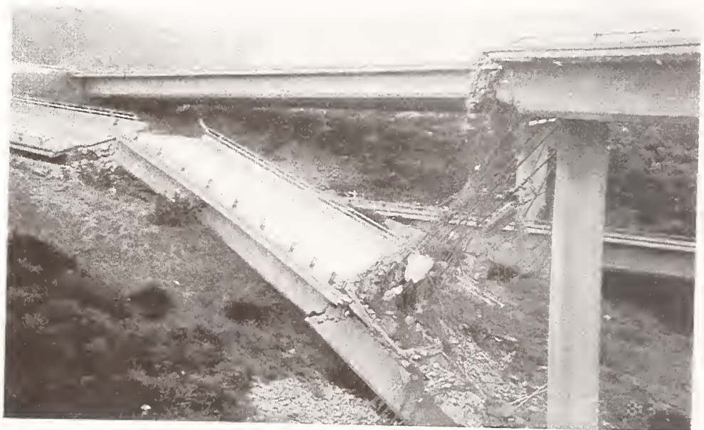
Figure 30 Collapsed portion of the SR14/I5 North Connector Overcrossing, looking east.. Pier 2 was at the left, near the broken hinge on the ground (Courtesy of EERC)
