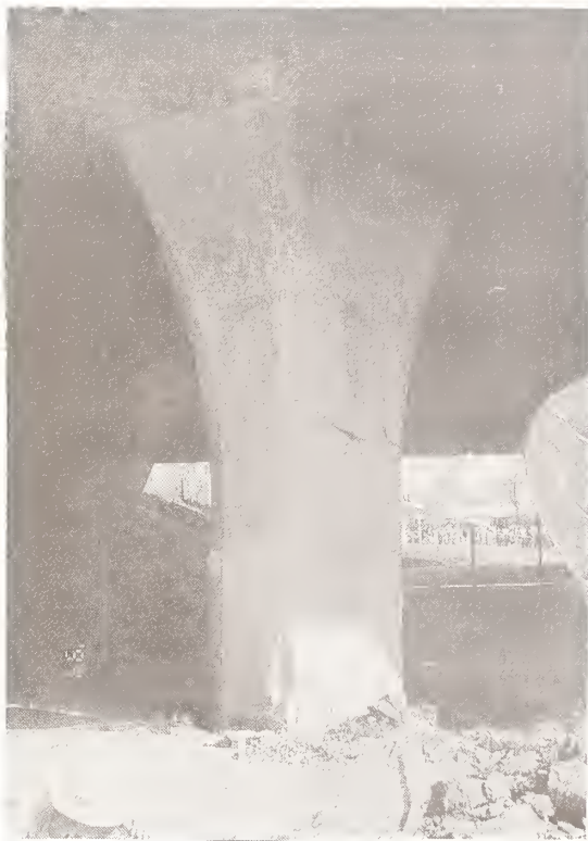
Photo 4.2 Initiation of Flexural Cracks (S-118 Mission/Gothic Undercrossing)
