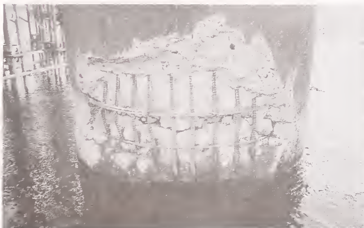
Photo 5.2 Damage of Pier P3 at Shin-shiriuchi Bridge
