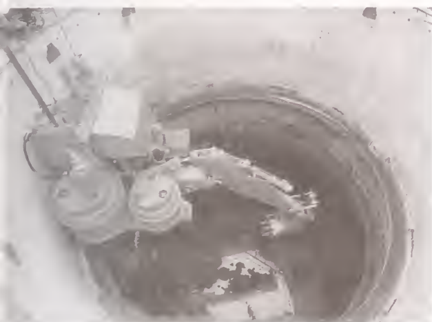
Plate - 3. The automatic excavators on the guide-rails
