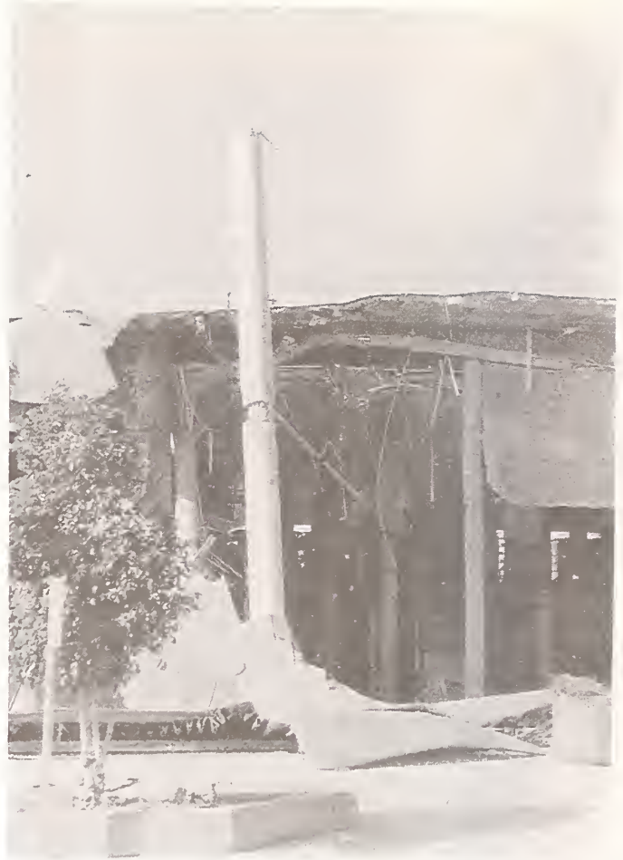
Figure 11 A portion of the concrete waffle slab roof and the interior floor slabs at the Bullock's department store at the Northridge Fashion Center mall fell to the basement, leaving many of the columns standing. No reinforcing steel can be seen in the remaining columns that would have connected the columns to the floor slabs.
