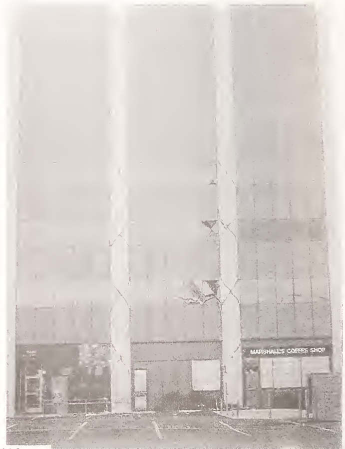
Figure 16 The stiff infill panels of the Barrington Building effectively shortened the concrete columns, forcing all the displacement into the column sections bounded by windows. Diagonal X-cracking decreased in severity towards the top of the building.
