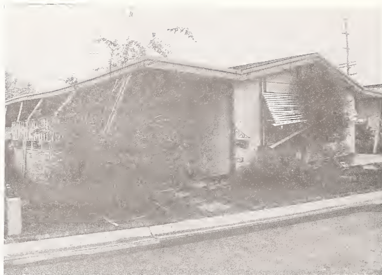
Photo 8.2 Damage of Mobile Homes due to Weak Supports
