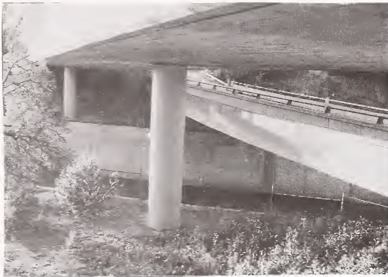
Photo 4.16 Effectiveness of Strengthening of Columns with Steel Jacketing
