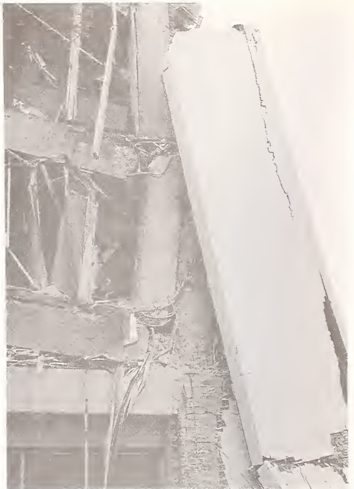
Figure 15 The exposed concrete frame of the Kaiser Permanente building, revealing deep beams, suggests that the building had a strong-beam, weak-column configuration. Except for the second story columns, the columns and beams remained intact while the joints disintegrated.
