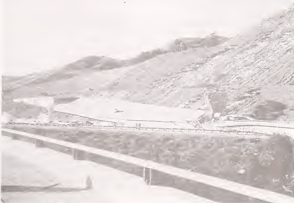
Figure 28 Overview of the collapse of the SR14/I5 Separation and Overhead, Ramp C, looking to the south at Abutment 1. Pier 3 can be seen at the right of the photograph (Courtesy of EERC)
