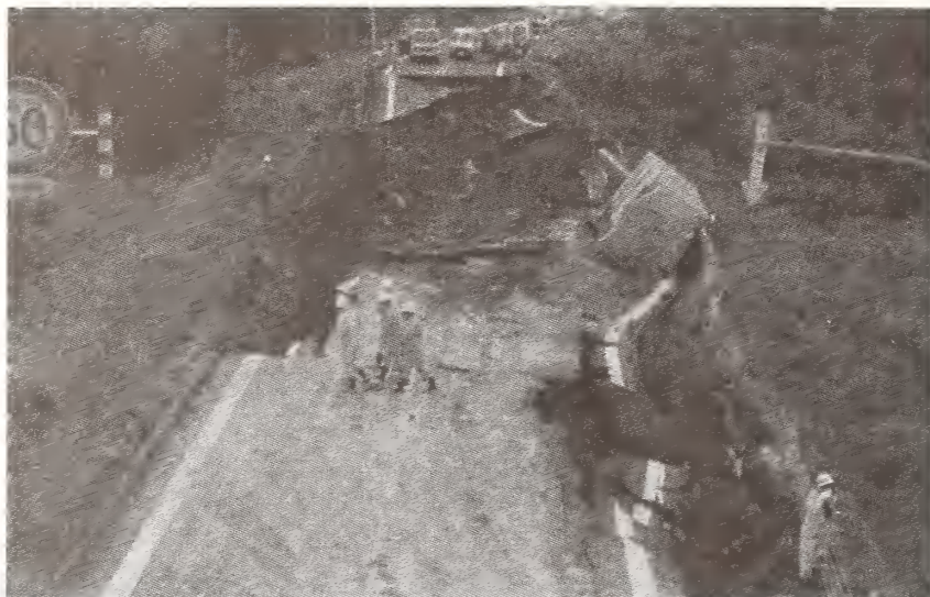
Photo 4.1 Collapse of An Embankment (National Road 5)
