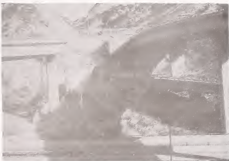
Photo 4.12 Collapse of North Connector Overcrossing (Courtesy of Patrick K. Hipley, Caltrans)
