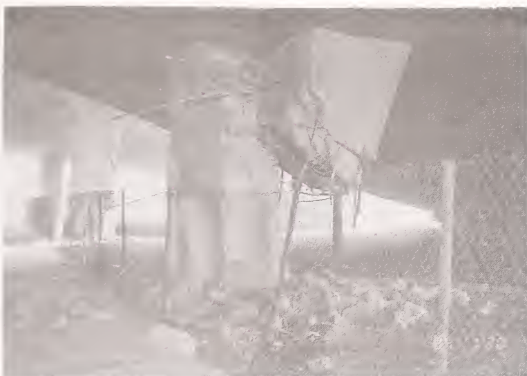
Photo 4.6 Complete Failure (S-118 Mission/Gothic Undercrossing)
