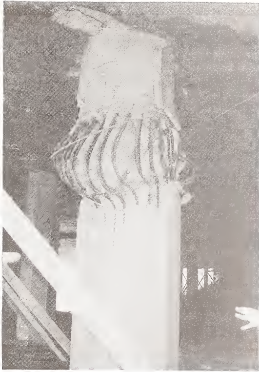
Photo 4.7 Damage of Columns of Bull Creek Channel Bridge
