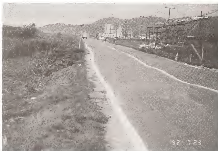
Photo 4.2 Permanent Undulating Deformation of Road Surface (National Road 5)
