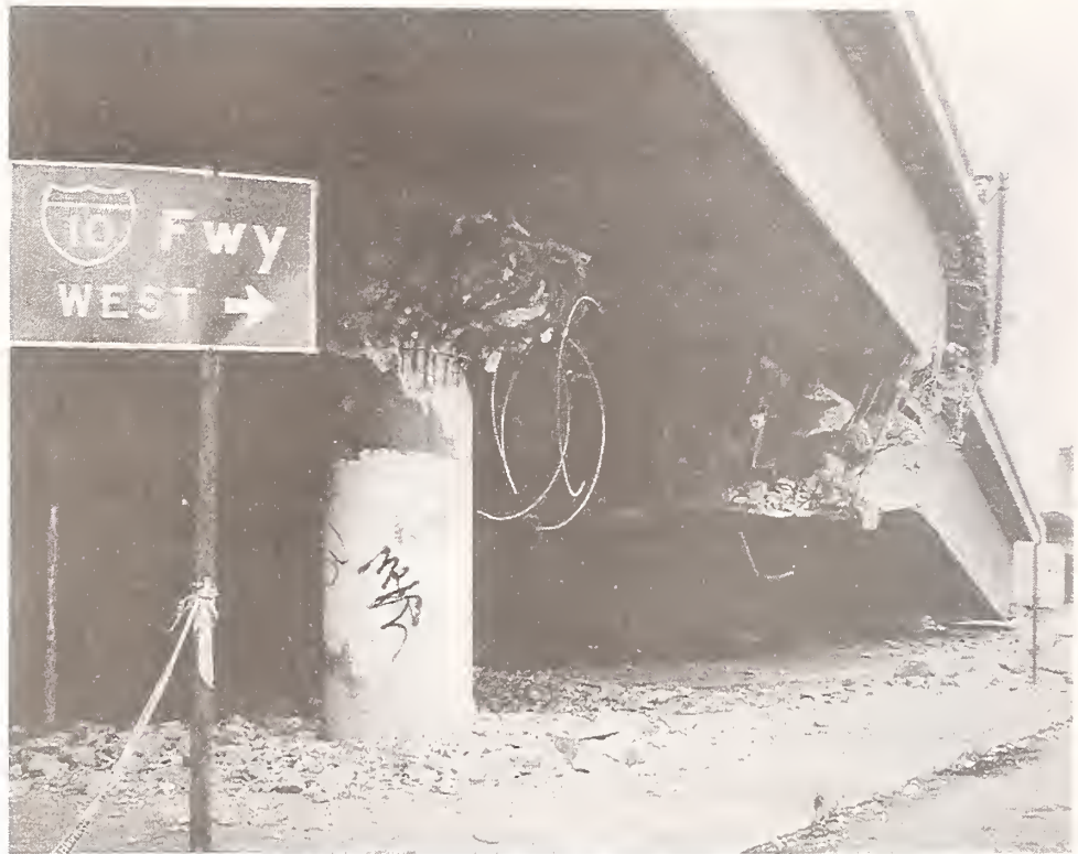
Figure 37 Collapsed westbound lane of I10 at Venice Blvd.; pier of Bent 7 in foreground
