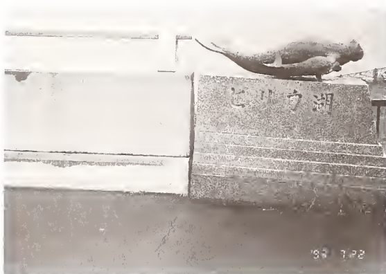
Photo.4 Settlement of Asphalt Paving and Gap of the Railing at the Crest around the Connection with Block 0 at Pirika Dam
