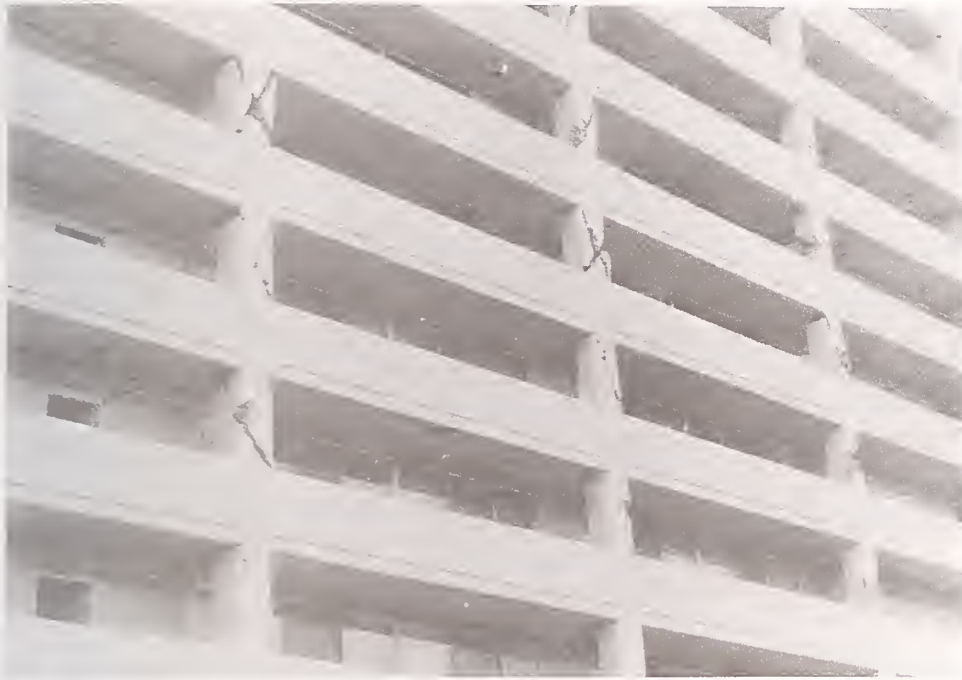
Figure 9 The back of the Champagne Towers building was badly damaged. The railings here are solid infill, which effectively stiffen the lower half of the columns. The shortened upper half of the columns were forced to accommodate all the displacement, and they failed in shear.
