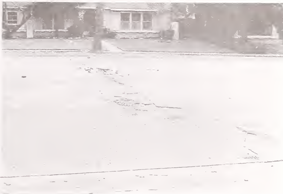
Figure 55 Transverse cracks in pavement along Balboa Boulevard in Northridge area.
