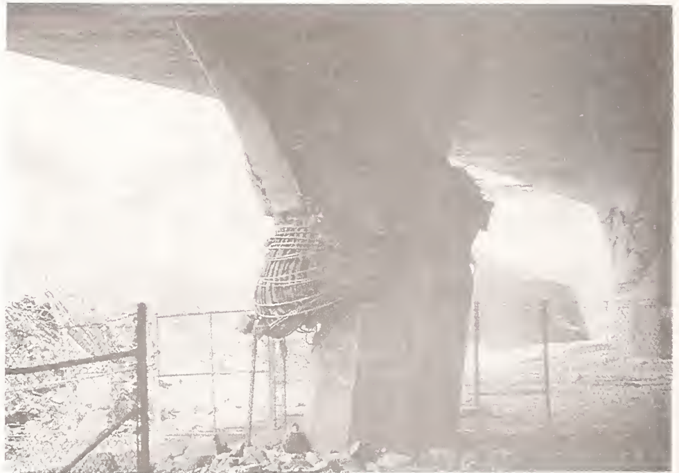
Figure 34 Damage to a pier of the SR118 Mission-Gothic Undercrossing, looking to the northwest at the southernmost pier of Bent 3 of the westbound bridge.
