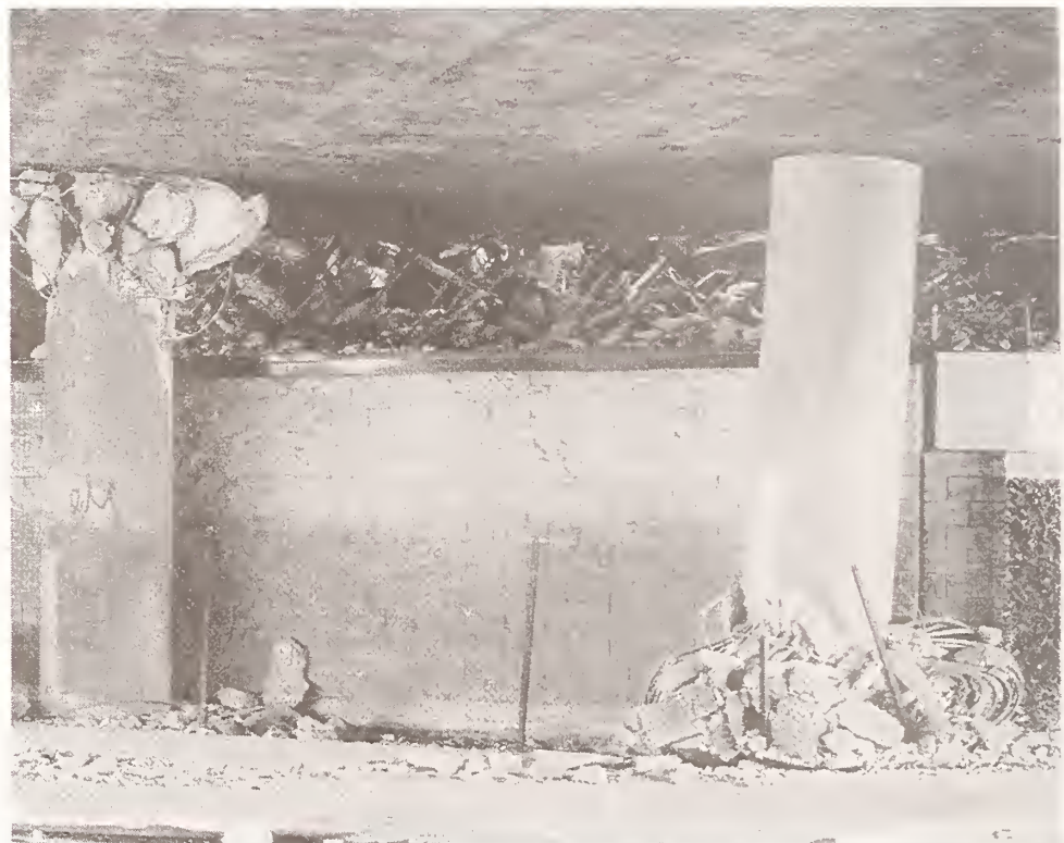
Figure 38 Failed piers in Bent 7 supporting westbound lane of I10 at Venice Blvd.
