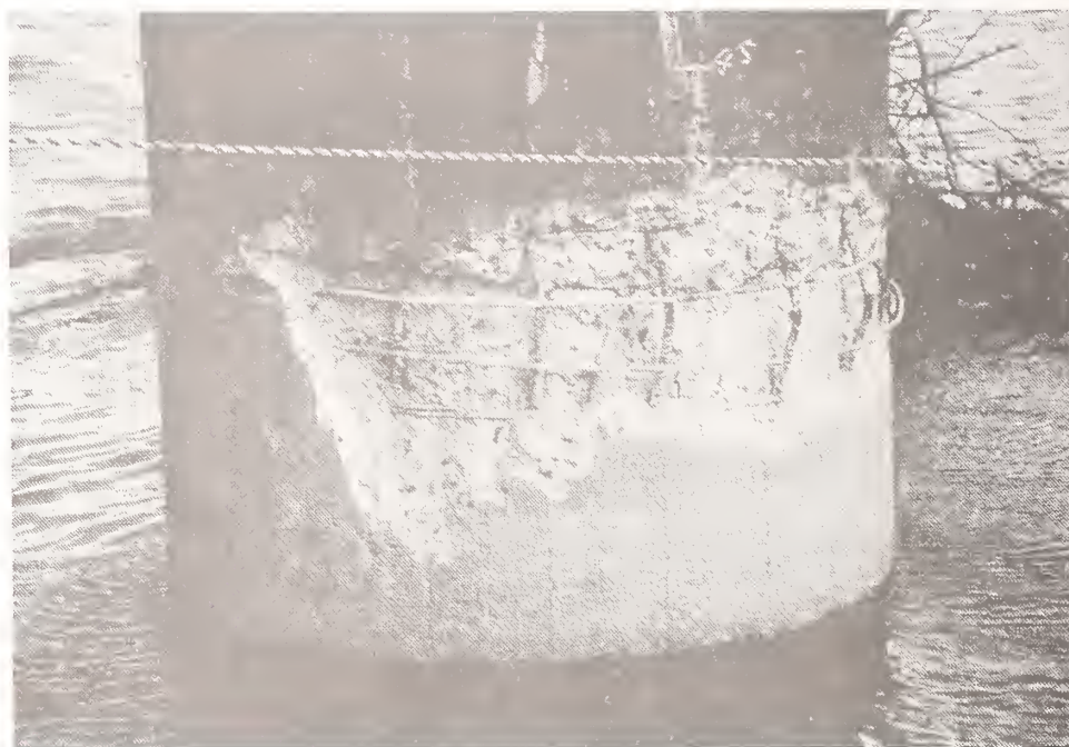
Figure 16C Detail of a damaged column of the bridge over the Assabu River. Note the buckling of the vertical reinforcing steel and the wide spacing of shear (horizontal) reinforcement. The estimated damage is 25 to 50% of the value of the bridge.
