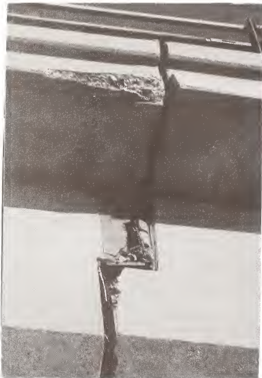
Photo 4.14 Large Separation and Damage of Hinge Seat (Courtesy of Patrick K. Hipley, Caltrans)
