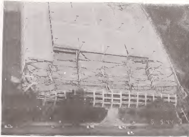
Photo 5.4 Damage of Parking Garage at California State University at Northridge
