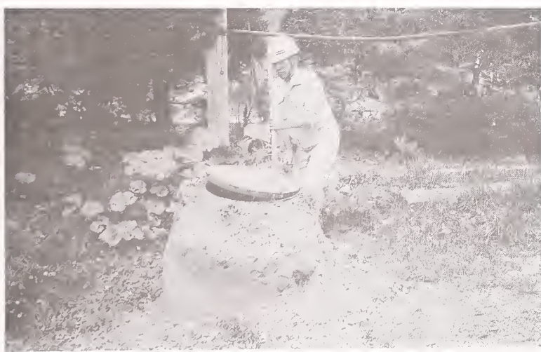
Photo 8.2 Uplift of Manholes
