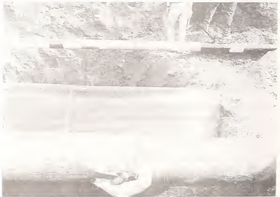
Figure 47 Ground contraction along Balboa Boulevard caused the rupture of a gas distribution line, the Rinaldi trunk water main, and a gas main.
