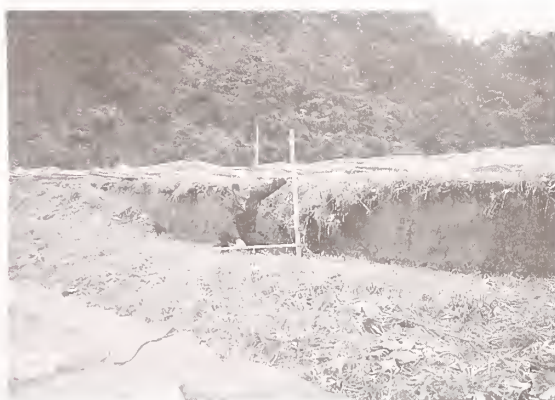
Photo.8 Level Difference on the Crest Caused by the Settlement of the Upstream Side of the Niwa-Ikumine Dam (Photographed on July 15, By the Courtesy of the Kita-Hiyama Land Improvement District)
