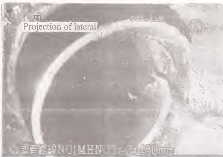
Photo 8.1 Pipe Damage Detected by A Small Video
