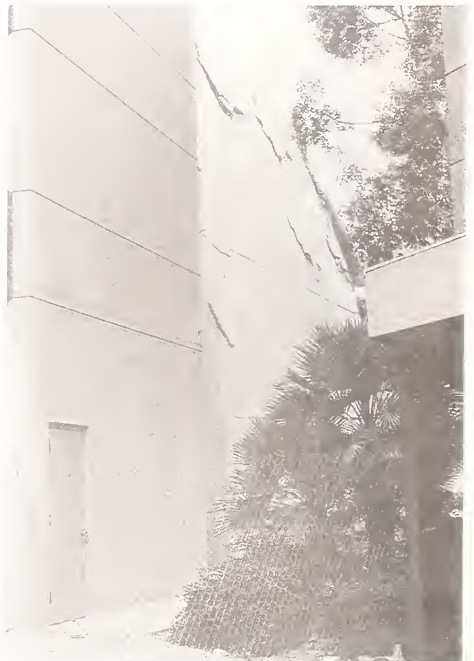
Figure 20 - At the east and west faces of the Kaiser Permanente Hospital parking garage, shear walls made up the lateral force resisting system. Both walls had horizontal cracks caused by the out-of-plane bending when the walls were pulled inward. Neither wall had major diagonal cracking, suggesting that the lateral load was never fully delivered to the walls. The stair towers remained erect. The east wall and stair tower are shown here.
