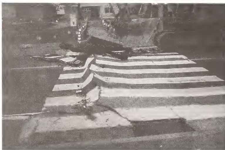
Photo 4.3 Crash and Uplift of Pavement (National Road 228)
