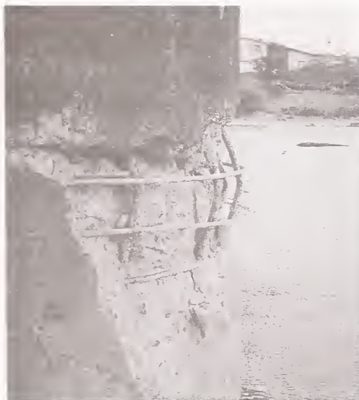
Photo 5.1 Damage of Pier P3 at Motoe Bridge
