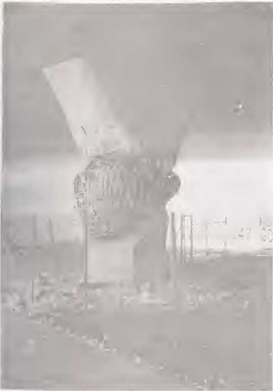
Photo 4.4 Shear Failure and Extensive Outward Deformation of Main Reinforcements (S-118 Mission/Gothic Undercrossing)
