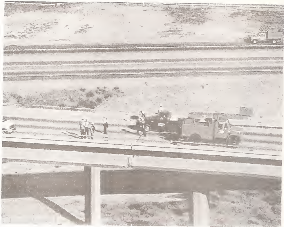
Figure 26 Example of pounding and offset at a hinge in the SR14/I5 interchange
