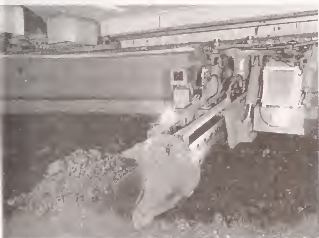
Plate - 5. The automatic excavator for Pneumatic caisson
