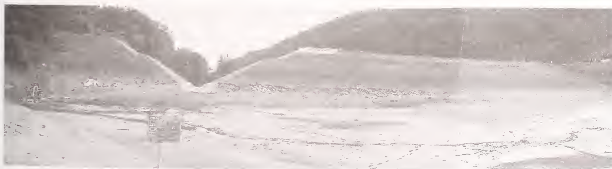
Photo.9 Channel Excavated as Emergency Work on the Niwa-Ikumine Dam (Photographed from the Reservoir Side on August 7, and by the Courtesy of the Kita-Hiyama Land Improvement District)
