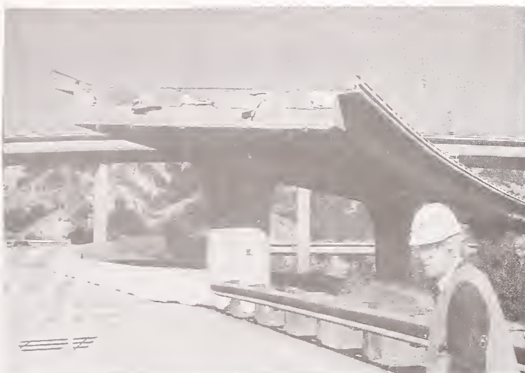
Photo 4.11 Failure of Cable restrainers at a Joint near P4
