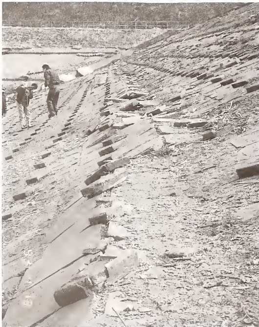
Photo.1 Raised Facing Concrete Blocks on the Upstream Slope Protection of Mombetsu Dam
