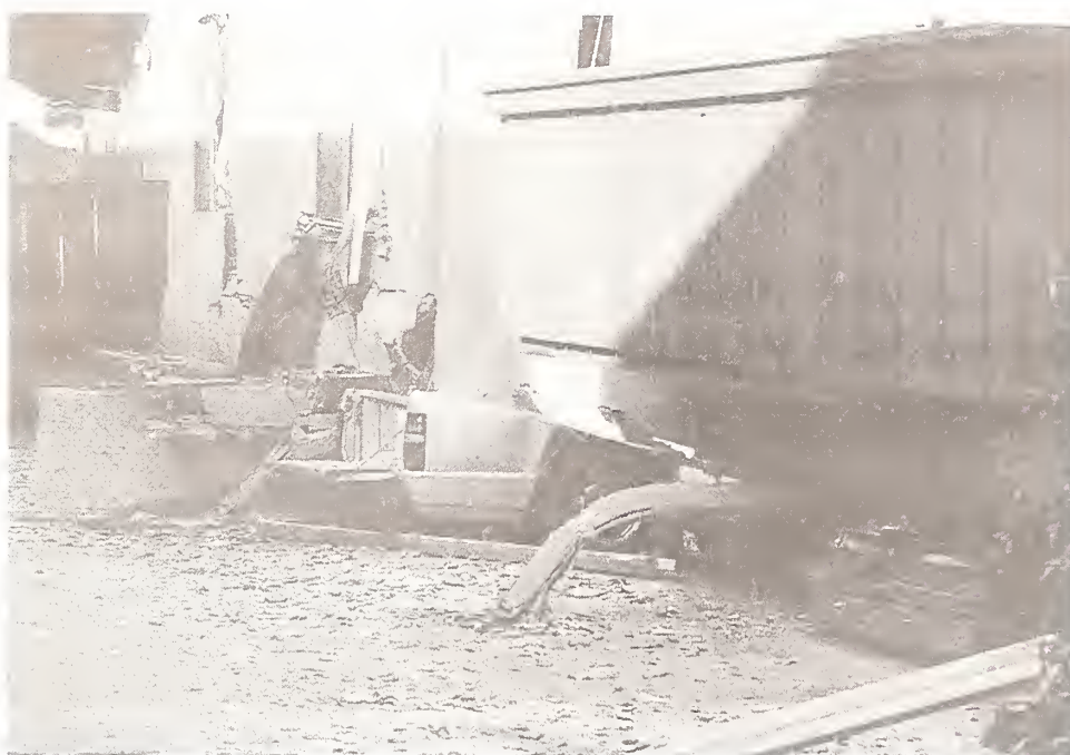
Figure 7 At Northridge Meadows, the first story steel pipe columns generally hinged near their bases but retained their length, controlling the displacement of the upper stories.
