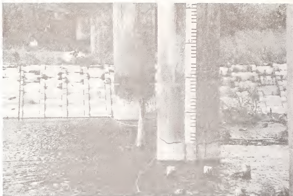
Figure 16B View of Assabu bridge piers--note cracking near waterline.
