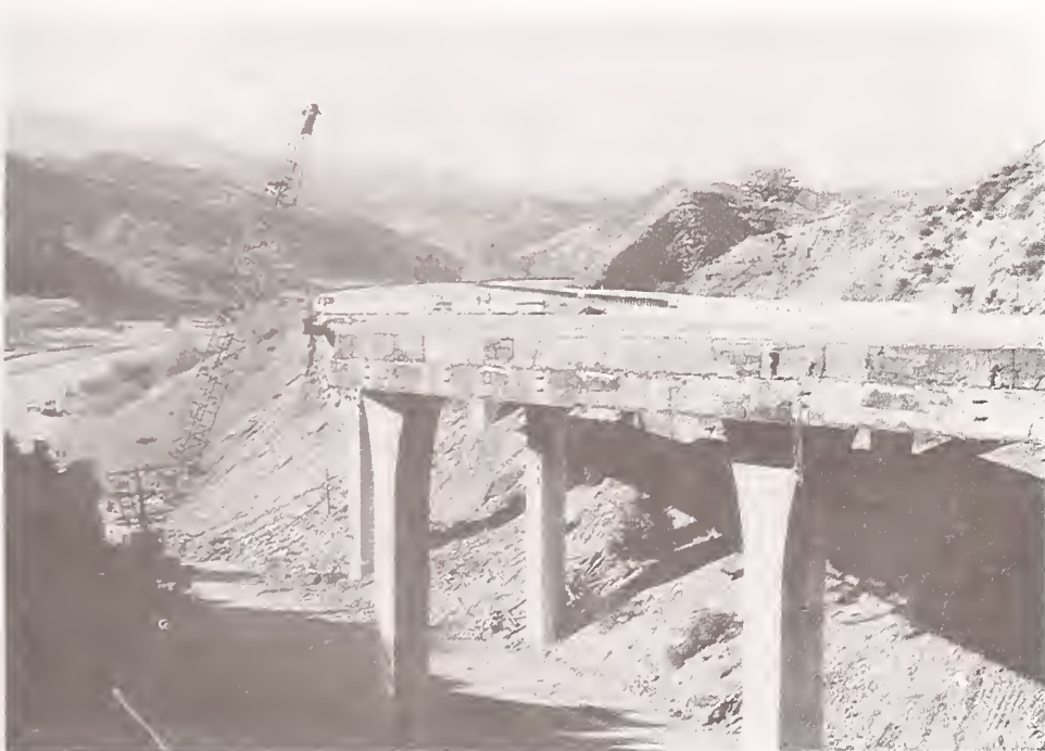
Figure 25 Ground level view of the southbound bridge at Gavin Canyon, looking to the northwest, showing the hinge bearing seat near Bent 3.
