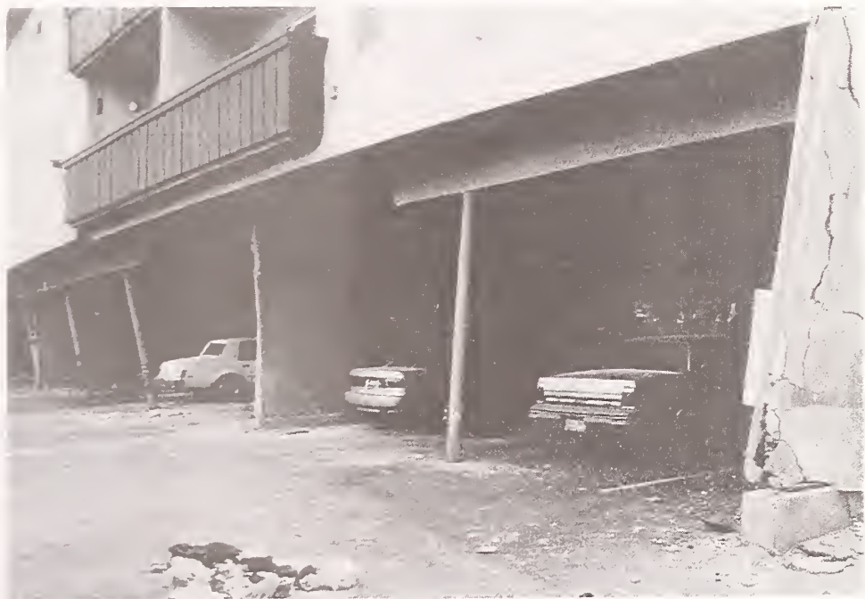
Figure 6 Steel pipe columns between parking bays supported the upper stories of the Northridge Meadows apartment buildings. Few of the buildings in the north half of the complex collapsed, but all were damaged.
