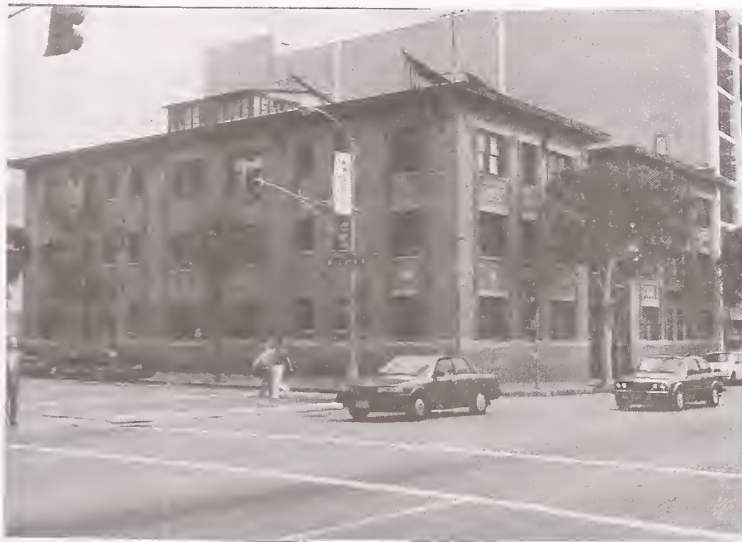
Photo 5.5 A Retrofitted Unreinforced Masonry Building in Santa Monica (This building suffered no damage)
