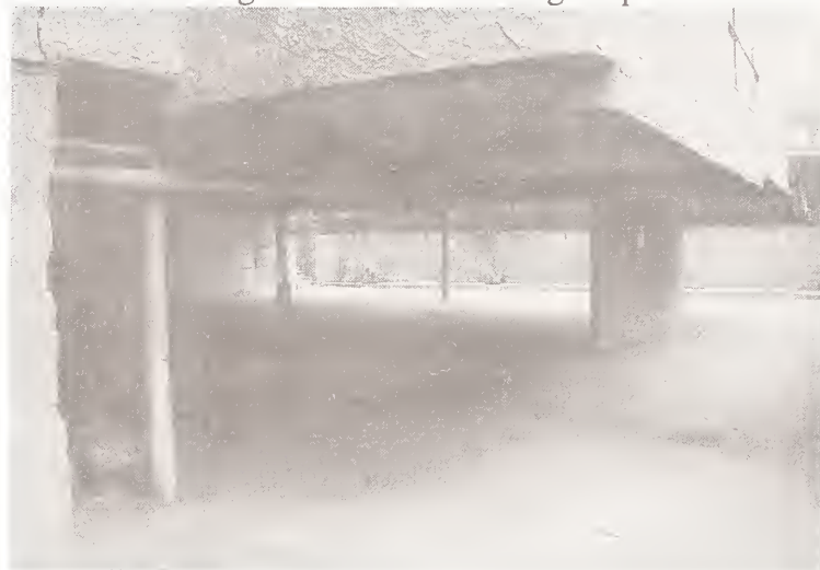
Photo 5.3 Basement Floor of an Apartment in Hollywood (To provide require parking spaces required, number of columns and walls at the basement floor is small)
