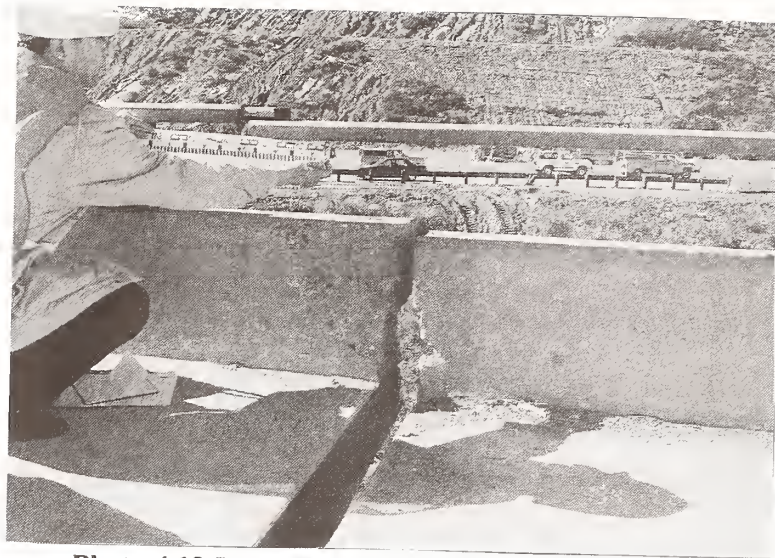
Photo 4.13 Large Separation Developed at Hinge
