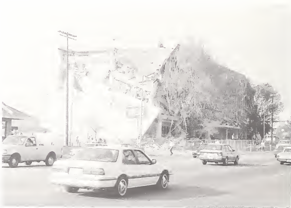
Figure 3.42. Both end walls of the Kaiser Permanente building slid, partially intact, to the ground. The south wall is pictured here. Both ends of the building suffered damage to the concrete frame at all story levels, while the middle half of the building, except for the second story, remained intact.
