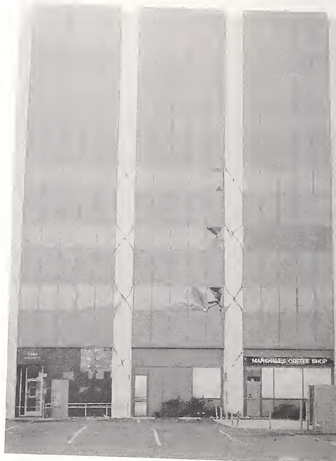
Figure 3.46. The stiff infill panels of the Barrington Building effectively shortened the concrete columns, forcing all the displacement into the column sections bounded by windows. Diagonal X-cracking decreased in severity towards the top of the building.
