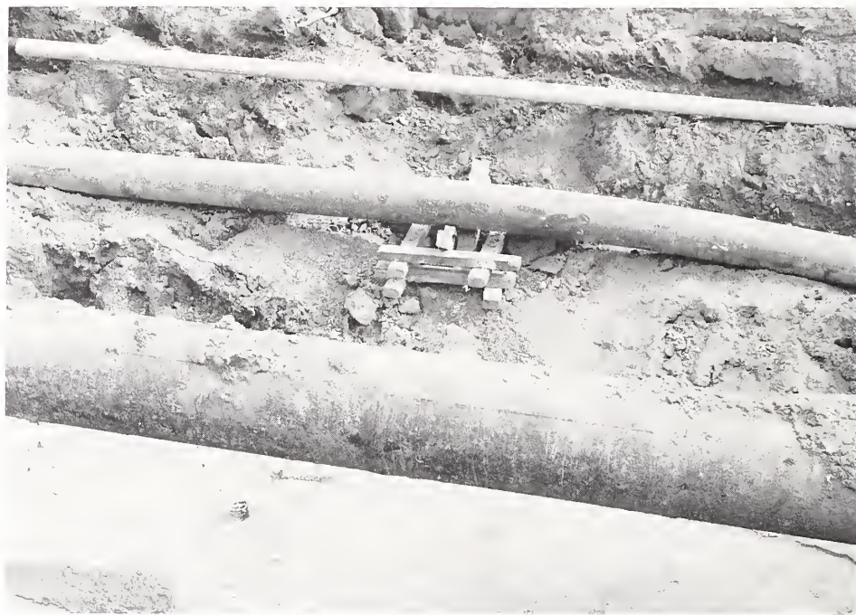
Figure 5.14. Some of the buried pipelines located near the intersection of Balboa Boulevard and Bircher Street showing the potential hazard of co-location of lifeline systems. At this site are three water lines (two of them main lines); three gas lines; two sewers; one crude oil line; overhead power, telephone, and cable TV lines; the street lighting system; and the street itself.
