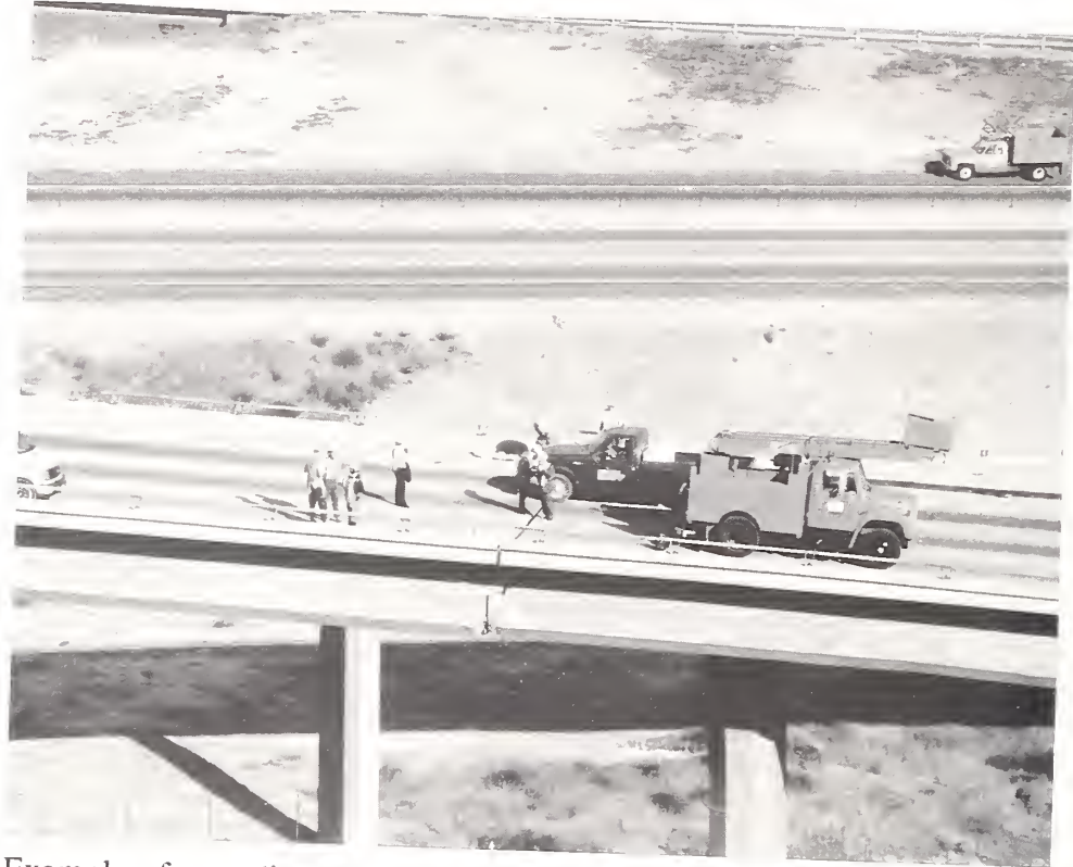
Figure 4.7. Example of pounding and offset at a hinge in the SR14/I5 interchange.
