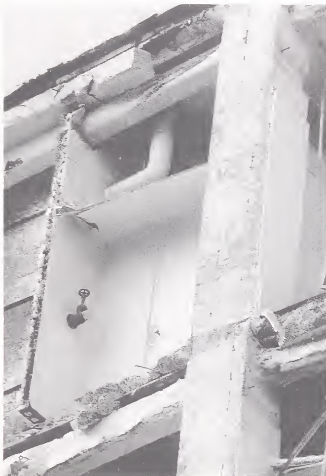
Figure 3.51. The exposed structure of the Sherman Way office building shows remains (at the floor level and the column) of the minimal ties that anchored the masonry facade.
