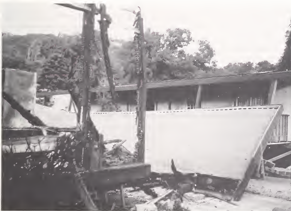
Figure 6.10. Collapsed roof which acted as a fire break in a manufactured housing development.
