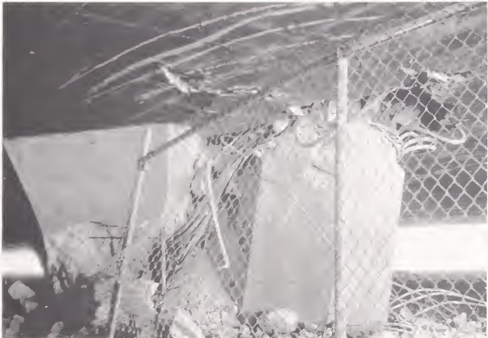
Figure 4.22. Damage to a pier of the SR118 Mission-gothic Undercrossing, looking to the west at Bent 4 of the eastbound bridge, which collapsed (Photo courtesy of EERC).
