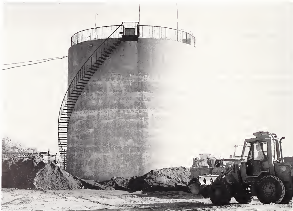
Figure 5.2. The reinforced concrete surge tank at Terminal Hill performed well during the earthquake--no damage was observed.
