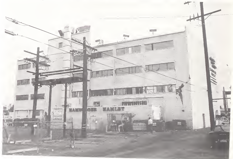
Figure 3.58. The reinforced masonry facade of this steel-framed building in Sherman Oaks was badly damaged.
