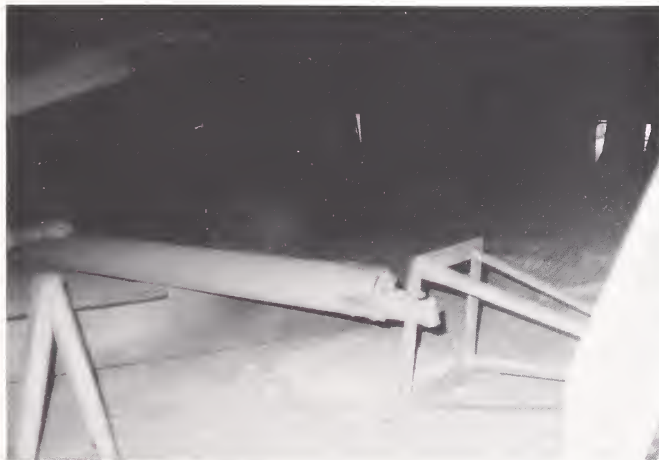
Figure 3.22. The metal supports under many homes tipped over, bringing down the houses above.
