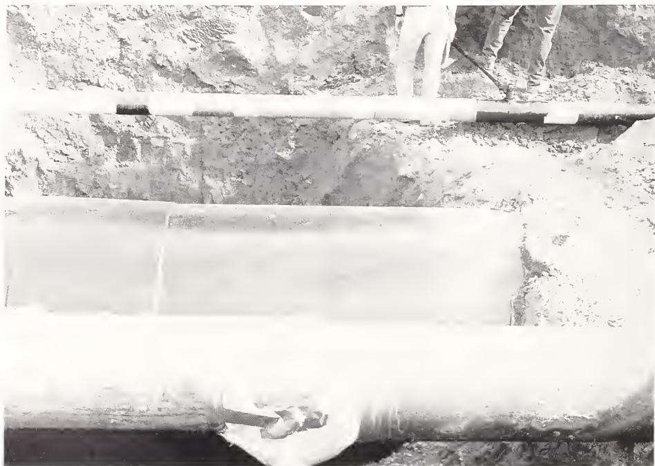
Figure 5.10. Ground contraction along Balboa Boulevard caused the rupture of a gas distribution line (top), the Rinaldi trunk 1.8-m (68 in) water main (center), and a gas main (bottom). The pipes were being repaired at the time this photograph was taken.
