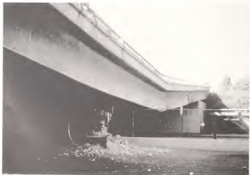
Figure 4.44. View of collapsed span of I10 over Fairfax Ave.; note rotation of girder over Pier 2 (Photo courtesy of EERC).
