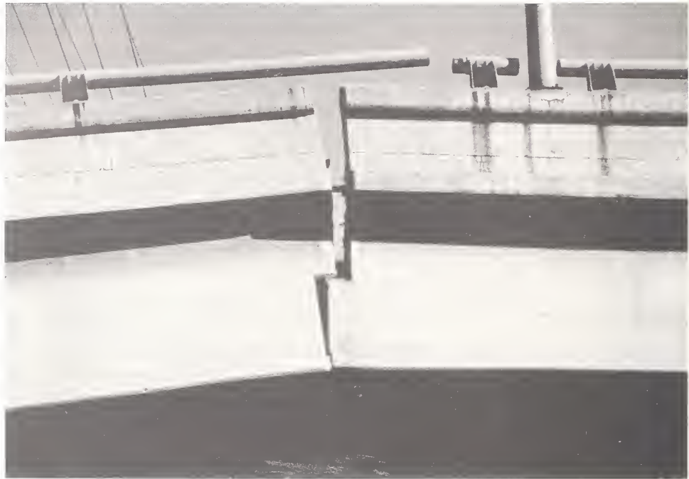
Figure 4.43. Hinge adjacent to Bent 4 of I 10 at Fairfax Ave.; cable restrainers prevented loss of support (Photo courtesy of EERC).
