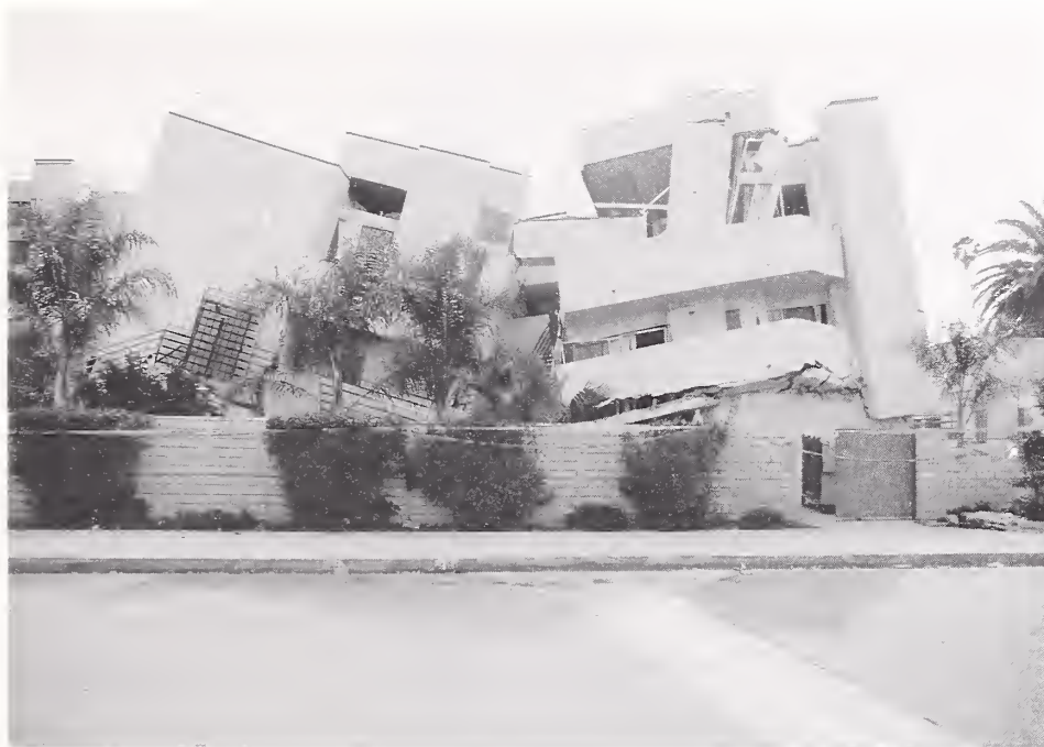
Figure 3.10. The central row of concrete first-story columns in a three story apartment building on Sherman Way in Van Nuys collapsed, causing the wood-framed upper stories to settle inward.
