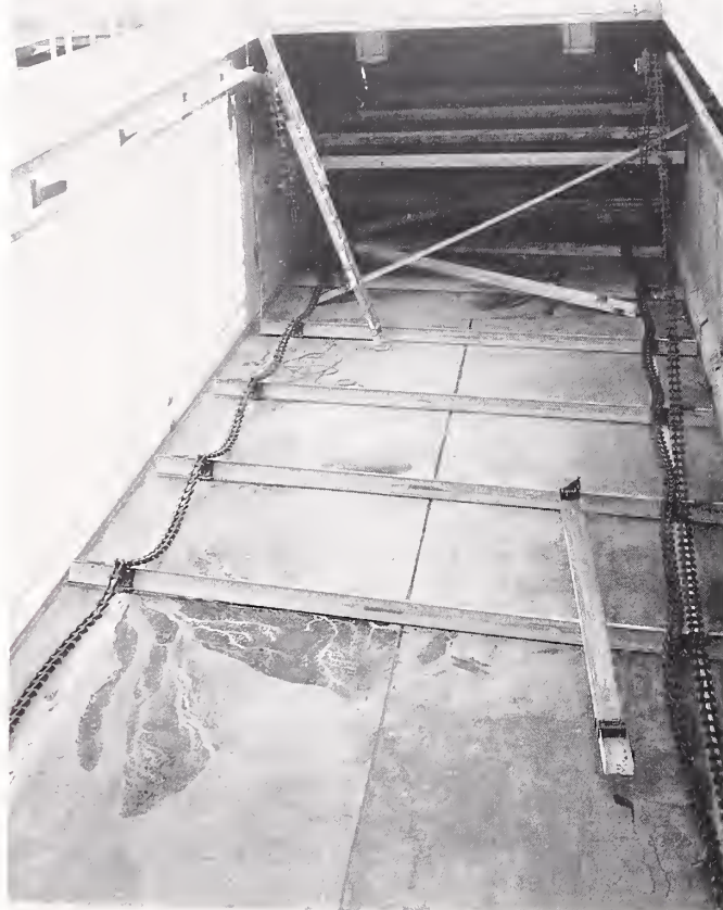
Figure 5.7. A damaged sludge scraper in a clarifier tank at the Tillman Water Reclamation Plant.
