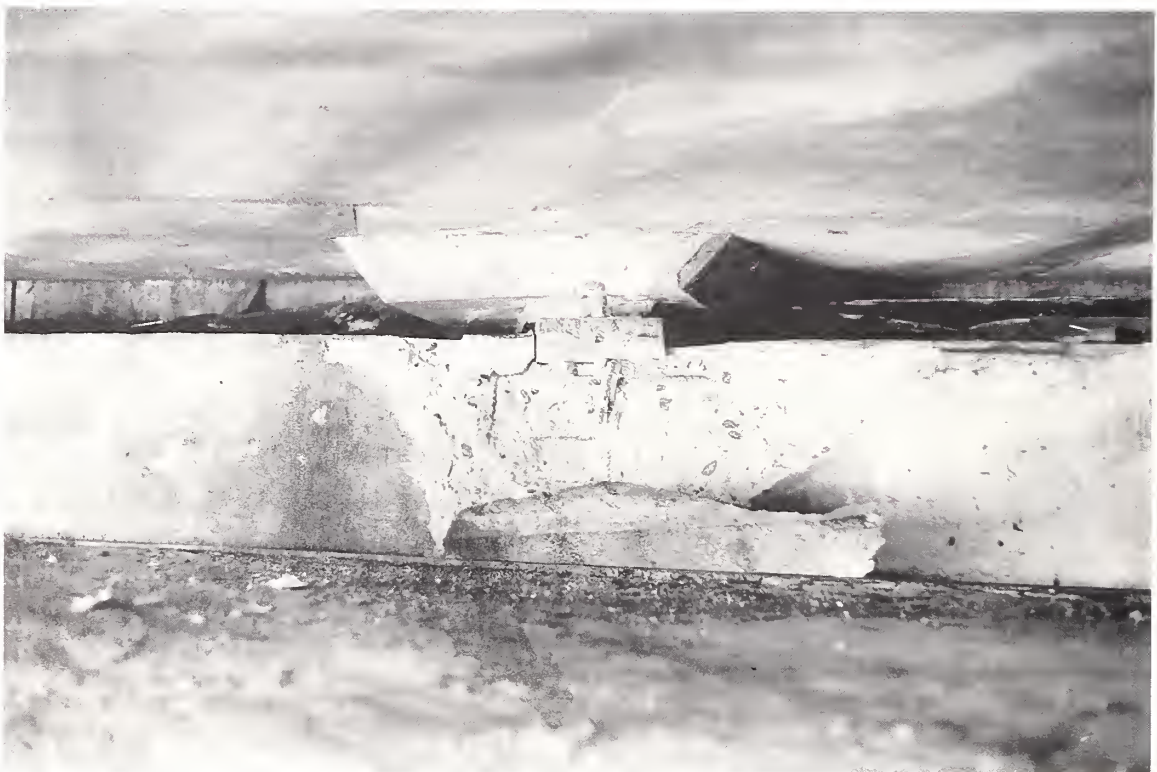
Figure 4.48. Abutment damage at sliding-type bearing.
