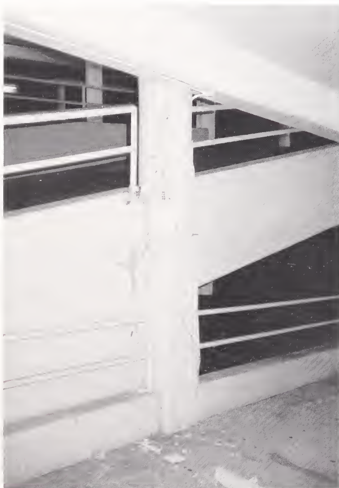
Figure 3.67. In parking garages, ramps can cause unintentionally shortened columns, which are vulnerable to damage, as shown here.
