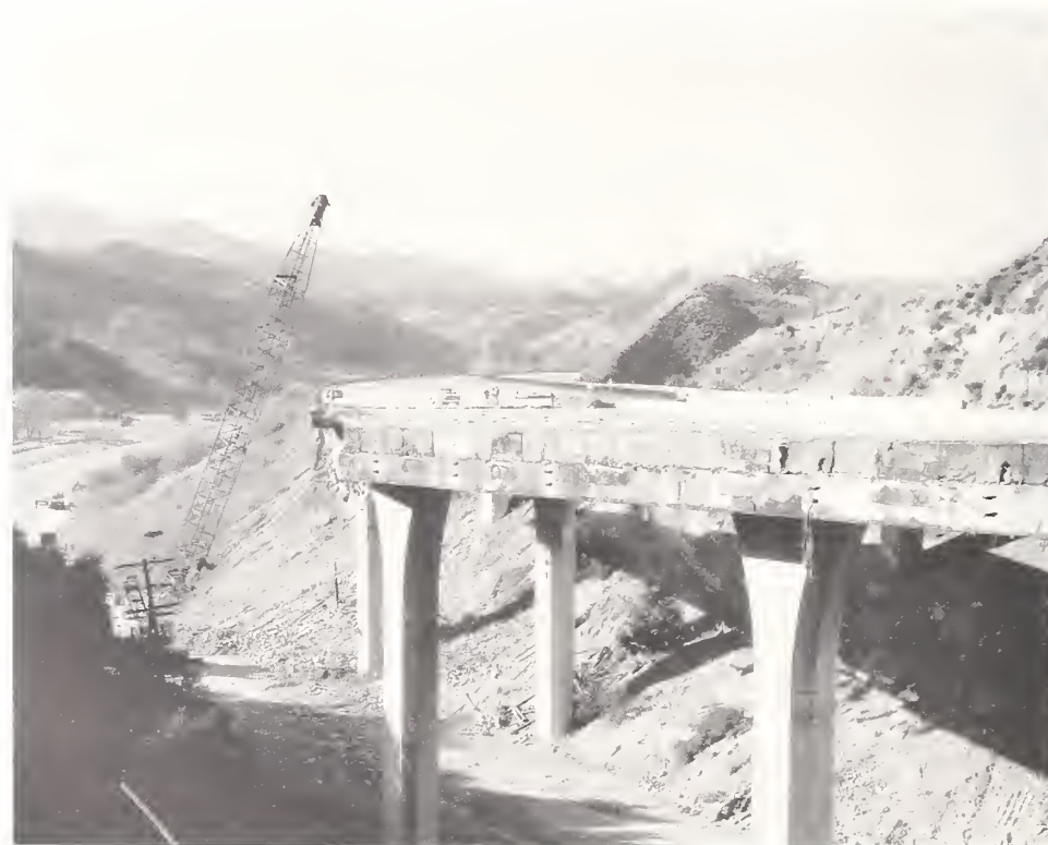
Figure 4.3. Ground level view of the southbound bridge at Gavin Canyon, looking to the northwest, showing the hinge bearing seat near Bent 3.
