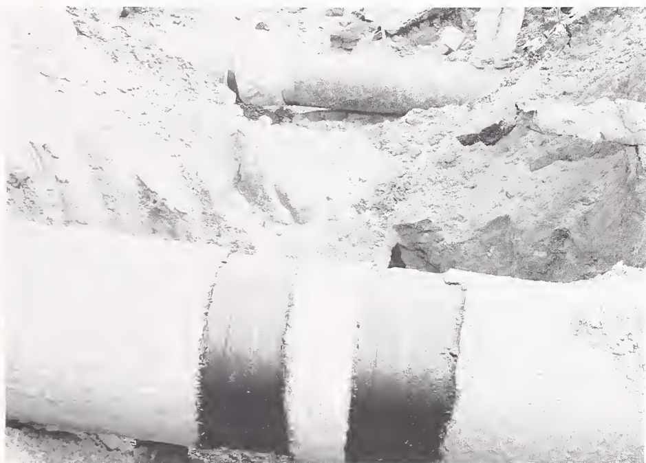
Figure 5.11. Ground extension along Balboa Boulevard resulted in the rupture of the same gas main shown in figure 5.10 (top) and a 1.2-m (48 in) water main (bottom). The rupture of the gas main here caused a major fire that engulfed five houses.
