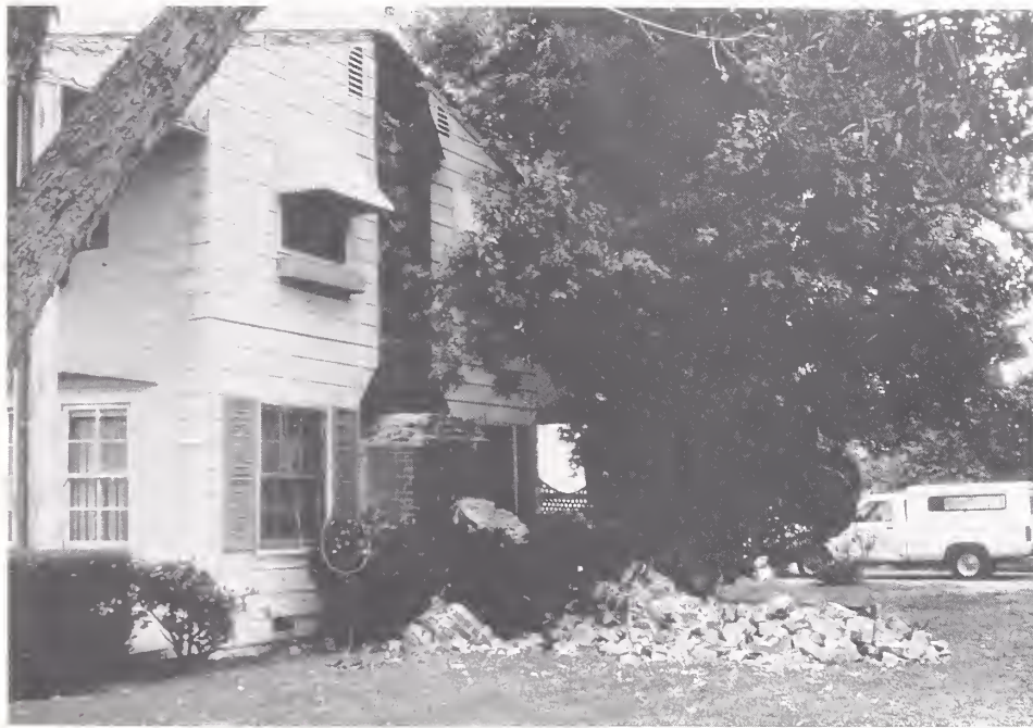
Figure 3.17. Failure of masonry chimneys was common.
