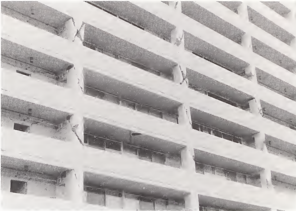
Figure 3.14. The back of the Champagne Towers building was badly damaged. The railings here are solid infill, which effectively stiffen the lower half of the columns. The shortened upper half of the columns were forced to accommodate all the displacement, and they failed in shear.
