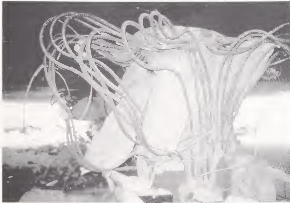
Figure 4.45. Failed column in Bent 3 of I10 at Fairfax Ave. (Photo courtesy of EERC).
