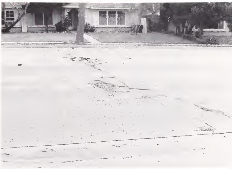
Figure 5.19. Transverse cracks in pavement along Balboa Boulevard in Northridge area.
