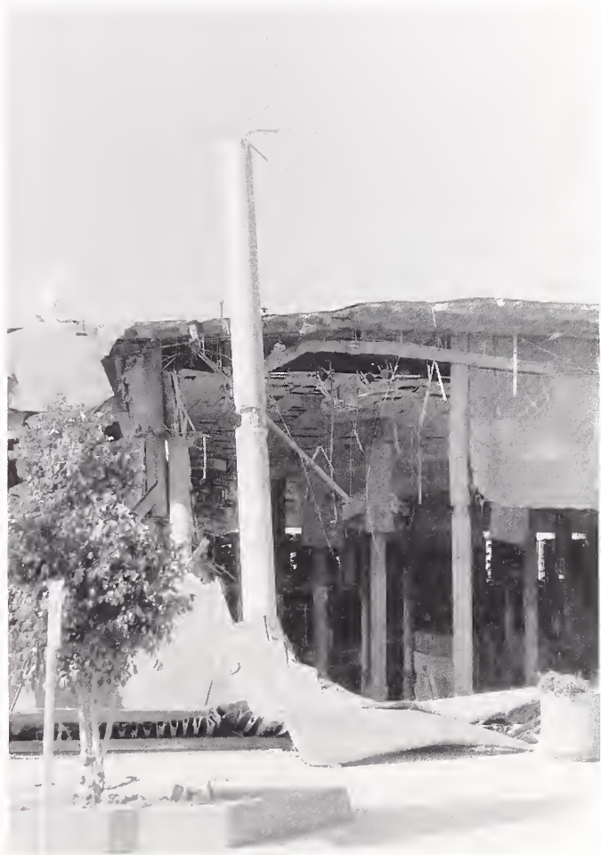
Figure 3.29. A portion of the concrete waffle slab roof and the interior floor slabs at the Bullock's department store at the Northridge Fashion Center mall fell to the basement, leaving many of the columns standing. No reinforcing steel can be seen in the remaining columns that would have connected the columns to the floor slabs.
