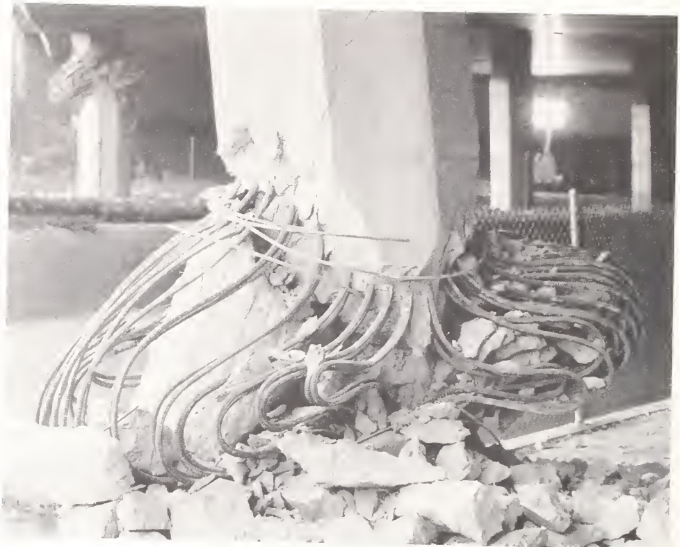
Figure 4.27. Damage to pier 3S-1 of State Route 118 at Bull Creek Canyon Channel, looking to the northwest.
