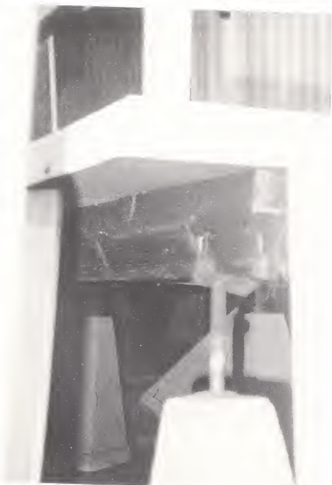
Figure 3.20. Small concrete base supports are a common foundation system used to support manufactured housing. This type of system provided little resistance to lateral forces.
