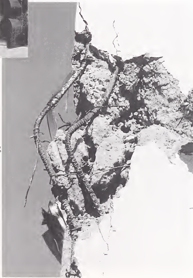
Figure 3.48. A close up of the damaged southeast corner of the Barrington Building shows the widely spaced, undeformed bars used for transverse reinforcement.
