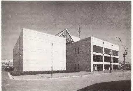
View of the acoustic and environmental vibration test building. (Left - base isolation building; Right - building with conventional technique).
