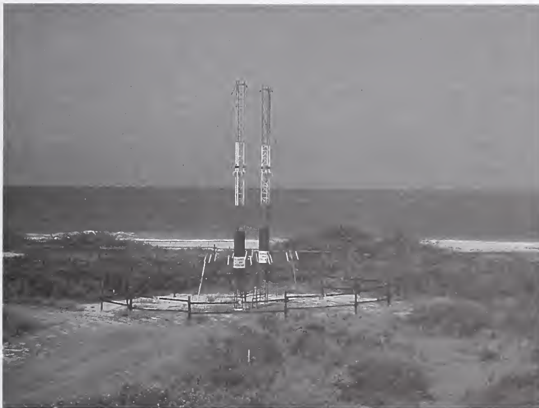
Figure 1.29. 15 MHz antenna at WWVH.
