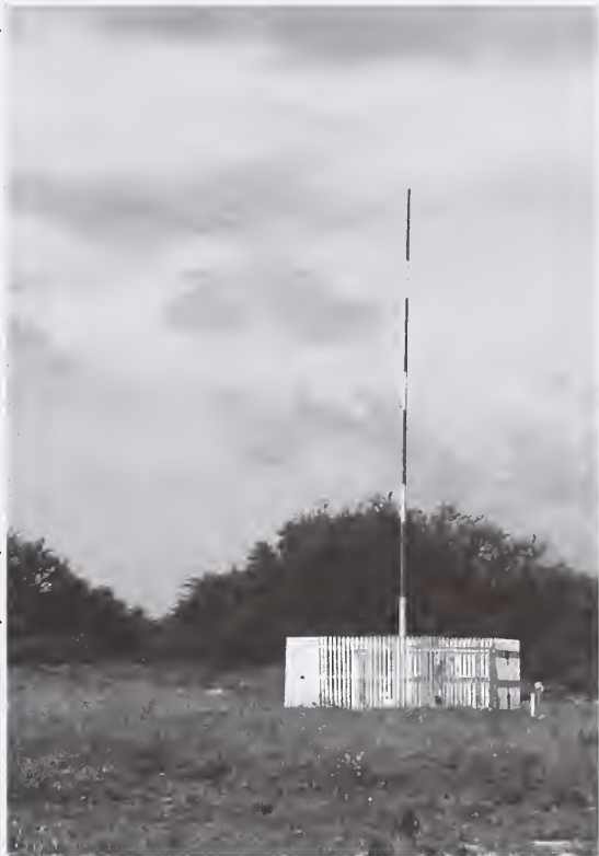
Figure 1.27. Fiberglass whip antenna at WWVH.
