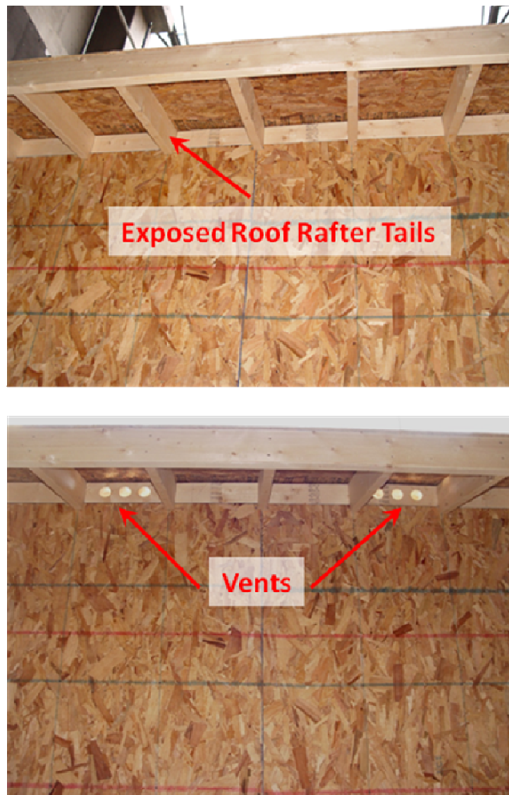
Figure 18 Images of open eave construction with no vents (top) and vents (bottom).
