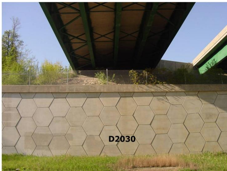
Figure B.53 Individual Elements: D2030 Earth Retention System
