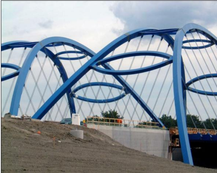
Figure C.6 Transverse View of the Arch Ribs Illustrates Unequal Lengths
