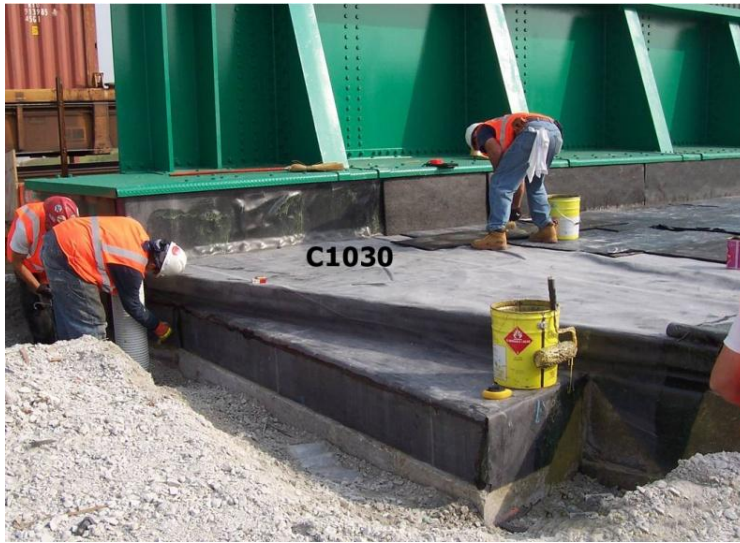
Figure B.36 Individual Elements: C1030 Protection Coats
