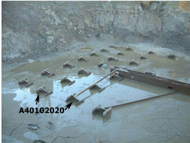
Figure B.18 Individual Elements: A4010 Thrust Blocks (Sub-Elements: A401020 Foundations (A40102020 Piles))
