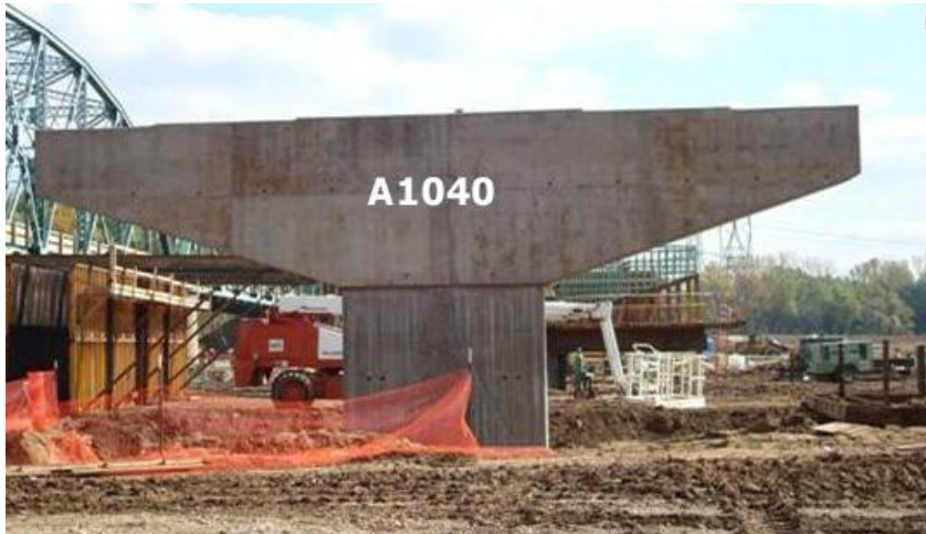
Figure B.10 Individual Elements: A1040 Cap Beams
