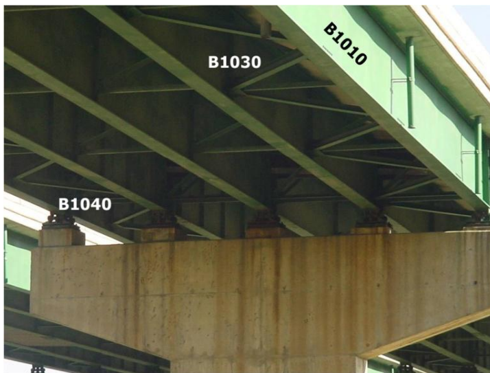
Figure B.25 Individual Elements: B1010 Flexural Members, B1030 Bracings, B1040 Bearings
