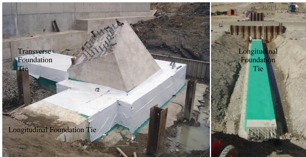
Figure C.4 Gateway Arch Bridge Foundation System
