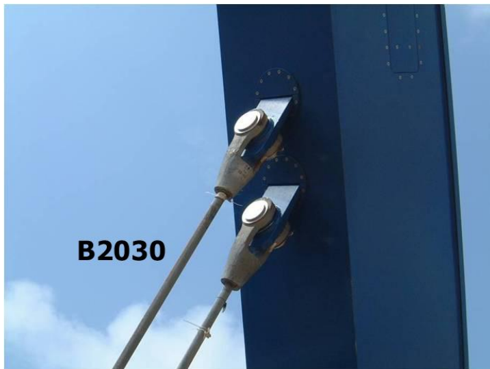
Figure B.27 Individual Elements: B2030 Hangers
