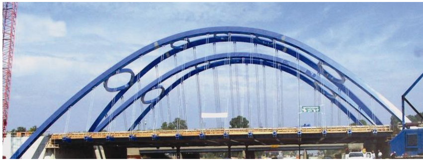
Figure C.5 Longitudinal View of the Arch Ribs
