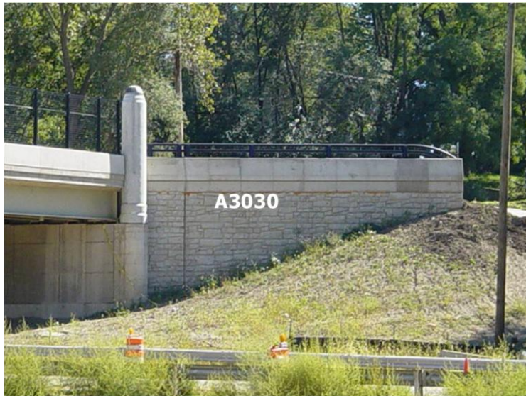
Figure B.16 Individual Elements: A3030 Wing Walls
