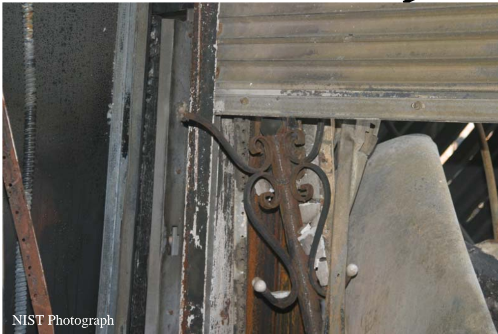
Figure O-54. Main showroom roll-down fire door looking toward rear of main showroom. Movement of door impeded by coat rack. Door only closed about one-third of the way.
