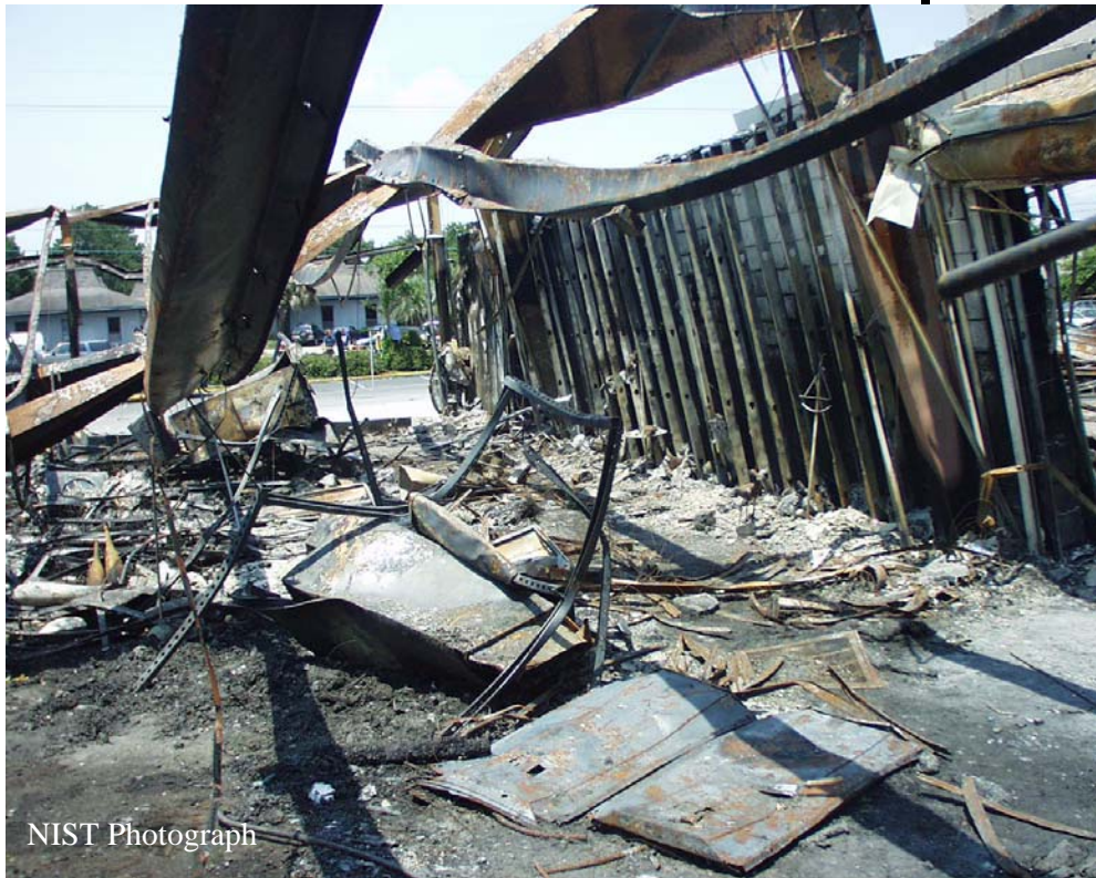
Figure E-29. Interior of west showroom along east wall toward front of store. Open roll-down fire door visible at right of photo.
