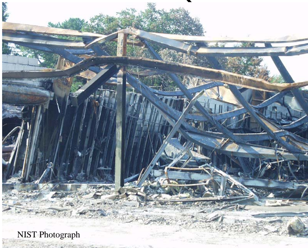
Figure E-13. Exterior view of west showroom looking into east-front portion of showroom. Metal stud wall attached to west wall of main showroom visible in center of photo. Open roll-down fire door partially visible at left center of photo.
