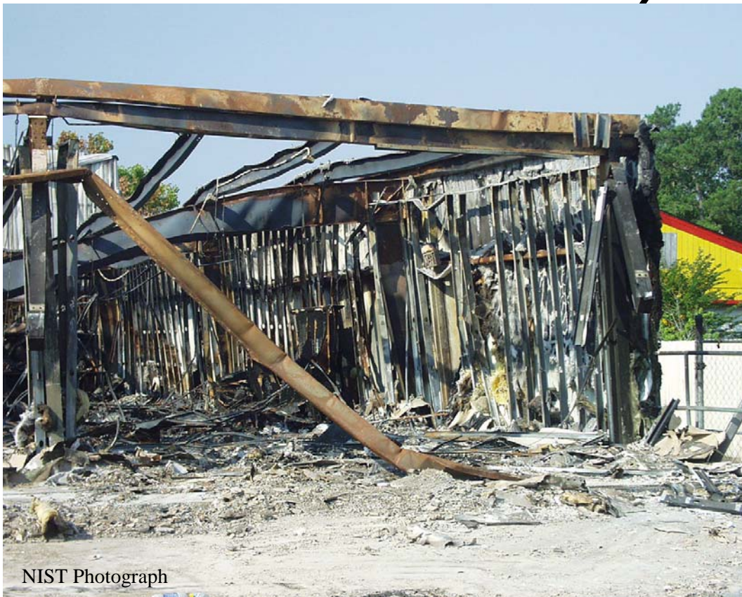
Figure E-14. Exterior view of west showroom looking into north-west corner of showroom. Vertical metal studs of interior wall visible in photo. Yellow automobile repair garage visible in right center background.
