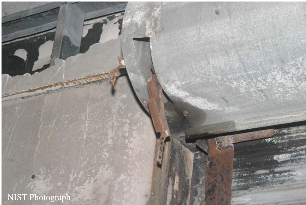
Figure O-45. South side of operating mechanism for roll-down fire door #6. Portion of fusible link visible in center of photo.
