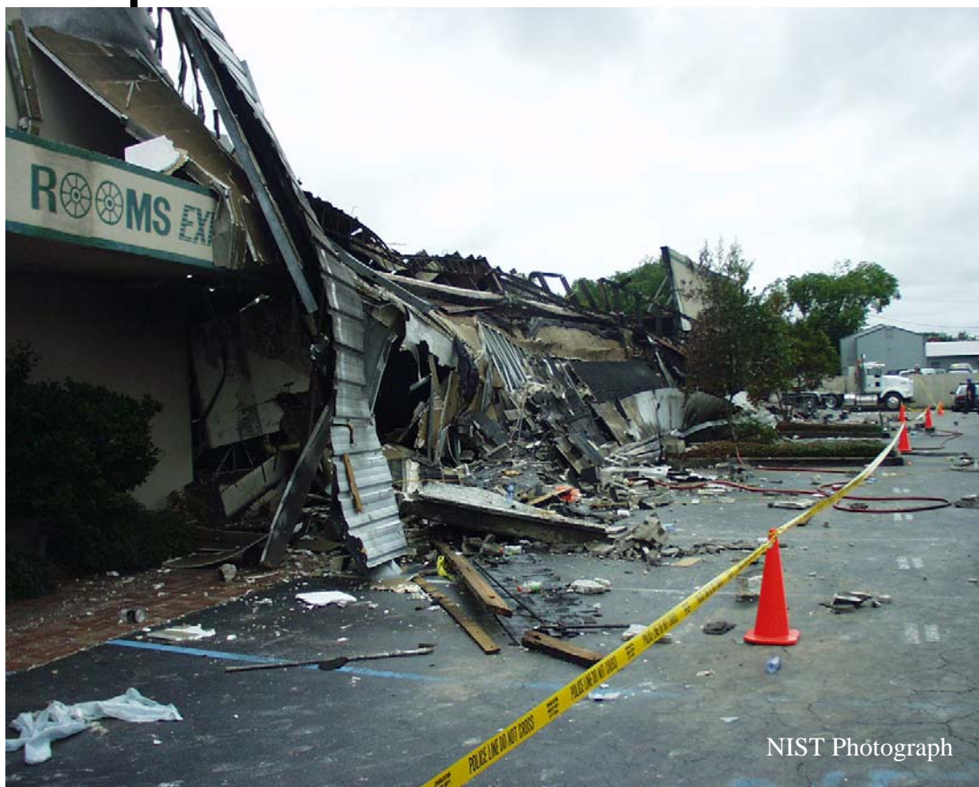
Figure D-3. Front of main showroom. Facade and parapet wall of main showroom collapsed into parking spaces.
