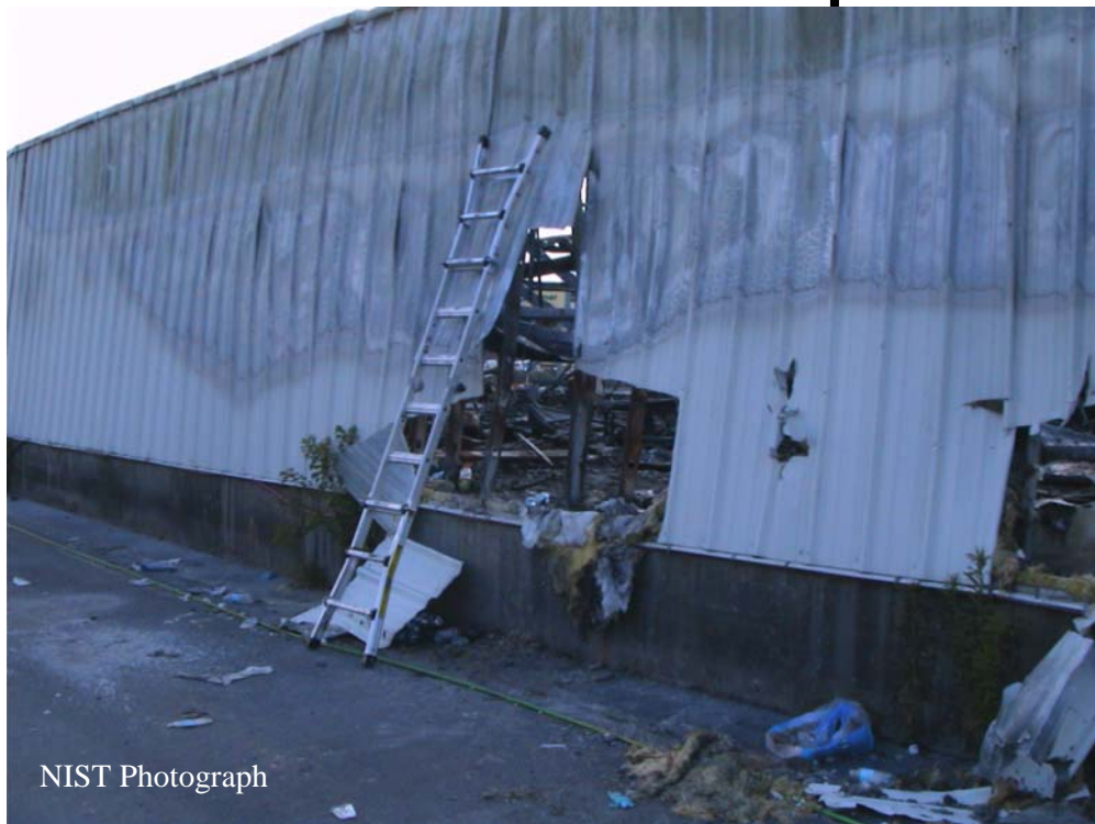
Figure E-9. Exterior of west wall of west showroom. Discoloration of metal siding visible at top of wall. Fire department cut access holes through metal siding during the fire.
