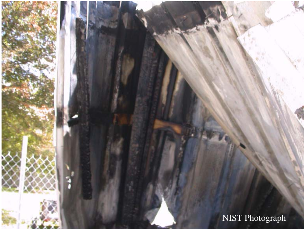
Figure H-6. Wood frame of repair shop.
