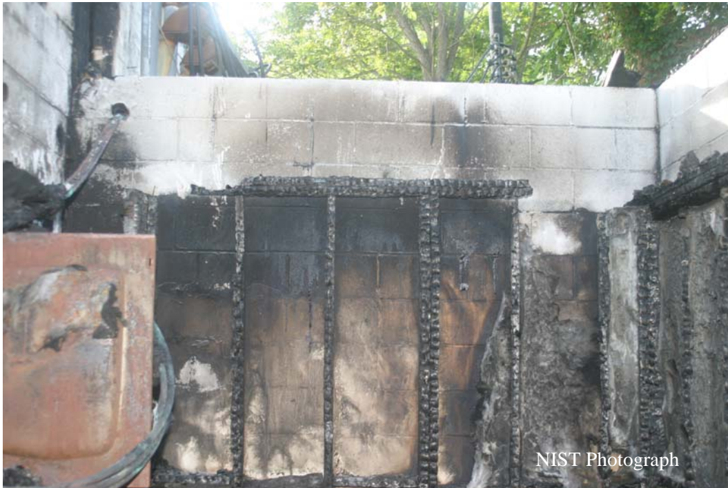
Figure I-6. Interior view of enclosed area at rear of main showroom. Doorway that was filled with concrete block is located beyond rusty metal electrical panel cover in left of photograph.
