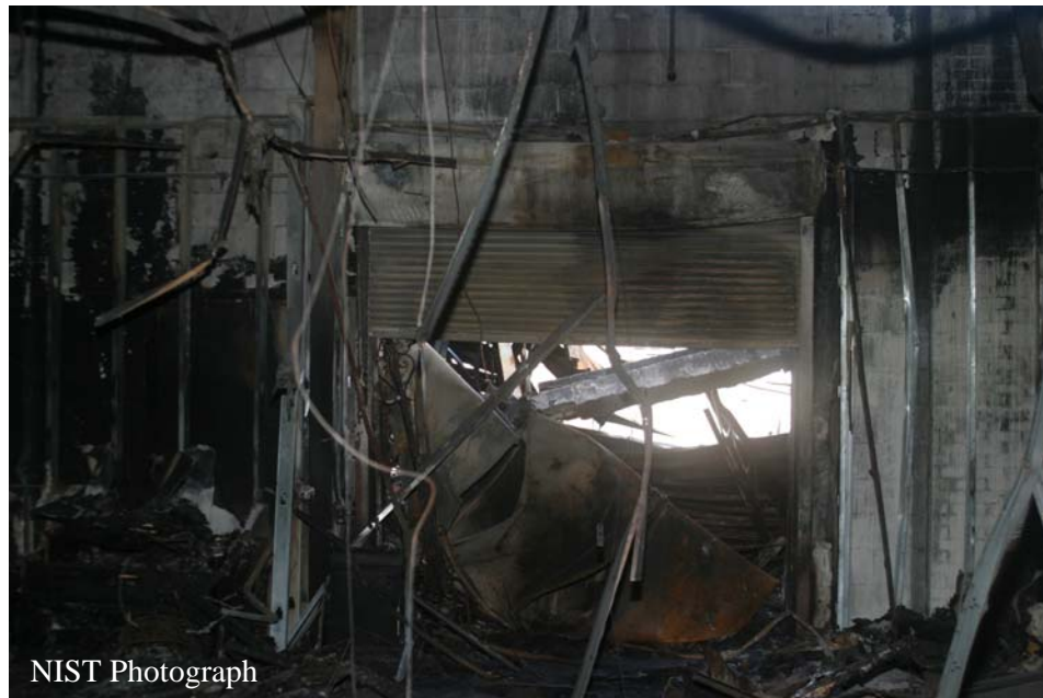
Figure O-48. Main showroom roll-down fire door looking toward rear of main showroom. Door identified as roll-down fire door #7 in Figure O-1. Door only closed about one-third of the way down during the fire.
