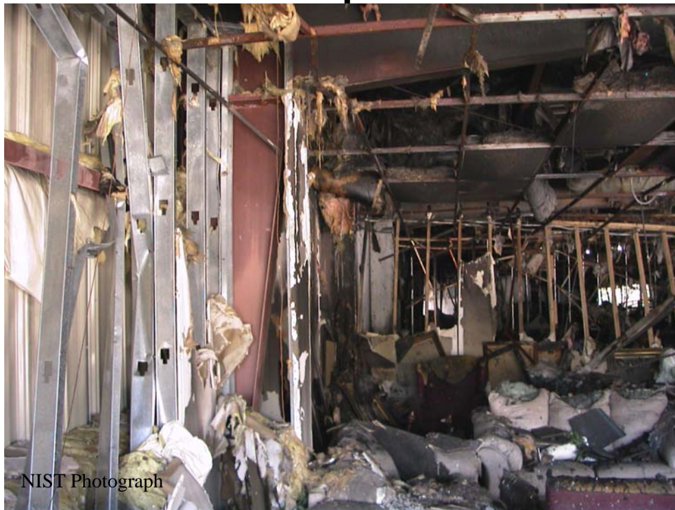
Figure F-21. Interior of east showroom looking along east wall toward rear of showroom. Exterior metal wall attached to exterior side of horizontal channel. Metal studs attached to inside face of horizontal channel. Gypsum wall board was installed over metal studs to form interior wall of showroom. Metal stud/gypsum wall appeared to extend approximately 0.3 m ( 1 ft) above drop ceiling along east wall. Reddish-brown steel I-beam column and roof beam also visible in photo.
