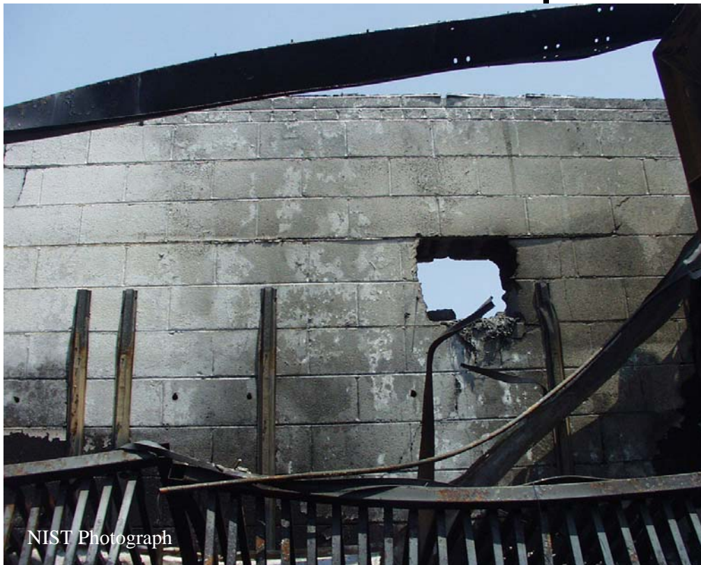
Figure E-26. Interior of west showroom above suspended ceiling looking toward main showroom. Open hole, approximately 0.5 m (1.5 ft) x 0.5 m (1.5 ft) opening through concrete block wall. This hole may have allowed smoke to move from interstitial space above suspended ceiling in main showroom to the interstitial space above the suspended ceiling in the west showroom.
