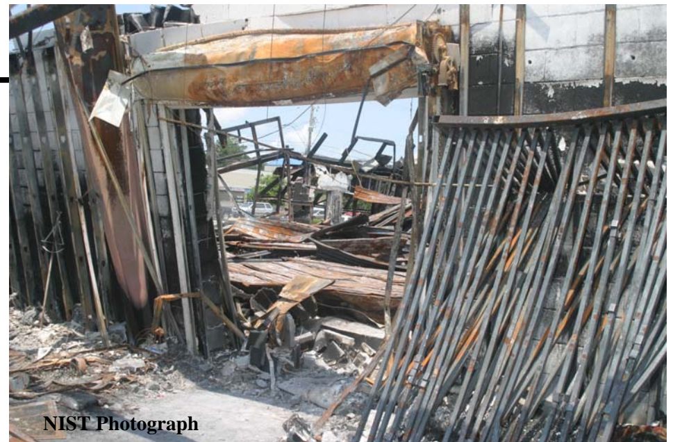
Figure O-22. Main showroom roll-down fire door looking toward middle of main showroom. Door identified as roll-down fire door #3 in Figure O-1.
