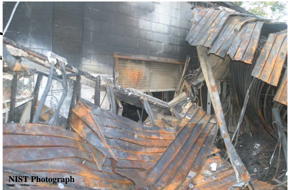
Figure O-55. Main showroom roll-down fire door looking toward rear of east showroom. Door identified as roll-down fire door #7 in Figure O-1. Door only closed about one-third of the way down during the fire.
