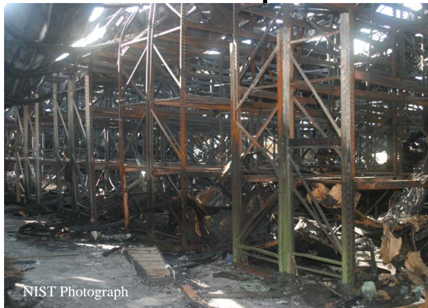
Figure G-16. High rack storage units inside warehouse.
