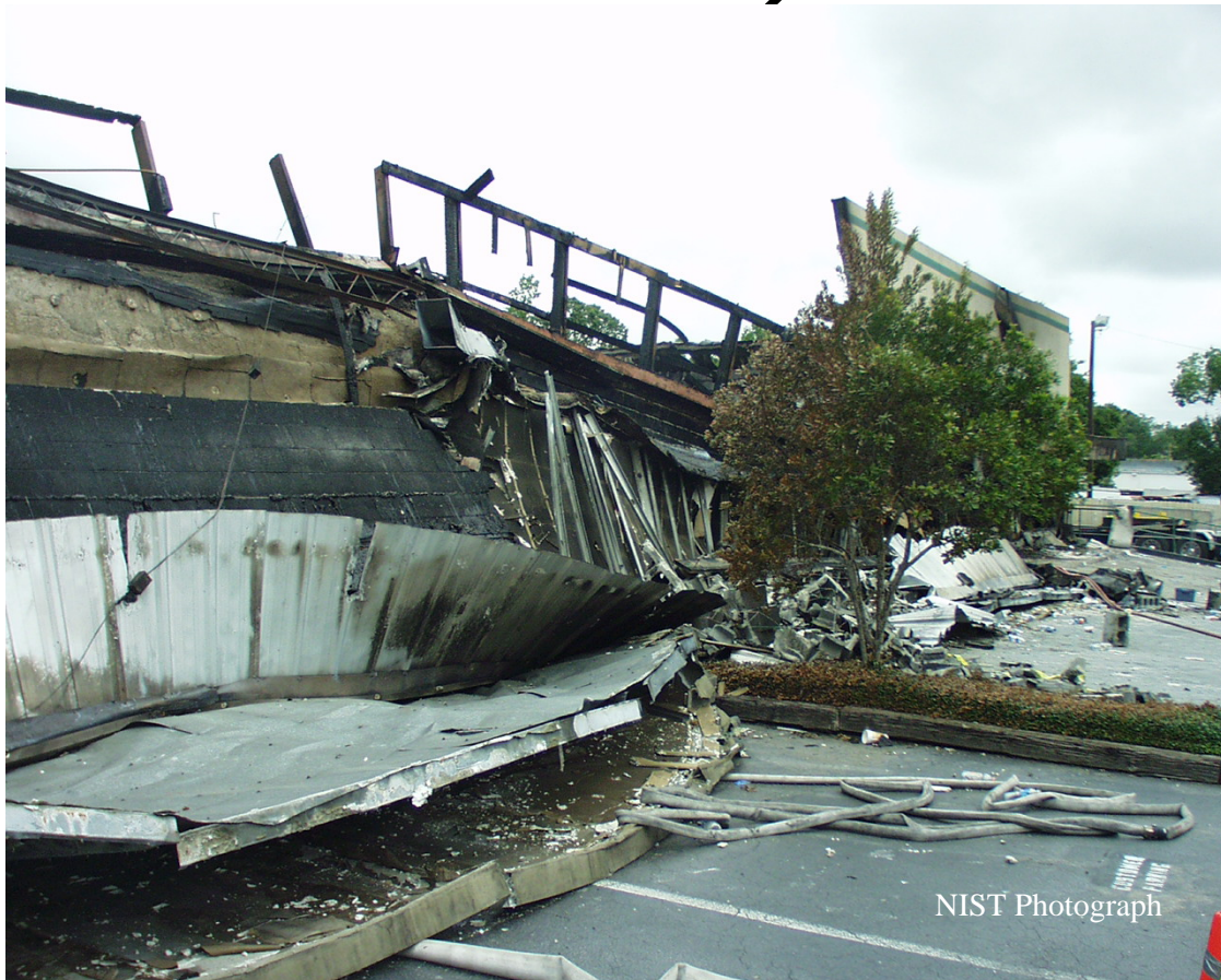
Figure D-2. Front of main showroom. Façade and parapet wall of main showroom collapsed into parking spaces.
