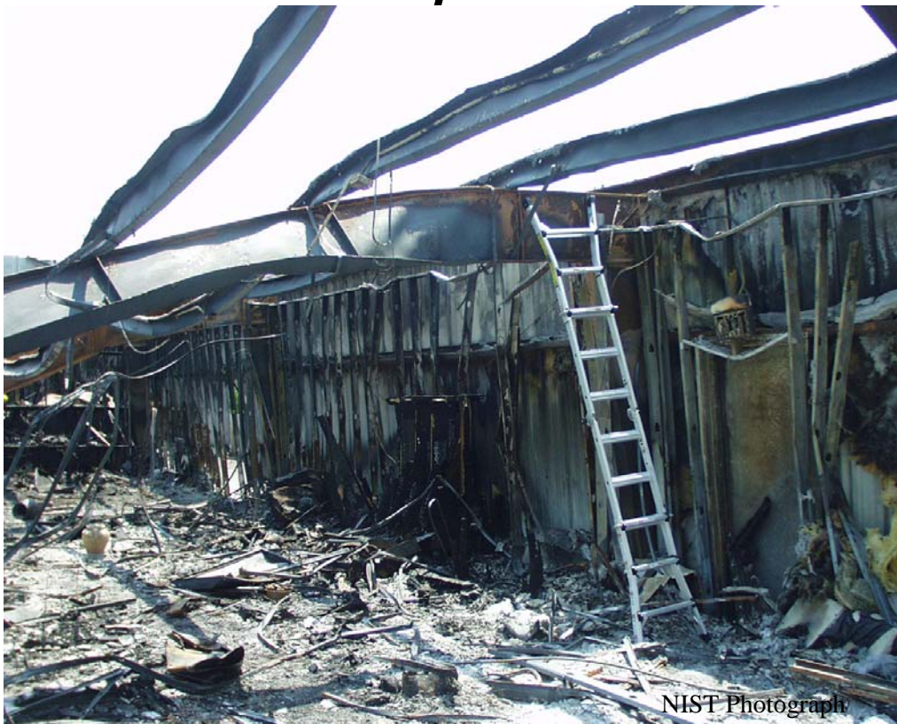
Figure E-17. Interior view of north-west corner of west showroom. Sagging I-beam and roof Z-channel visible in photo. Exit door in west wall near front of showroom visible to the right of ladder.
