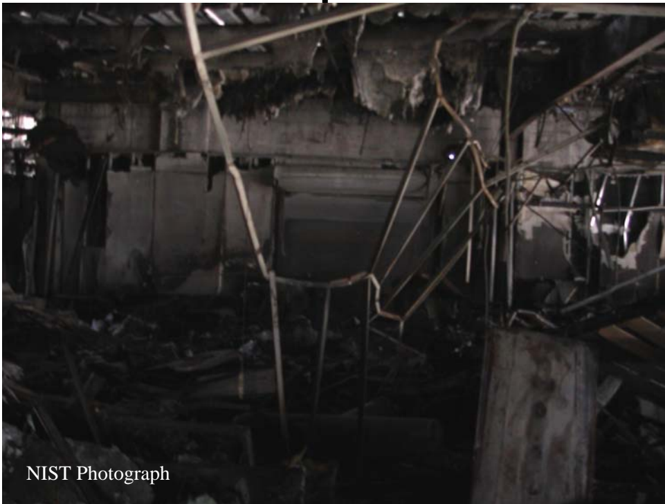
Figure F-15. Interior of east showroom looking toward main showroom. Closed roll-down fire door visible in center of photo. Photo displays more damage from fire in this center section of east showroom.
