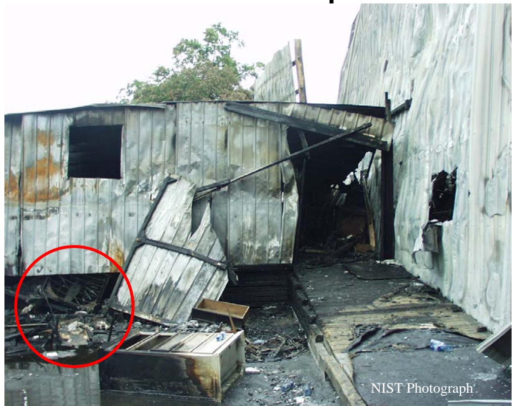
Figure C-4. Right side of west wall of loading dock. Inclined ramp led from warehouse loading dock. Fire ignited in pile of trash outside loading dock (within red circle).
