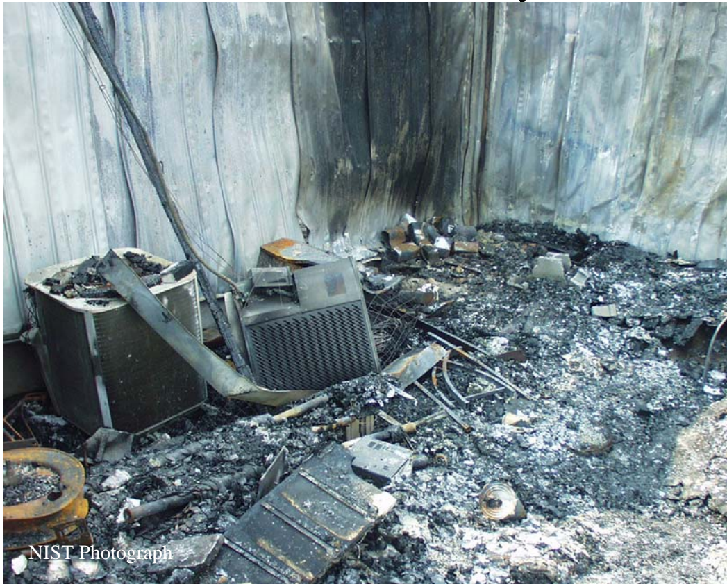
Figure C-18. Intersection of breezeway wall and north wall of warehouse. Heat pumps were located in small courtyard area between loading dock and breezeway wall. Gallon containers of hydrocarbon solvent can be seen at base of breezeway wall.
