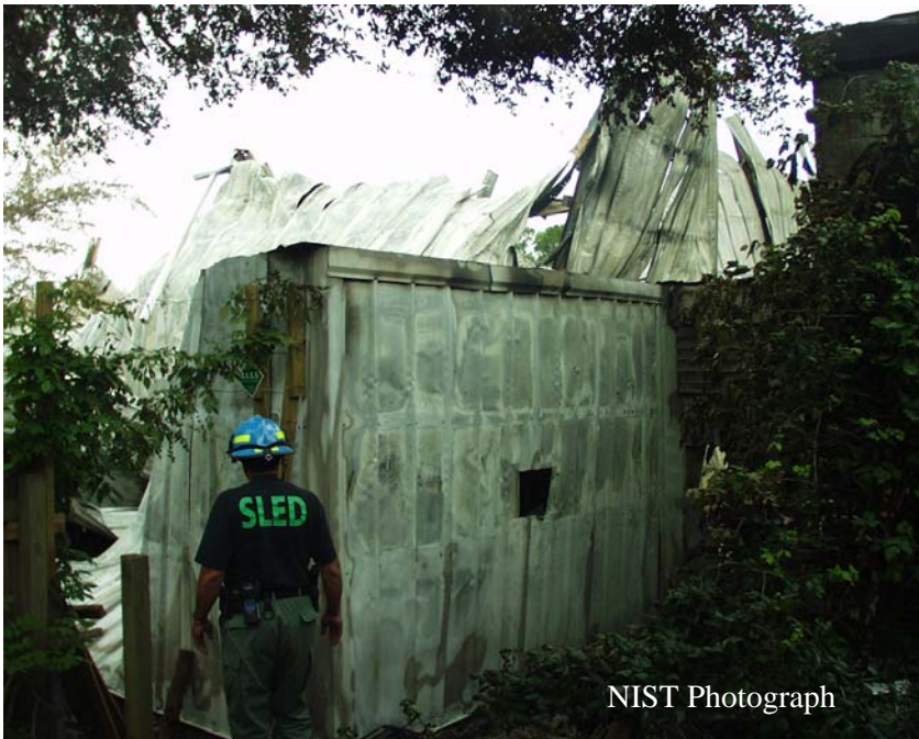
Figure H-2. North wall of repair shop looking toward warehouse, from rear of main showroom. Air conditioner was mounted in small rectangular hole in center of wall.
