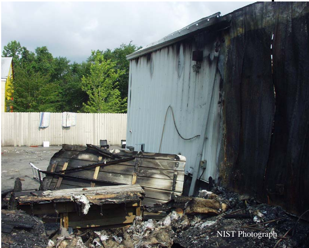
Figure C-15. Loading dock floor in foreground. Rear wall of west showroom on right of photograph. Darker section of rear wall was inside the enclosed loading dock area. Lighter portion of wall was outside enclosed loading dock.
