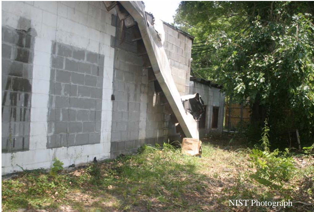
Figure I-7. Rear wall of main showroom. Openings in wall have been filled with concrete block. Wood fence is visible in center right of photograph.
