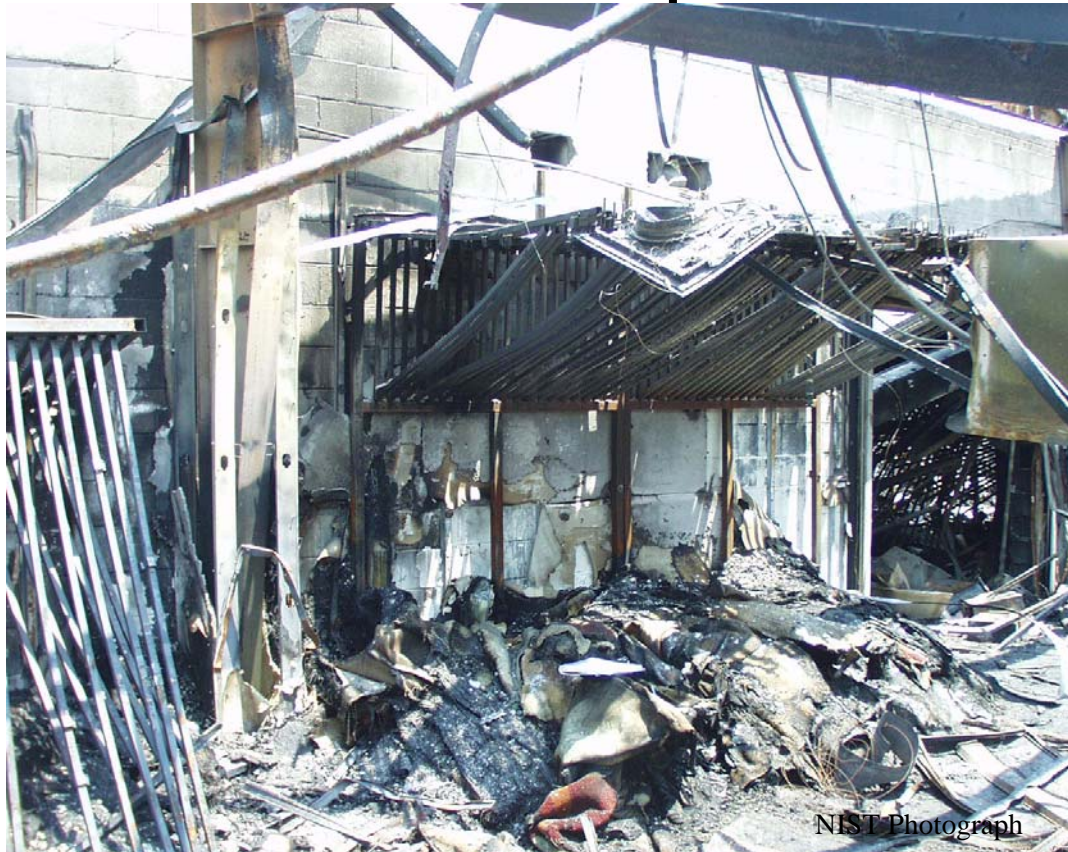
Figure E-25. Area rug support racks in west showroom. Open roll-down fire door visible on right of photo.
