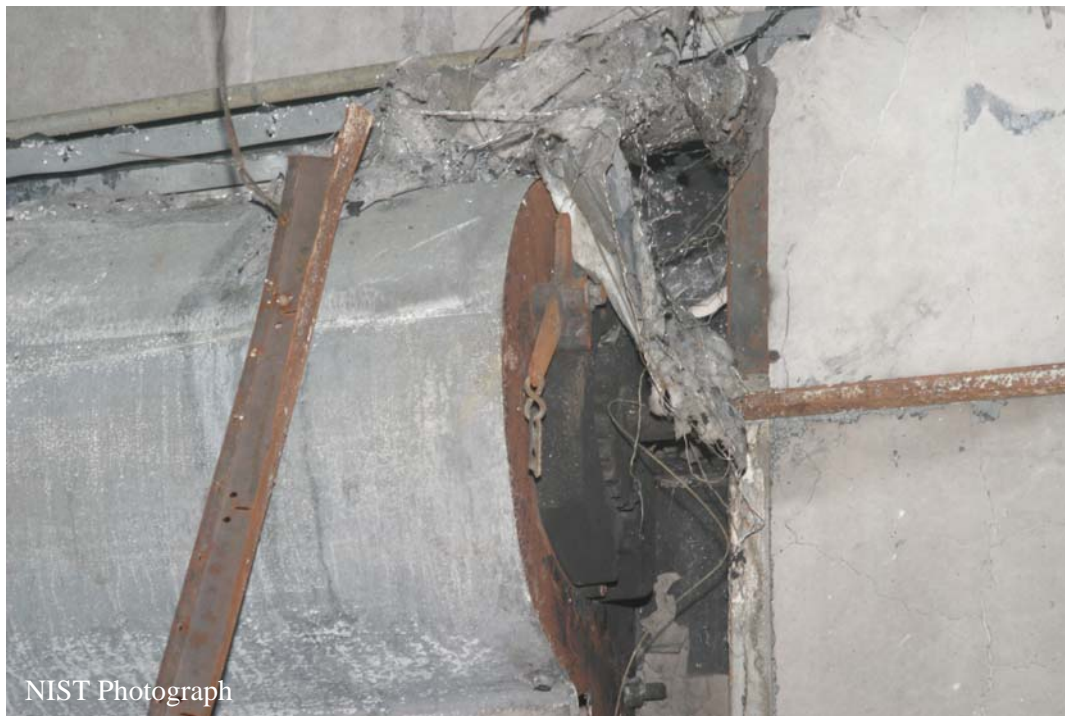
Figure O-43. North side of operating mechanism for roll-down fire door #6. Portion of fusible link visible in center of photo.
