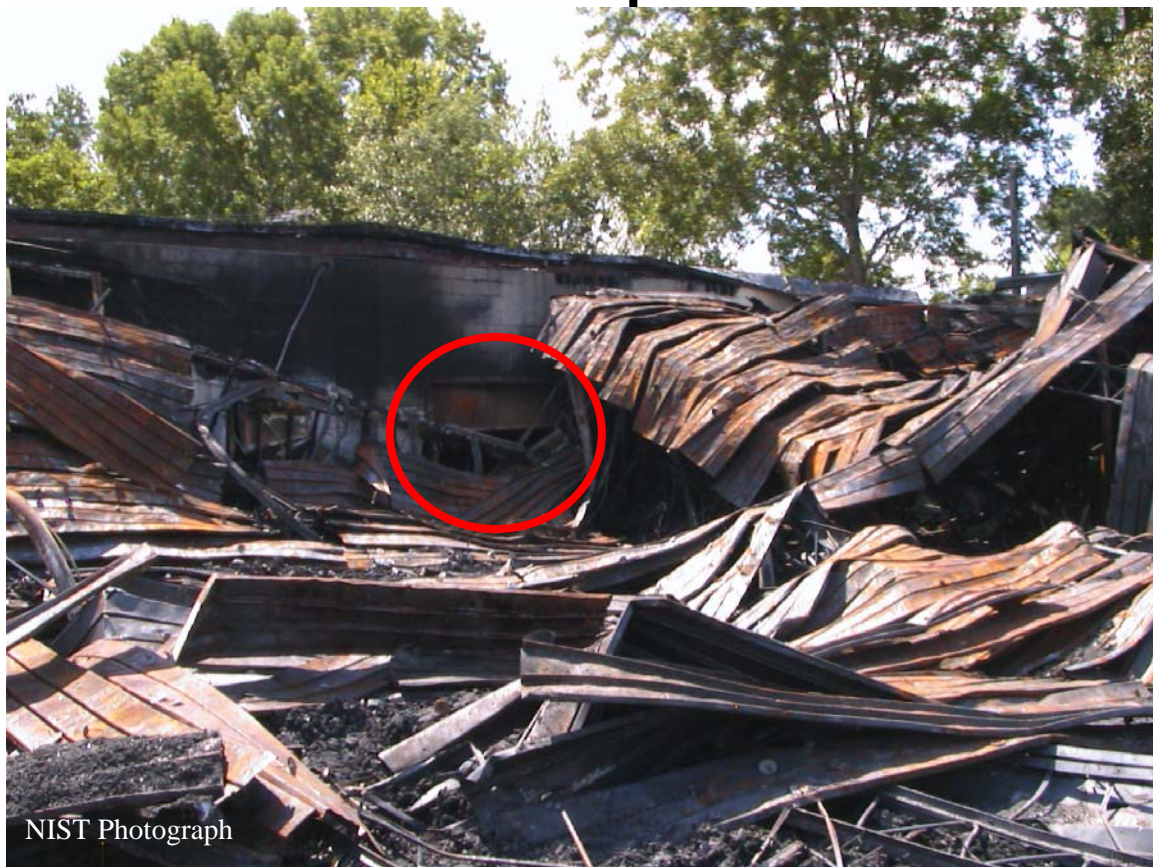
Figure D-23. Interior of main showroom looking toward east wall. Partially closed roll-down fire door circled.
