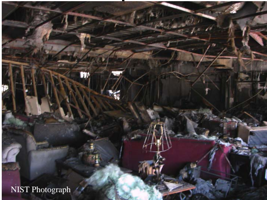
Figure F-14. Interior of east showroom looking toward main showroom. Closed roll-down fire door visible in center-right background. Partially closed roll-down fire door visible in center background. Photo displays less fire damage to furniture in front section of east showroom.
