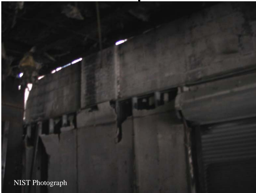
Figure F-20. Interior view of east showroom looking toward main showroom. Concrete block wall was originally exterior wall of grocery store. Gypsum wall board attached to metal stud which were attached to concrete block wall. Metal studs/gypsum wall board extended up to suspended ceiling, but not above suspended ceiling.
