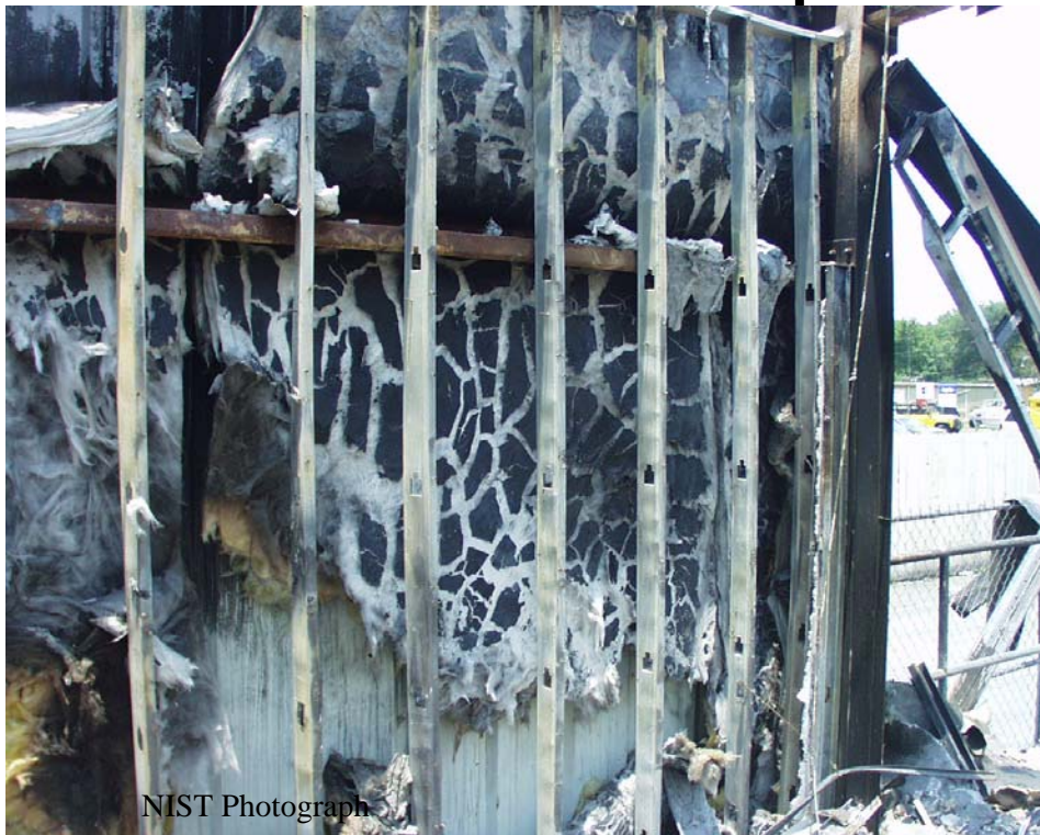
Figure E-31. Interior of west showroom looking at west wall near front of store. Exterior metal wall attached to exterior side of horizontal channel. Metal studs attached to inside face of horizontal channel. Gypsum wall board was installed over metal studs to form interior wall. Metal stud/gypsum wall appeared to extend approximately 0.3 m (1 ft) above suspended ceiling along west wall. Fiberglass insulation is visible between metal studs and exterior metal siding.
