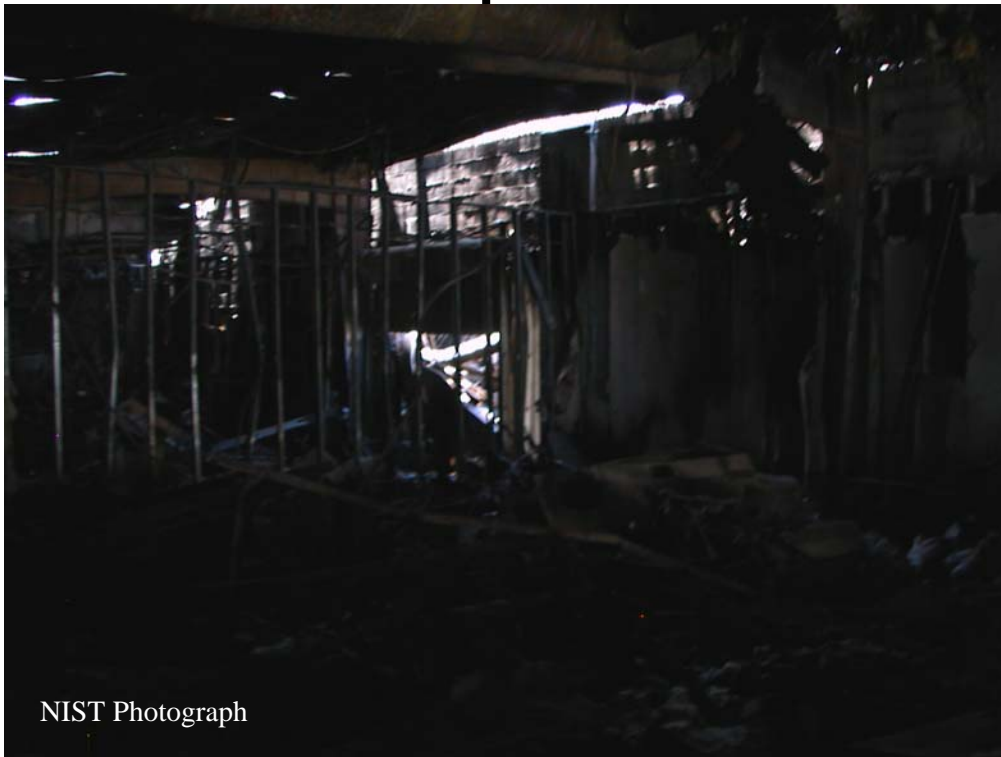
Figure F-16. Interior view of east showroom looking toward partially closed roll-down fire door. Metal studs of rear partition wall visible in left-center background of photo.
