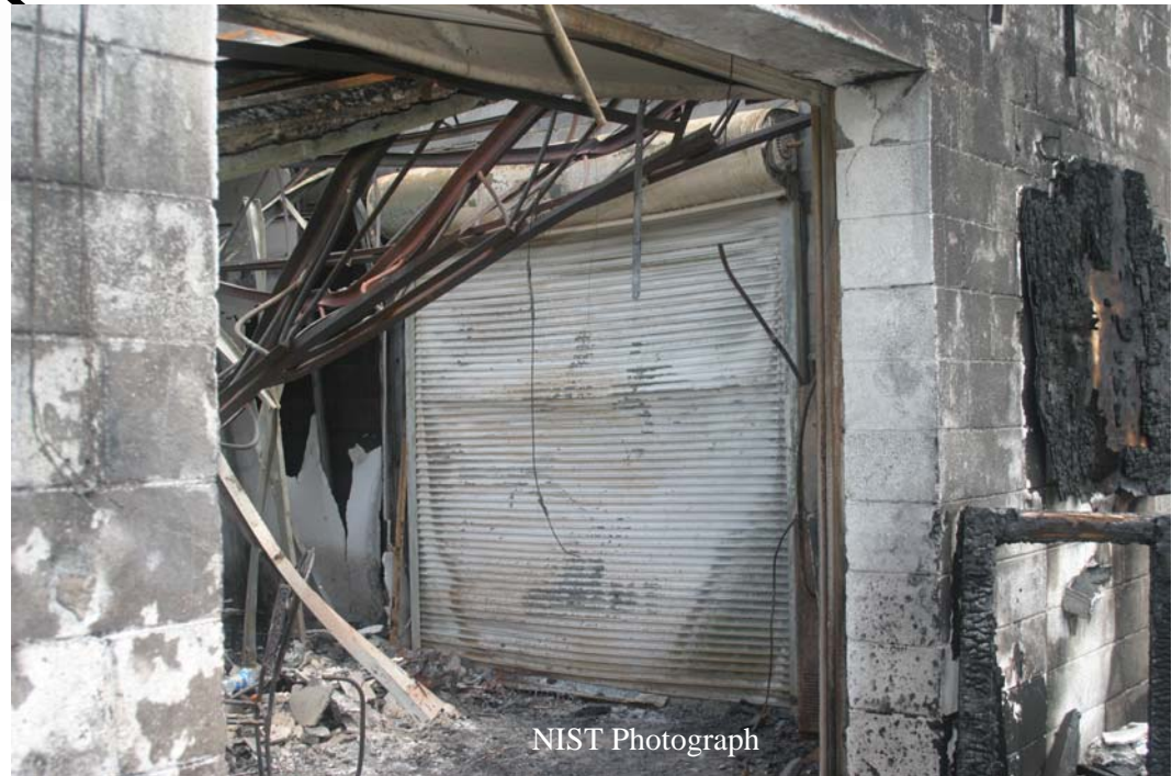
Figure O-7. Breezeway roll-down fire door looking from loading dock area through loading dock non-fire roll-down door. Fire door identified as roll-down fire door #1 in Figure O-1.
