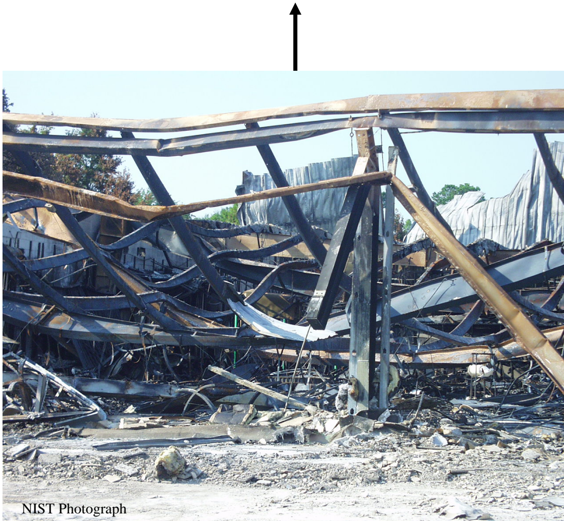
Figure E-12. Exterior view of west showroom looking into enter-front portion of showroom. Roof Z-channel and I-beam supports sagged to within 1m (3.3 ft) of showroom floor.
