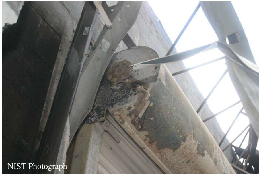
Figure O-9. East side of breezeway roll-down fire door mechanism.
