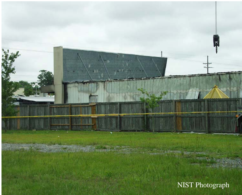
Figure E-5. Rear of front wall of west showroom. Metal sided west wall of showroom also visible in center of photo. Wooden fence separates furniture store from an adjacent property.
