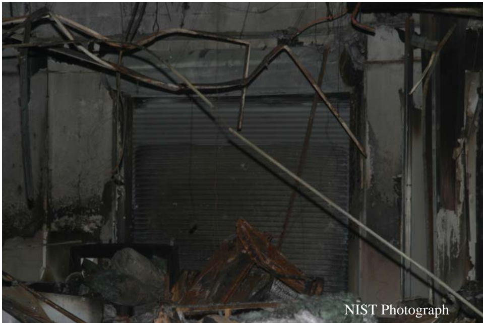
Figure O-40. Main showroom roll-down fire door looking toward middle of main showroom. Door identified as roll-down fire door #6 in Figure O-1.
