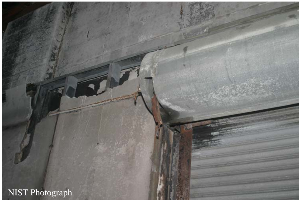
Figure O-44. South side of operating mechanism for roll-down fire door #6. Portion of fusible link visible in center of photo.
