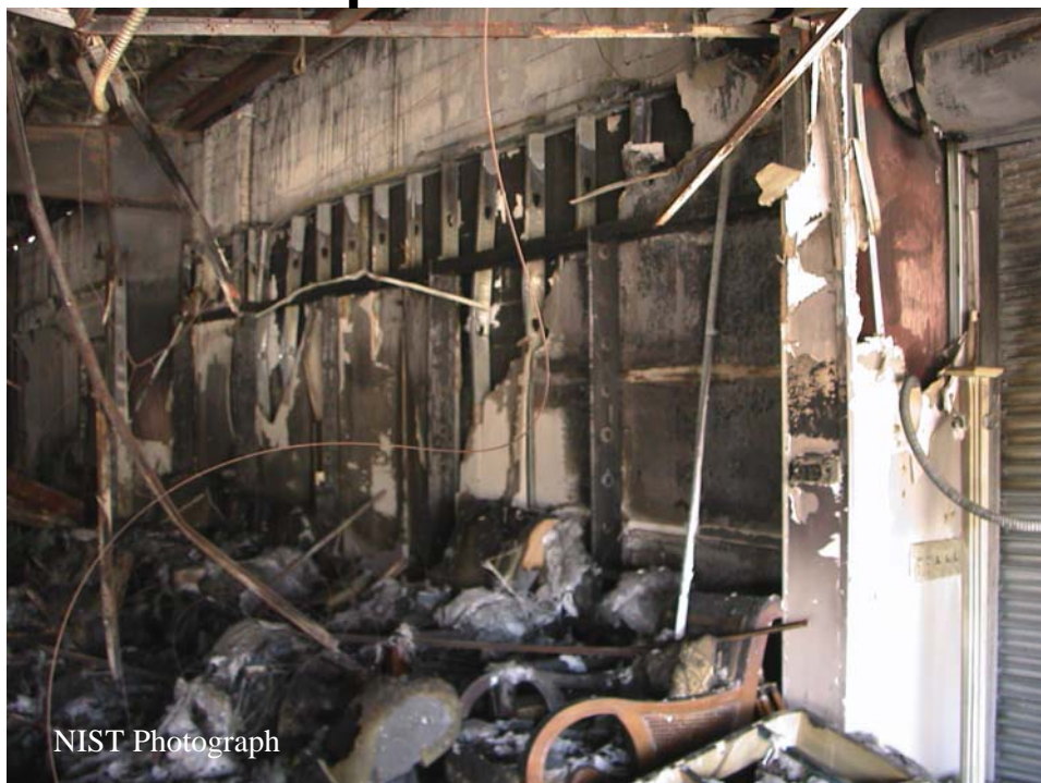
Figure F-19. Interior of east showroom. Closed roll-down fire door visible on right of image.
