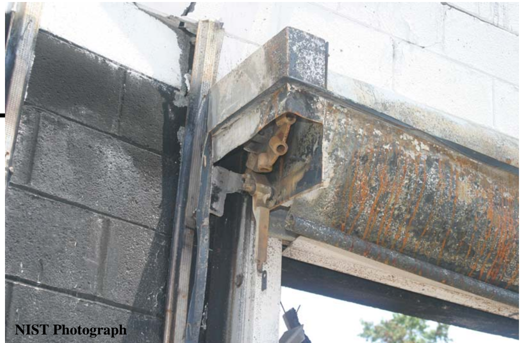
Figure O-19. North side of operating mechanism for roll-down fire door #4. Portion of fusible link visible in center-bottom of photo.
