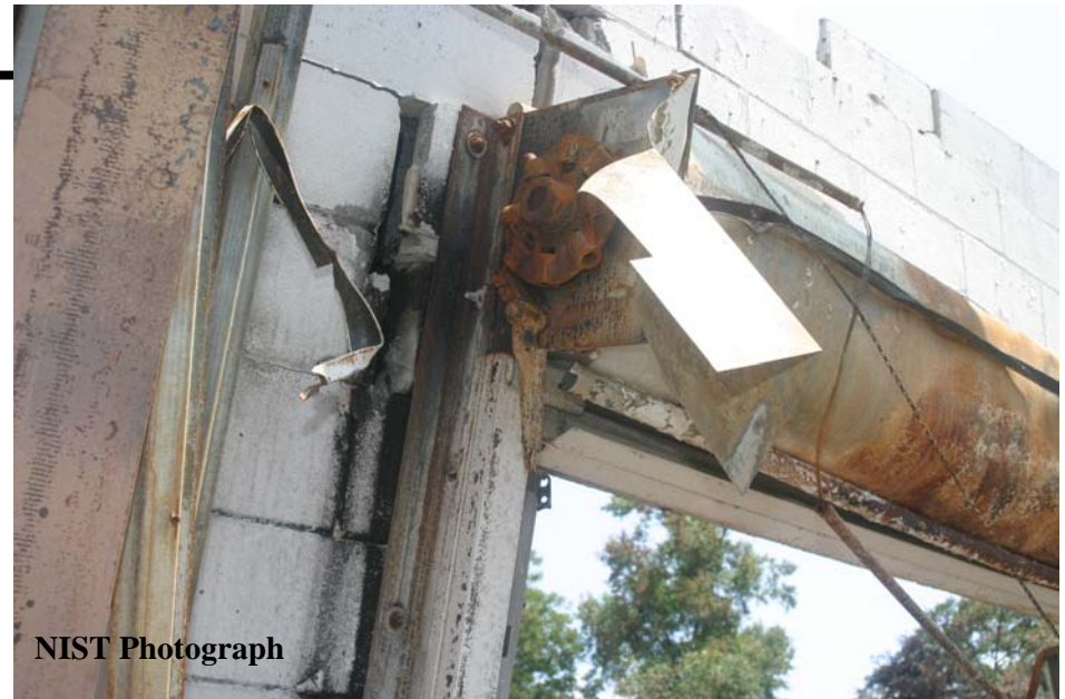
Figure O-26. North side of operating mechanism for roll-down fire door #3. Portion of fusible link visible in center of photo.
