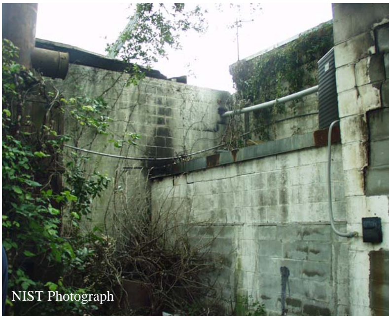
Figure I-11. Openings on the rear wall of main showroom that were filled in with concrete blocks. Incinerator exhaust stack visible in left of photograph.
