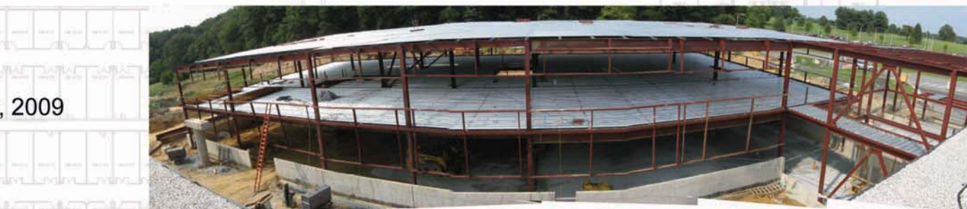
Panoramic view of Technical Support Building construction
