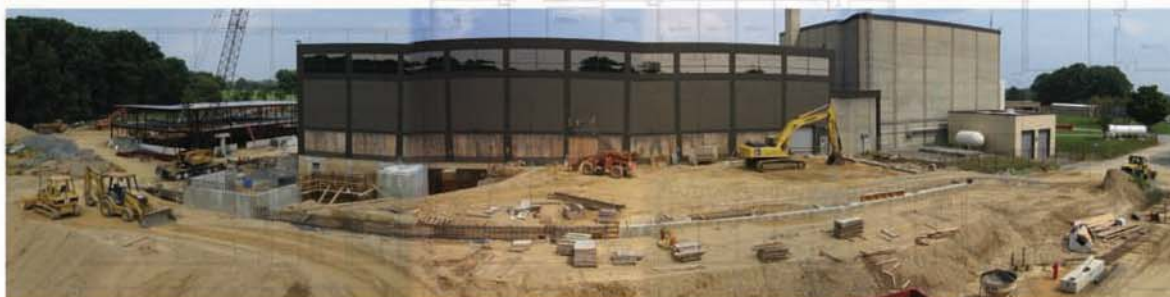
Panoramic view of New Guide Hall construction
