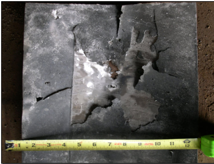
Figure 9–26. Post-Test Damage Image of EPP-05 Enhanced Powder Panel.
