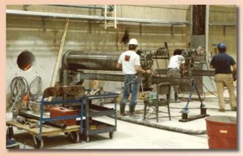
Prílling through 20' concrete wall to bring neutron guides from the source, 1989.
