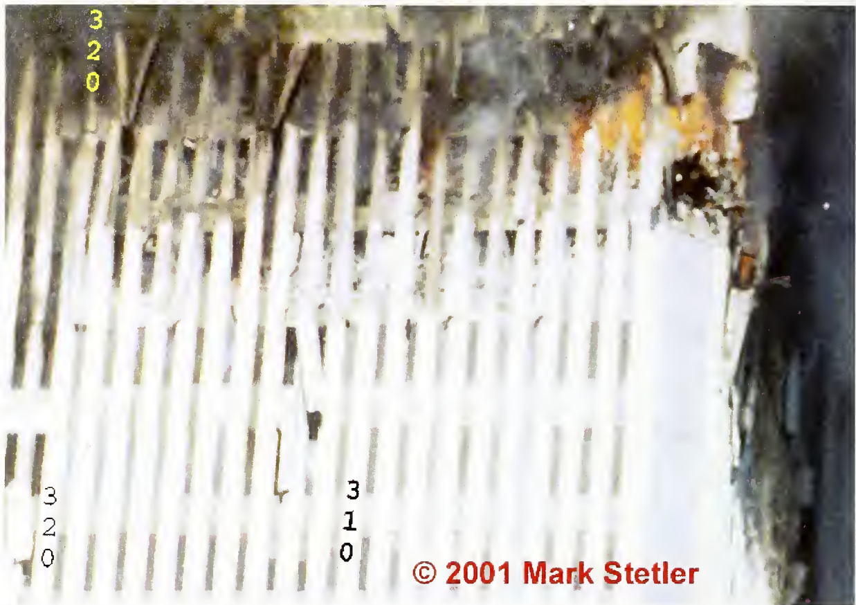
Figure H-7. This photograph is cropped from the image shown in Figure H-6. It was taken on September 11 and shows the east face of WTC 2 at the northeast corner from floor 77 to floor 82. Note the large piles of debris evident on floor 80 and floor 81.
