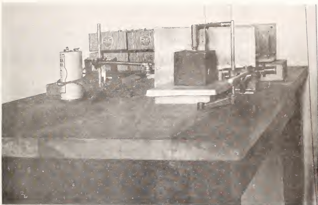
Photo No. 7. Gold-leaf electroscope (in black shield) and Duane-type ionization chamber (in background). The x-ray source is in lead-lined room behind chamber (1933).
