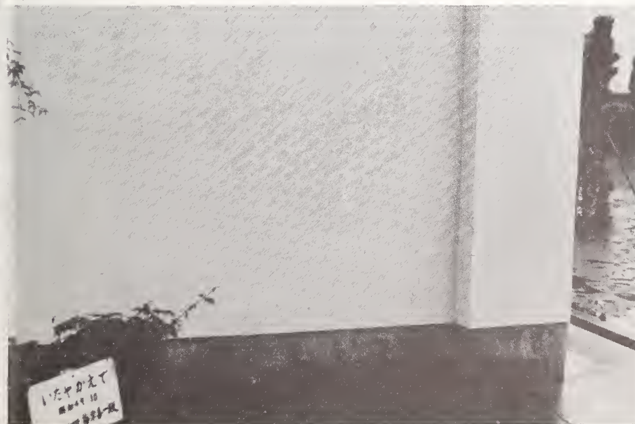
Figure 6.61 Izumi High School. The diagonal crack in the exterior wall shows that foundation settlement or uplift took place at the corner.
