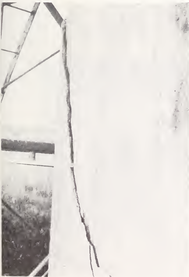
Figure 7.15 Yuriage Bridge. The face of Pier 1 showing severe distress. The plaster of paris patchwork is used to determine if additional pier cracking has occurred.
