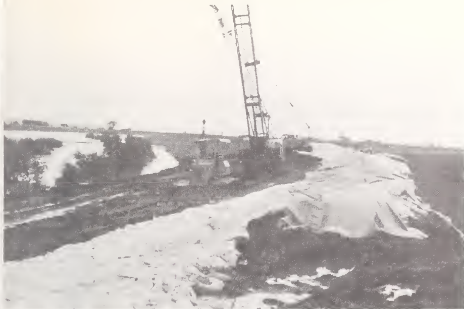
Figure 8.10 Site 3, Yoshida River. View east (downstream) along section of dike where repairs are underway. Dike crest settled as much as 1 m over a length of 5 km. Sand bags have been placed as part of repair process.
