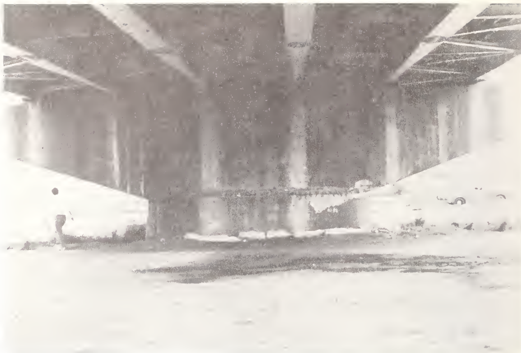
Figure 7.21 Sendai Ohashi Bridge. Typical pier configuration. The cross pier dimensions are approximately 5 m x 2 m. Note the massive pier caps. (Courtesy J.M.O.C.)
