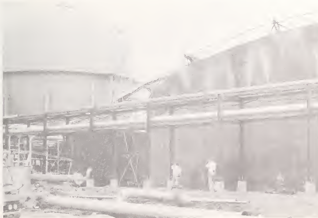
Figure 6.32 Haranomachi Plant, Sendai City Gas Bureau: The newly erected pipeway, with the collapsed holder in the background. Note the undamaged pressurized propane gas sphere in the back.
