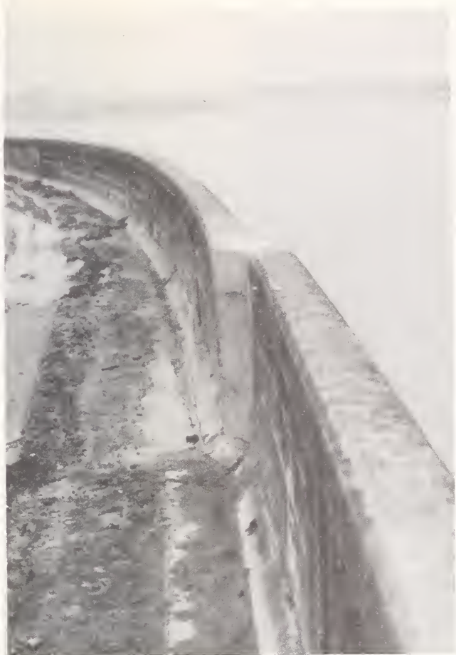
Figure 8.6 Site 2, Natori River. View is west along repaired portion of dike. Note patch across offset in retaining wall offset caused by lateral spreading during earthquake. Retaining wall rises approximately 1 m above roadway.
