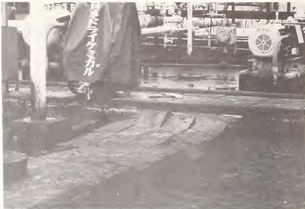
Figure 6.48 Sendai Refinery, Tohoku Oil Company, Ltd.: ground settlement at the refinery.
