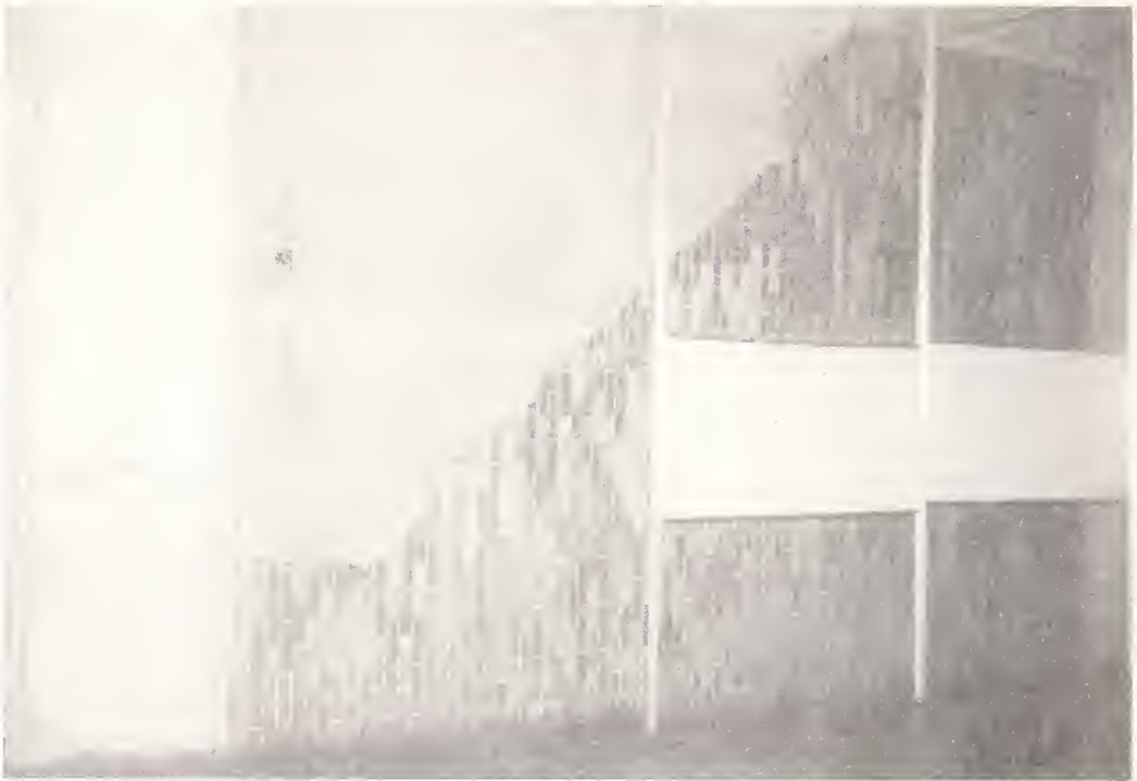
Figure 5.80 Tohoku University Engineering Building. Damage to glazed tile veneer of shear wall at ground level.
