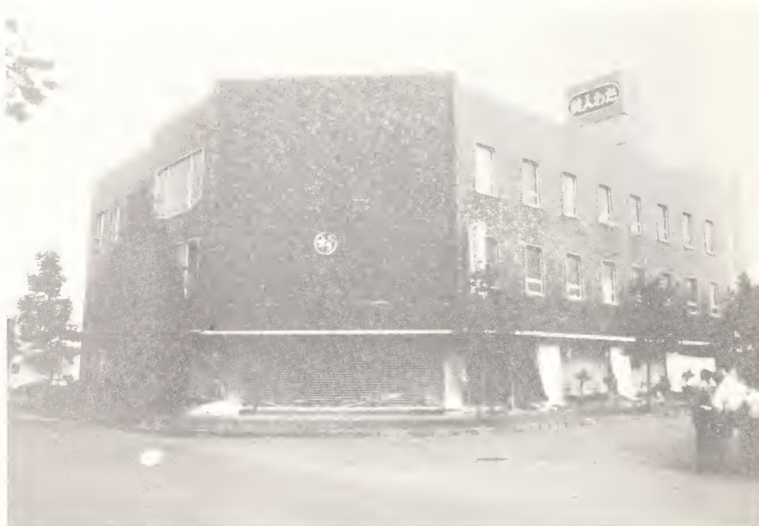
Figure 5.33 Kinoshita Building. The brick facing on the west side of the structure showed little sign of damage.
