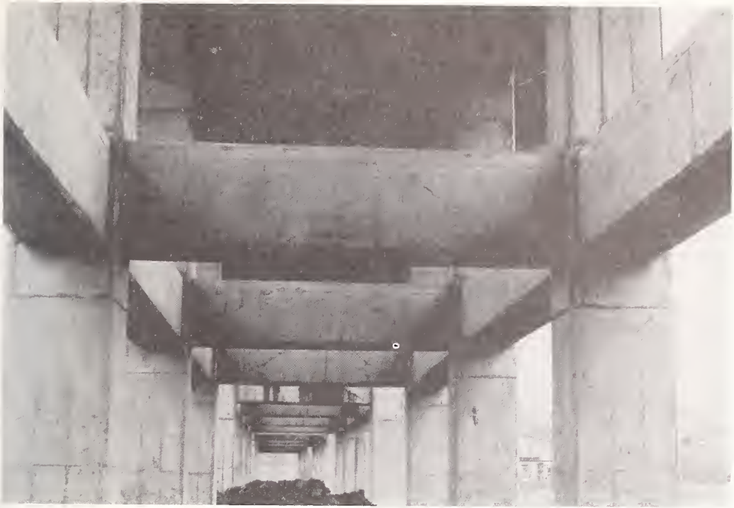
Figure 7.53 Tensile cracking of space frame tie beams near the Rifu Construction Office.
