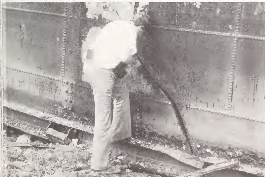
Figure 6.36 Haranomachi Plant, Sendai City Gas Bureau: a fracture of the 3/8-in. plate wall of the collapsed gas holder. The length of the fracture is approximately 1.5 m (5 ft).
