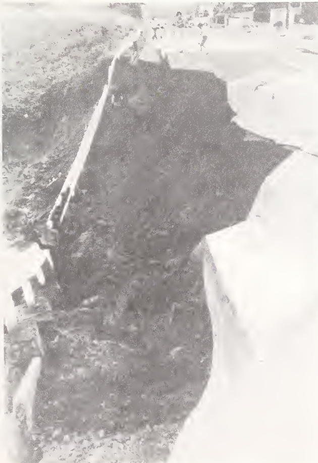
Figure 7.44 Typical Road Fill Failure.
