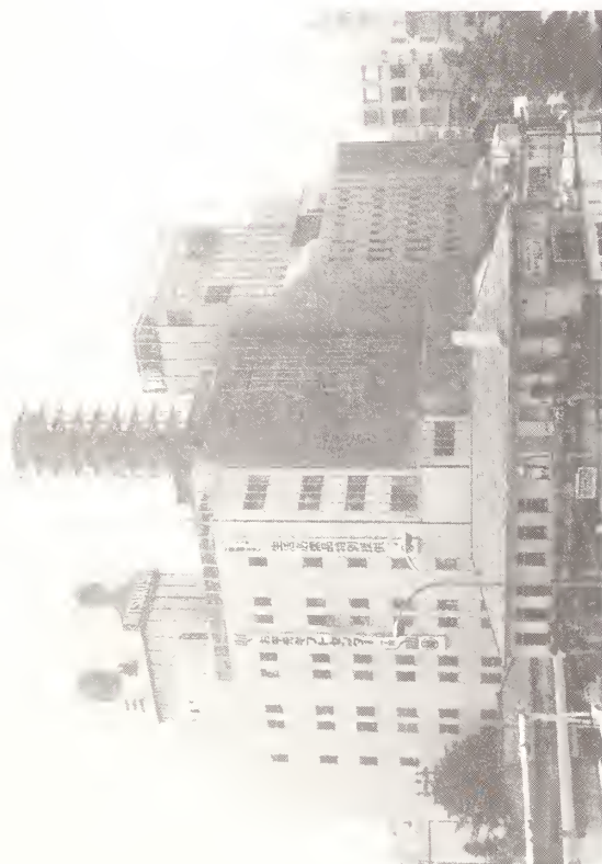
Figure 5.8 Chimney damage to the Mitsukoshi Department store. Numerous such chimneys suffered such damage.
