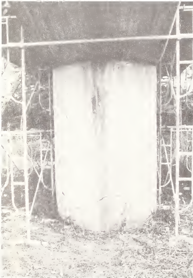
Figure 7.13 Yuriage Bridge. Evidence of light girder impacting with the abutment and pronounced shear cracking of exterior girder at the bearing.
