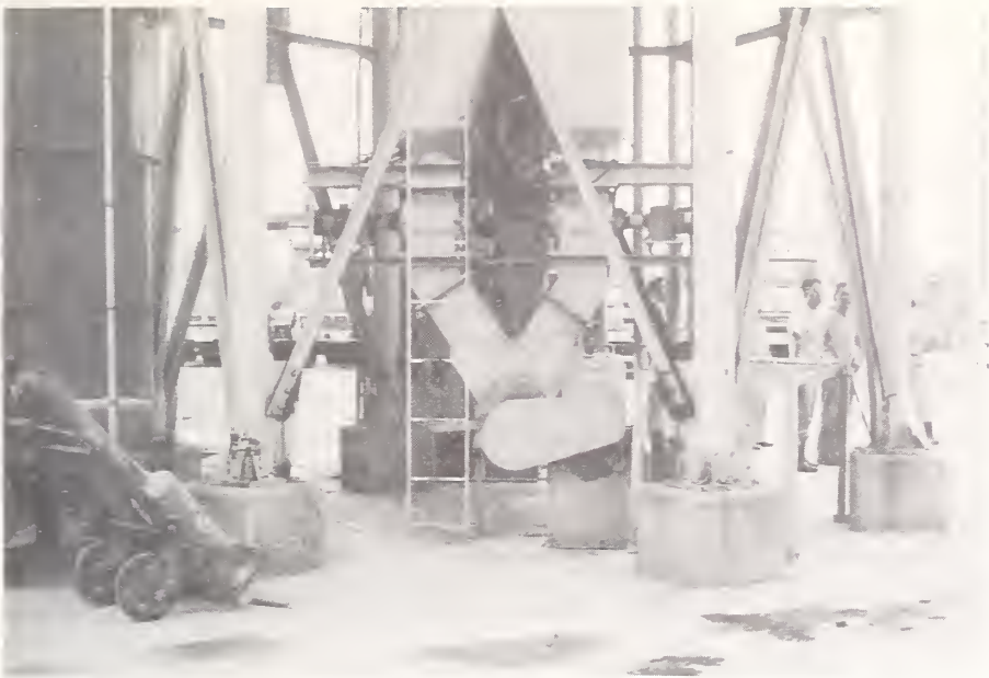
Figure 6.50 Concrete Batch Plant, Sendai: view of the repaired supporting substructure of a cement bin and related equipment. The sheared bolts at the brace connections have been removed and the braces have been welded to the gusset plates. Some of the buckled braces have been replaced entirely.
