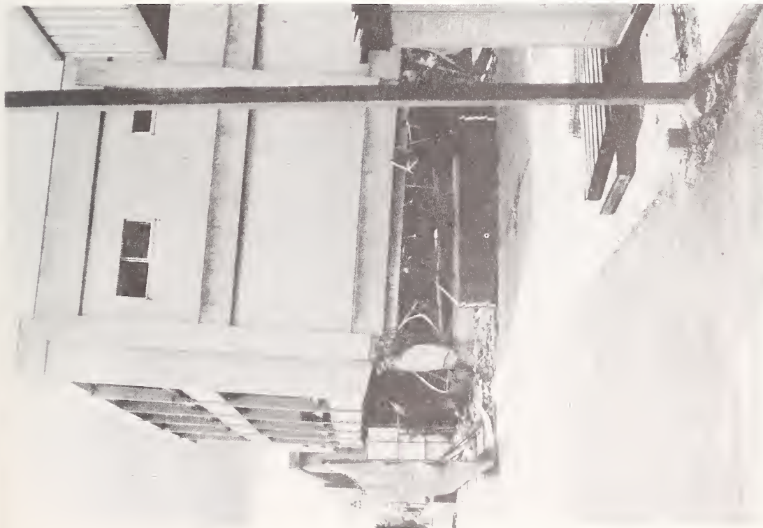
Figure 5.24 Maruyoshi Building, view from the east. Failure of first story columns occurred in shear.
