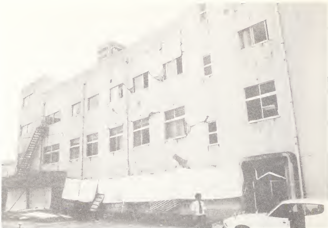
Figure 5.32 Kinoshita Building, Oroshicho area, of Sendai. Extensive diagonal cracking was observed on the east face (rear) of the building.
