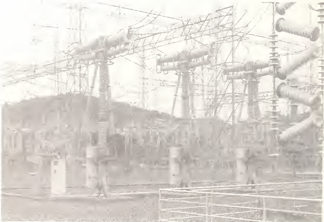
Figure 6.22 Sendai Substation, Izumi: three replaced 3-phase circuit breakers. This type of T-shaped circuit breaker suffered a high percentage of damage. Often the three symmetrical guides broke before the main stem. In all cases the structural steel supports appeared to be undamaged.
