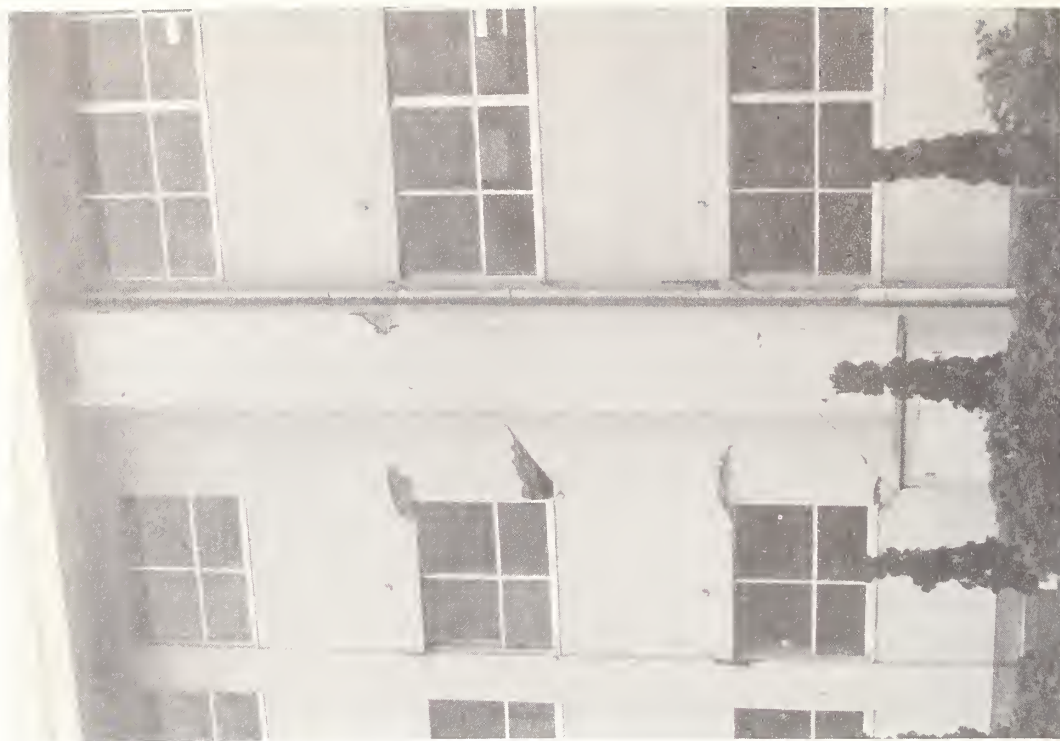
Figure 5.63 Izumi High School, typical classroom building, north face. All faces with the larger infill panels were similarly damaged.
