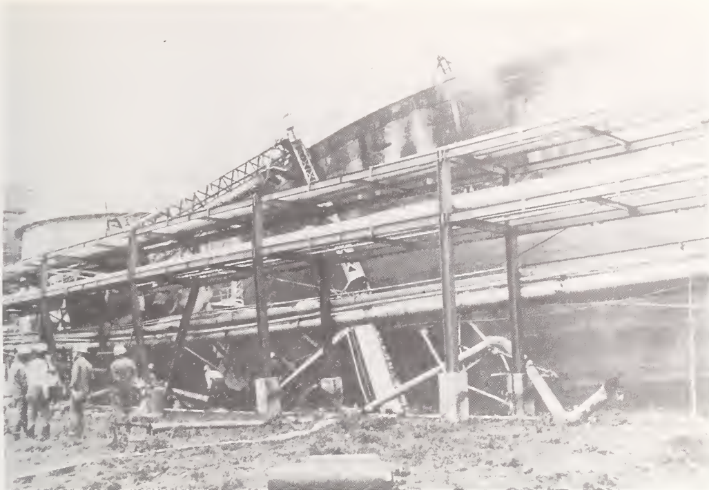
Figure 6.31 Haranomachi Plant, Sendai Gas Bureau; collapsed gas holder and the damaged adjacent pipeway structure just after the earthquake, (Sendai Gas Bureau Photograph)
