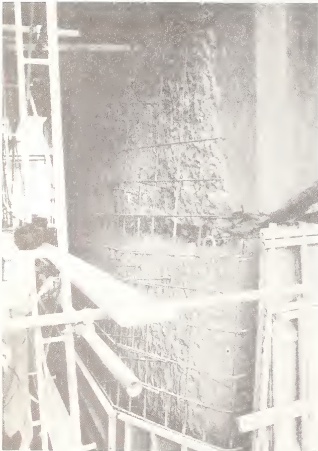
Figure 7.25 Sendai Ohashi Bridge. Typical damage being repaired at the base of the pier. Note the outward buckling of the underformed vertical rebar. The concrete cover had been roughened, the footing strengthened, and additional rebar placed to strengthen the pier.
