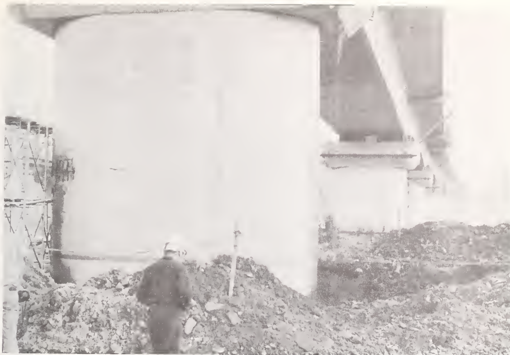
Figure 7.49 The Natori River Bridge is a three-span continuous single cell reinforced cast-in-place concrete box girder structure on 3 m x 6 m piers approximately 8 meters above grade. Typical damage included cracking in the central part of the pier where the gross cross-sectional area of vertical steel was reduced.
