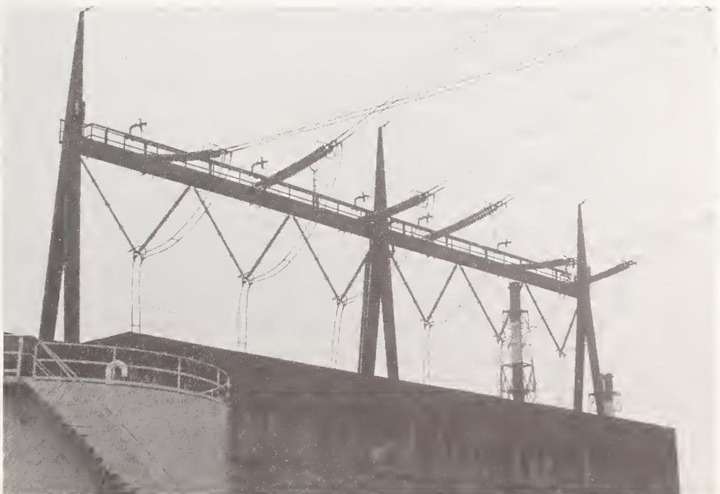
Figure 6.10 Fukushima Nuclear Power Plant. Broken ceramic insulators were the only damage reported for the site. The damaged insulators had been replaced, as illustrated above, within hours after the earthquake and before the reconnaissance visit.
