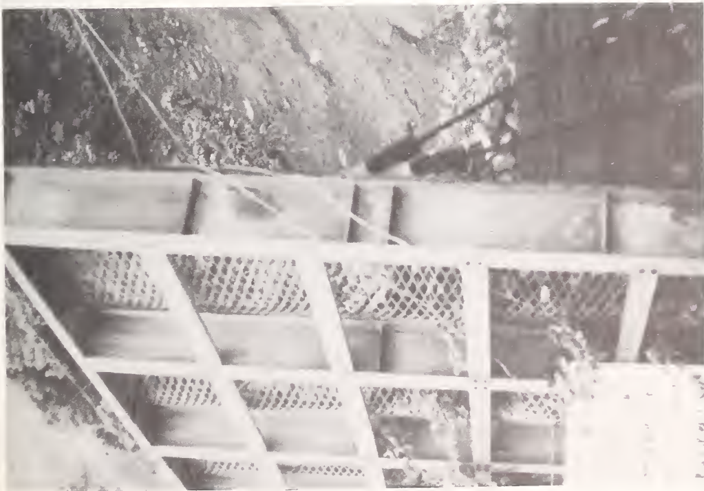
Figure 7.47 Steel bins constructed to contain rockslides along highways.
