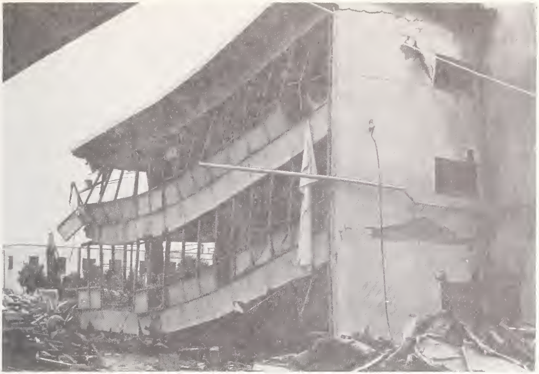
Figure 5.52 Taiyo Fisheries Plant, viewed from the northeast. The reinforced concrete shear wall on the north end was badly damaged.
