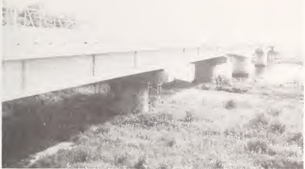
Figure 7.11 General view of the Yuriage Bridge showing the first two columns which were heavily damaged.
