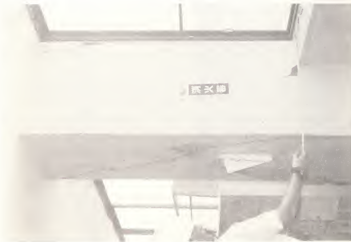
Figure 5.67 Tohoku Institute of Technology. Typical damage to seventh story column of the north facade of building 5.
