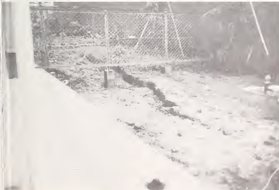
Figure 5.83 Sunny Heights Apartment Building. Ground cracking and settlement adjacent to walkway surrounding the building.
