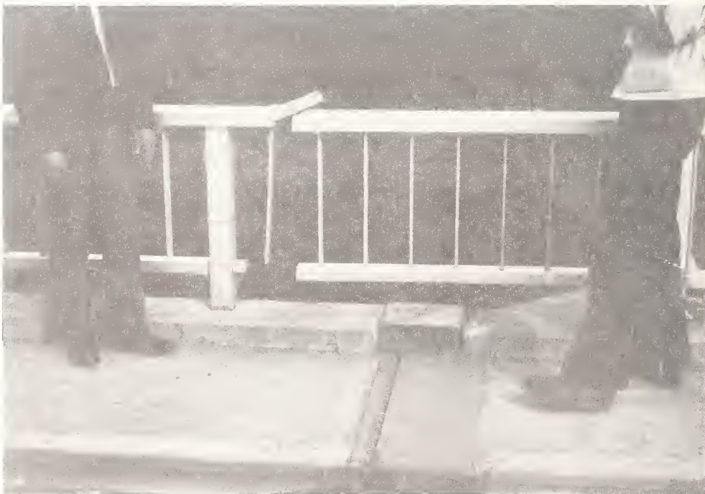
Figure 7.18 Yuriage Bridge. Evidence of 8 cm of longitudinal movement as shown at the handrail expansion joint, Pier 2. However, there was no evidence of damage to the girders or the second pier.
