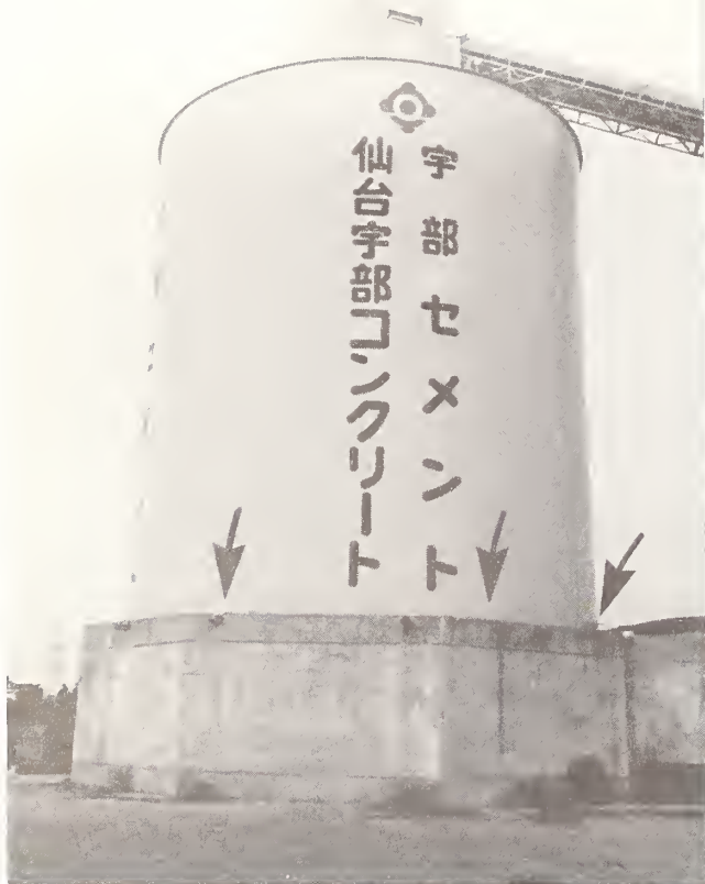
Figure 6.53 Concrete Batch Plant, Sendai: a detailed view of the damaged base of the sand and gravel storage tank. Note the closely spaced anchor bolts. Similar damage occurred at several locations along the circumference.
