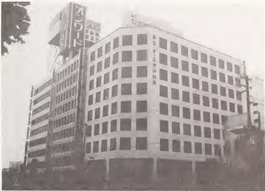
Figure 5.6 Second Eastern Building Company Building, Sendai. A typical modern building in Sendai; the only apparant damage to the glazed tile veneer on the exterior was cracking on spandrels and shear walls.
