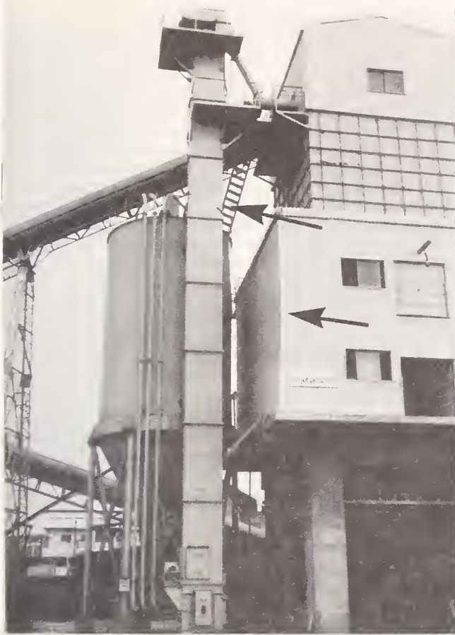
Figure 6.54 Concrete Batch Plant, Sendai: displacement due to damage to the light, unbraced steel superstructure damaged the vertical stack and the conveyor belt structure.
