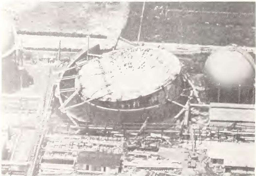
Figure 6.30 Haranomachi Plant, Sendai City Gas Bureau: an overall view of a collapsed propane gas holder and some of the surrounding propane storage tanks and affected pipeway and equipment. (Kahoku Newspaper Co. photograph)
