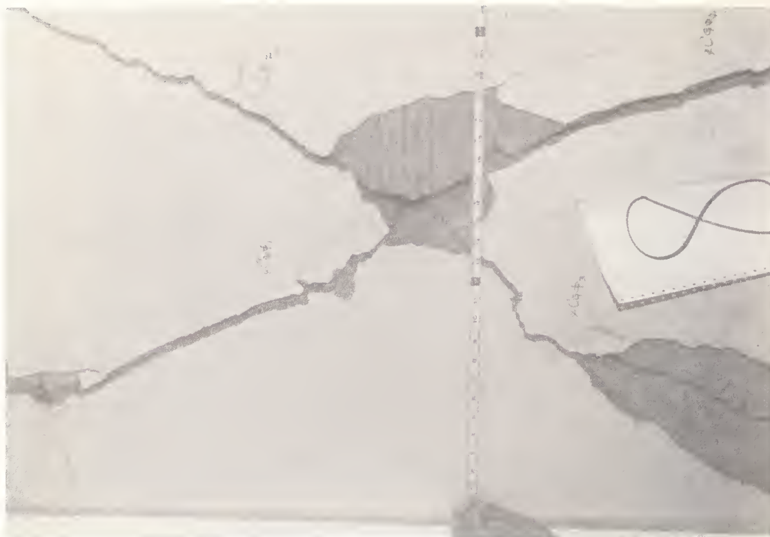
Figure 5.68 Tohoku Institute of Technology, Building 5. Detail of column damage.
