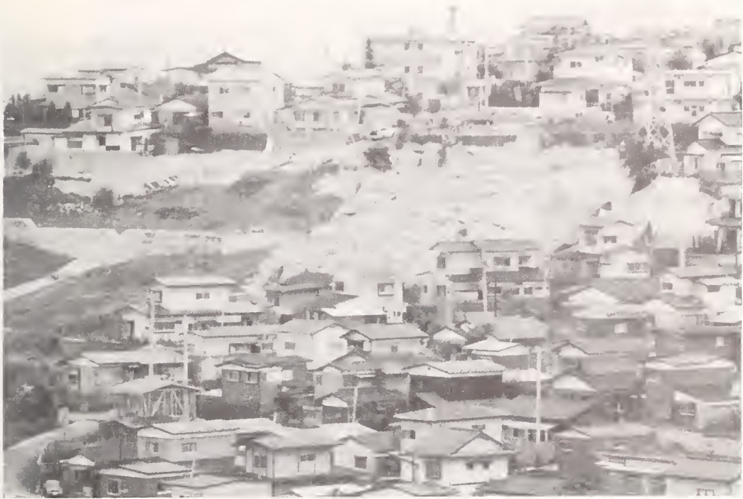
Figure 9.17 Rotational slump in artificial fill in Sendai (area covered by tarps) which destroyed one house and is threatening others. To left of slump is concrete slope protection dam (sabo works).
