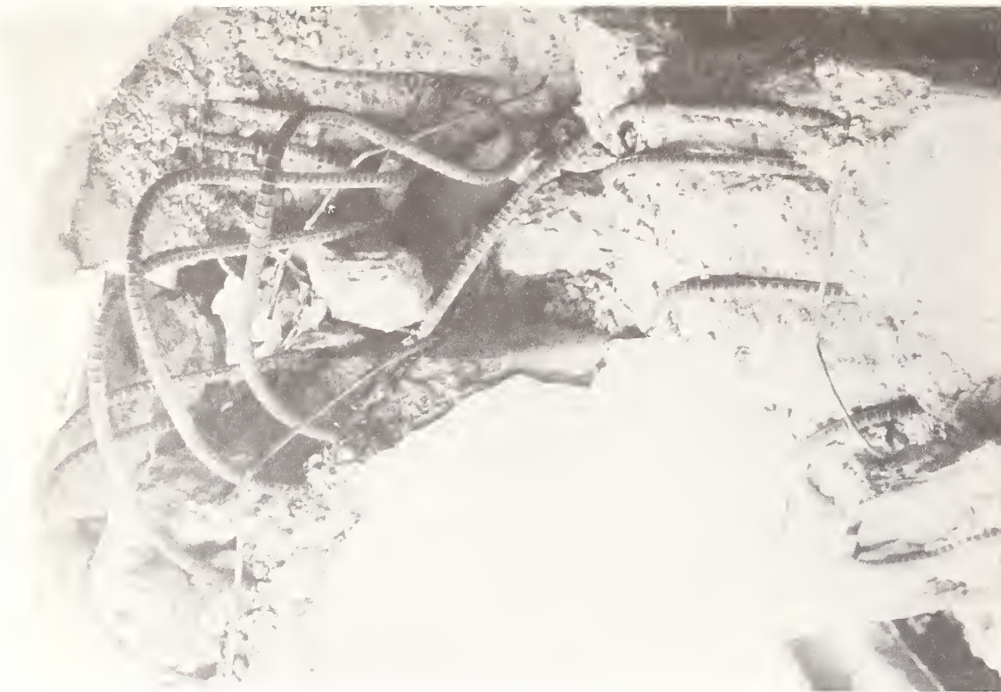
Figure 5.43 Yazaki Industries Buildings. Detail of column shear failure, east side. Note use of deformed bars.
