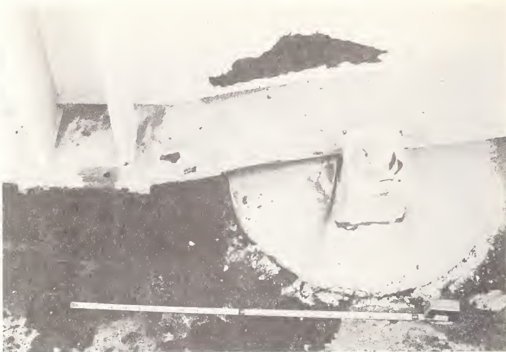
Figure 7.5 Kin-noh Bridge. The girders at Pier 8 displaced longitudinally toward the abutment 55 cm allowing the unrestrained suspended span to drop off the 45 cm hinge seat. The movable girder bearing plate came to rest at the edge of the pier cap. The fixed bearing on Pier 7, the opposite side of the suspended span, displaced longitudinally 0.5 cm.
