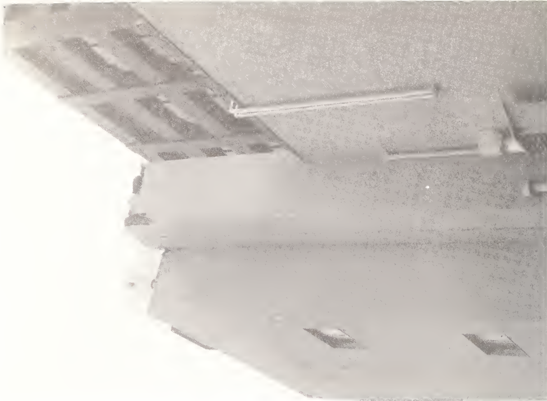
Figure 5.8 Chimney damage to the Mitsukoshi Department store. Numerous such chimneys suffered such damage.
