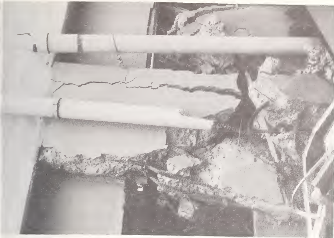
Figure 5.41 Yazaki Industries, showing damage to lower story reinforced concrete column.
