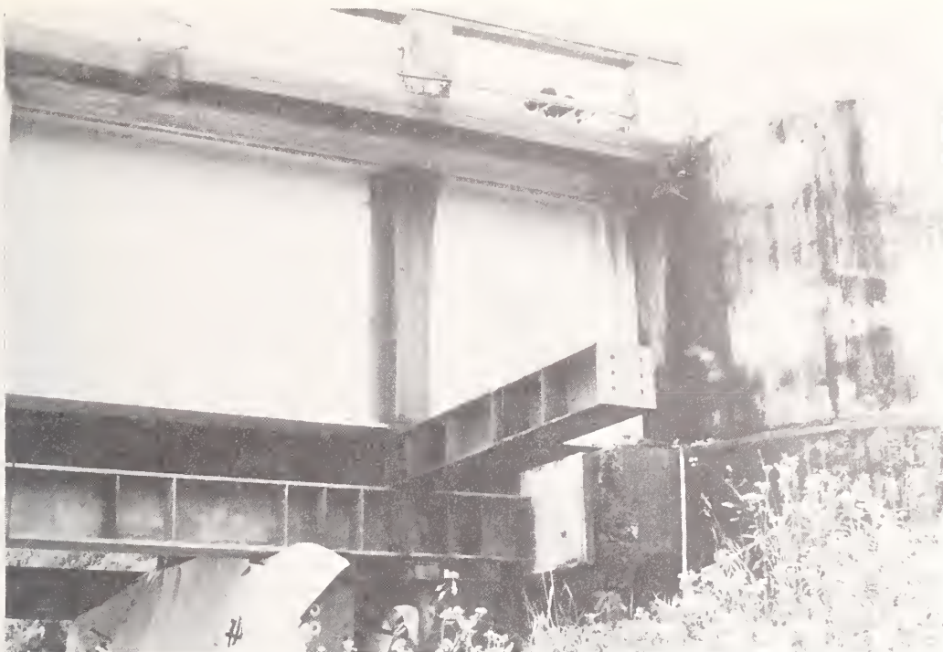
Figure 7.7 Kin-noh Bridge. Damaged abutment from the February 20, 1978, 6.7 magnitude earthquake. New web stiffener at point of temporary shoring.
