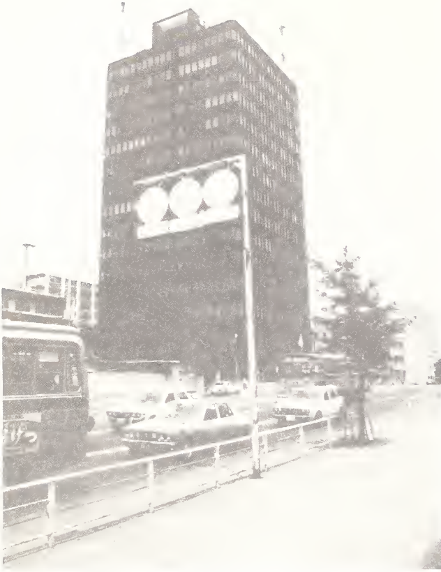
Figure 5.13 Sendai Second Government Building. This modern steel frame structure suffered no damage.
