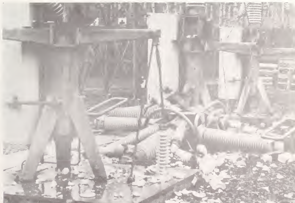
Figure 6.24 Sendai Substation, Izumi: another three failed 3-phase, T-shaped circuit breakers. Note the failed main stems, the loose guide wires and the undamaged steel supports which are attached to their foundations. (Tohoku Electric Power Co. photograph)
