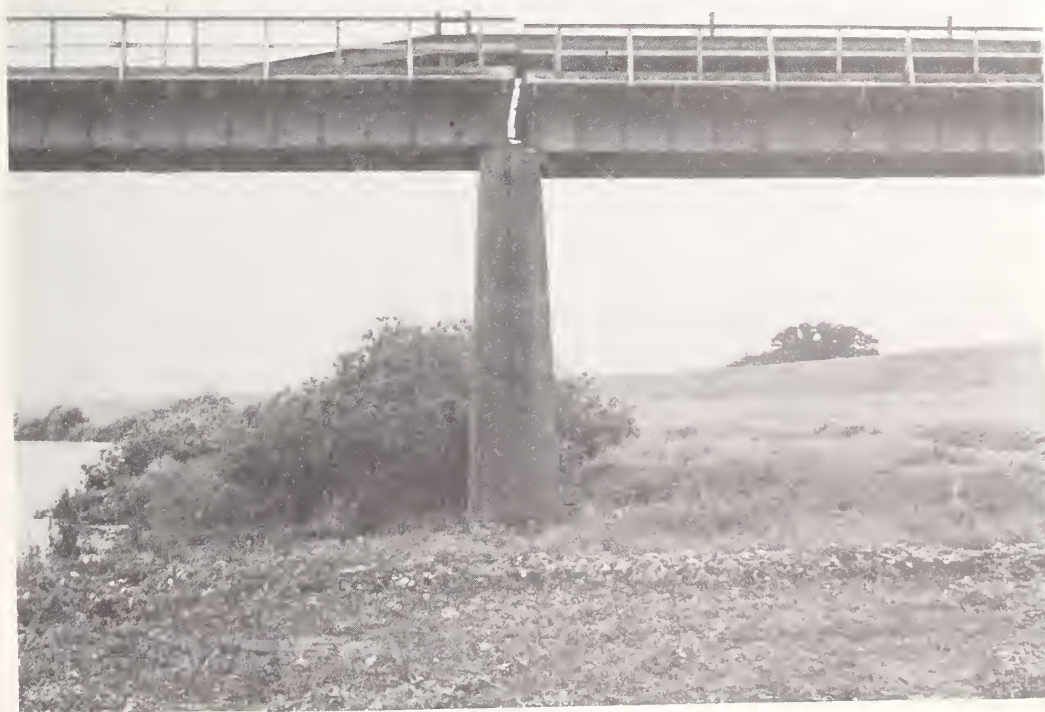
Figure 7.38 Longitudinal displacement of superstructure. Note the temporary structure which spans the dislodged main span.
