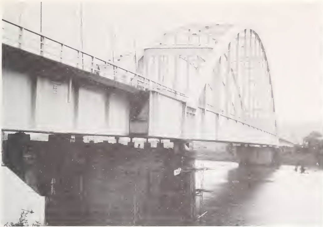
Figure 7.33 The main tied arch span of the Tenno Bridge with the cracked wall pier in the foreground. Note the smaller, pedestrian bridge in the background.
