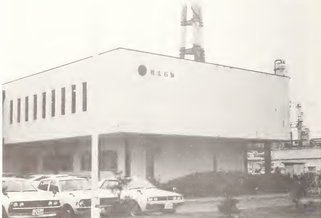
Figure 6.49 Sendai Refinery, Tohoku Oil Company, Ltd.: A wing of the damaged steel-framed administration building. Damage was obvious only to the architectural finishes.
