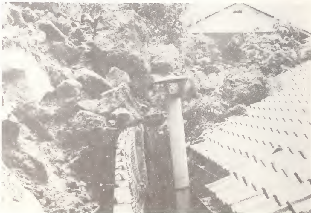
Figure 9.11 Rock fall damage to retaining wall and roof of house in left-hand portion (arrow) of figure 9.10. (Photograph courtesy of Y. Tsuruya)
