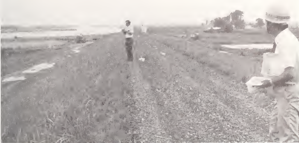
Figure 8.2 Site 1, Natori River, view downstream (southeast) along repaired portion of dike. Dike is made of compacted sand. It rises 2 m above the high water level of the river and has side slopes of 2H:1V. Natori River in center-left background.
