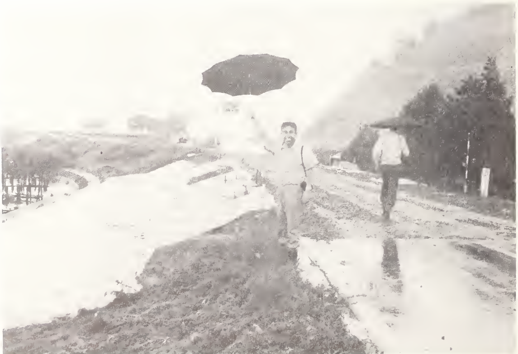
Figure 7.36 Road damage and temporary stabilization of the Kitakami Dike near the bridge site.
