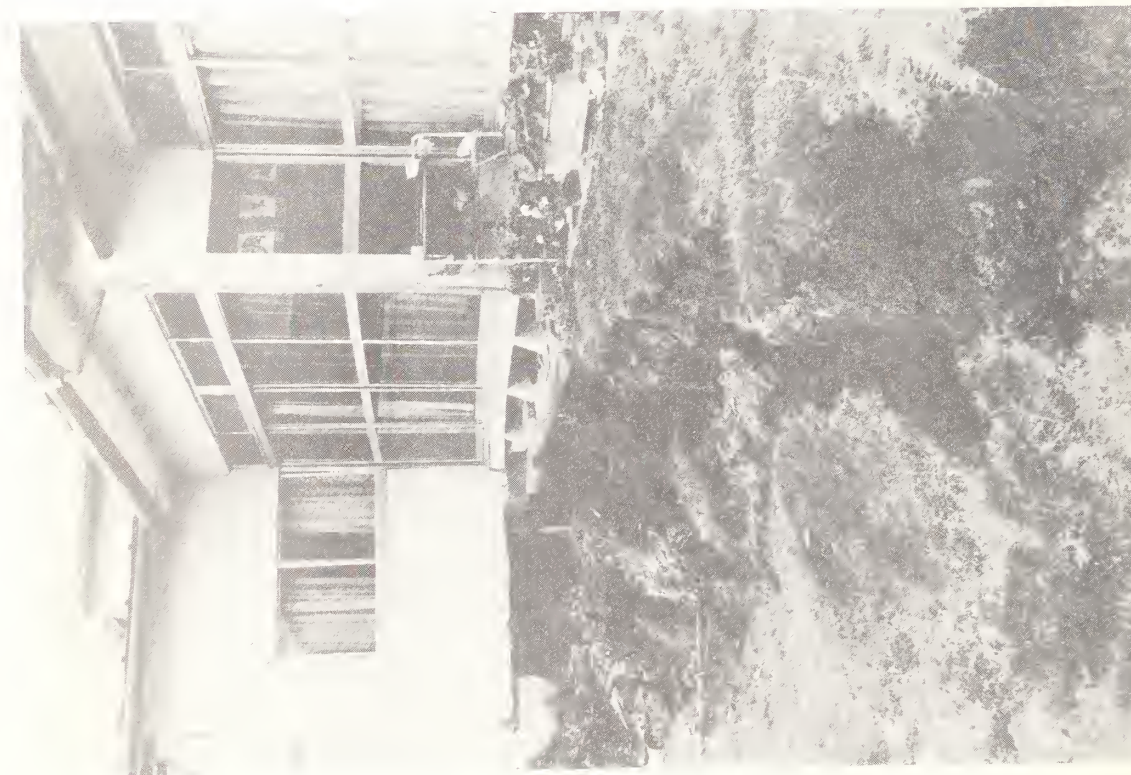
Figure 5.84 Sendai. Damage to single family residence due to loss of foundation support. (Japan National Land Agency photograph)
