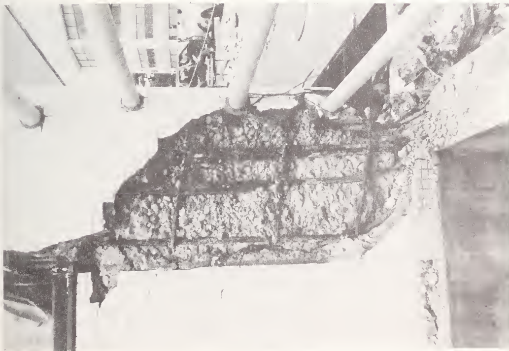
Figure 5.77 Tohoku Institute of Technology, Building 3. Detail of one of the damaged columns of the exterior frame on the south side of the building showing reinforcing details.
