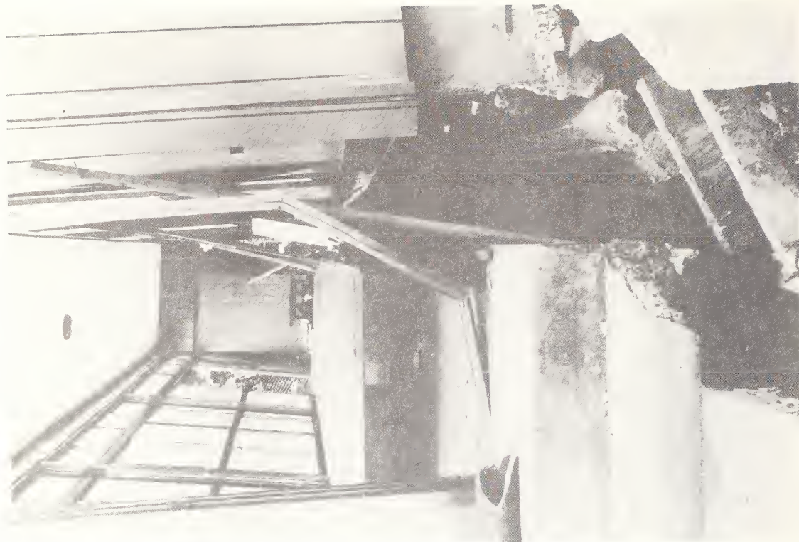
Figure 5.85 Sendai. Damage to single family residence due to ground settlement. (Japan National Land Agency photograph)
