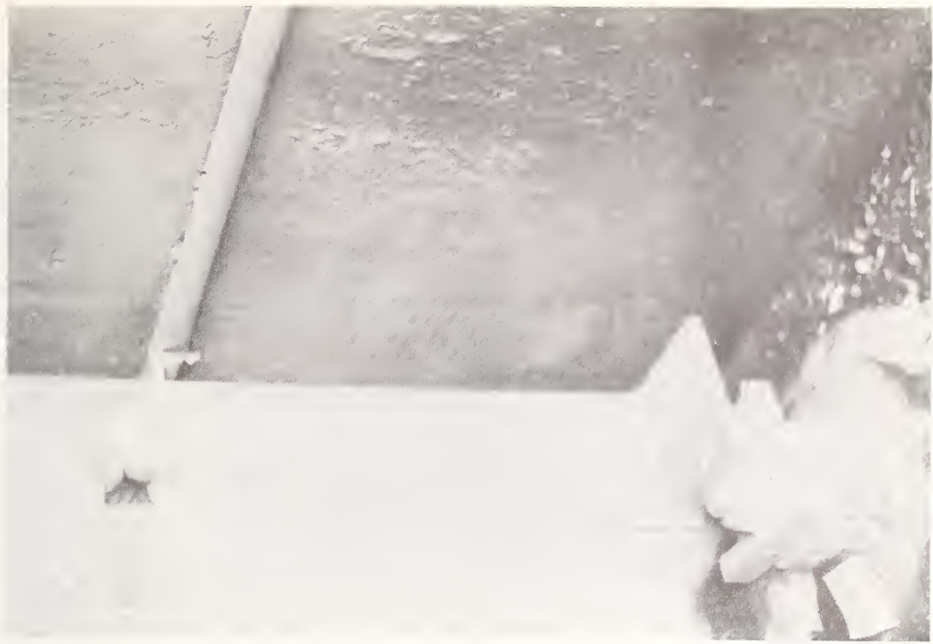
Figure 7.27 Sendai Ohashi Bridge. Abutment damage. Bearing plate broken and evidence of girder impact at abutment.
