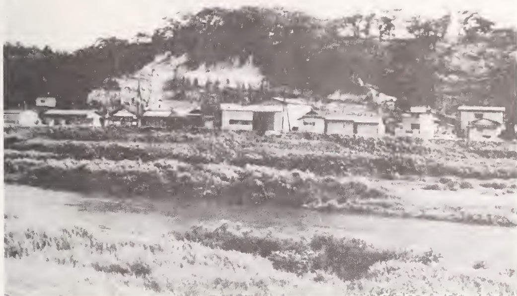
Figure 9.12 Steep slope near Hebinumayama in heavily fractured tuff which underwent failure as rock falls damaging portions of houses in front of the slope.
