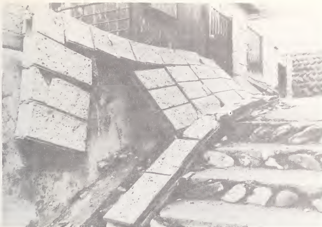
Figure 5.88 Failure of a reinforced concrete masonry privacy wall in Sendai. (Japan National Land Agency photograph)
