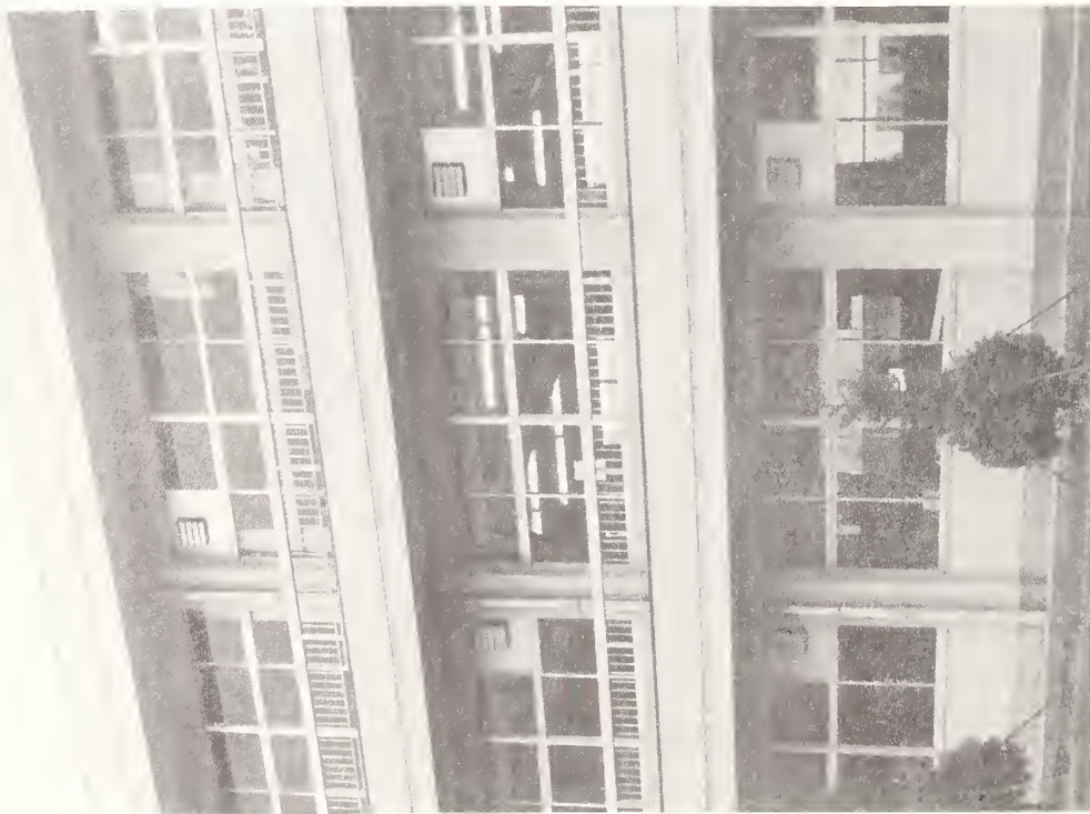
Figure 5.62 Izumi High School, typical classroom building, south face. This side of the building, which is relatively open, suffered little damage.
