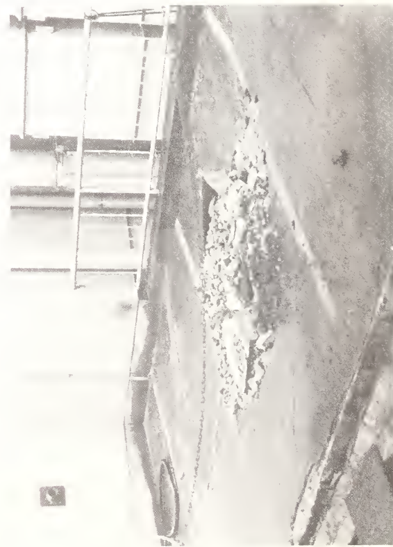
Figure 5.10 Impact area of chimney failure (see Figure 5.9)
