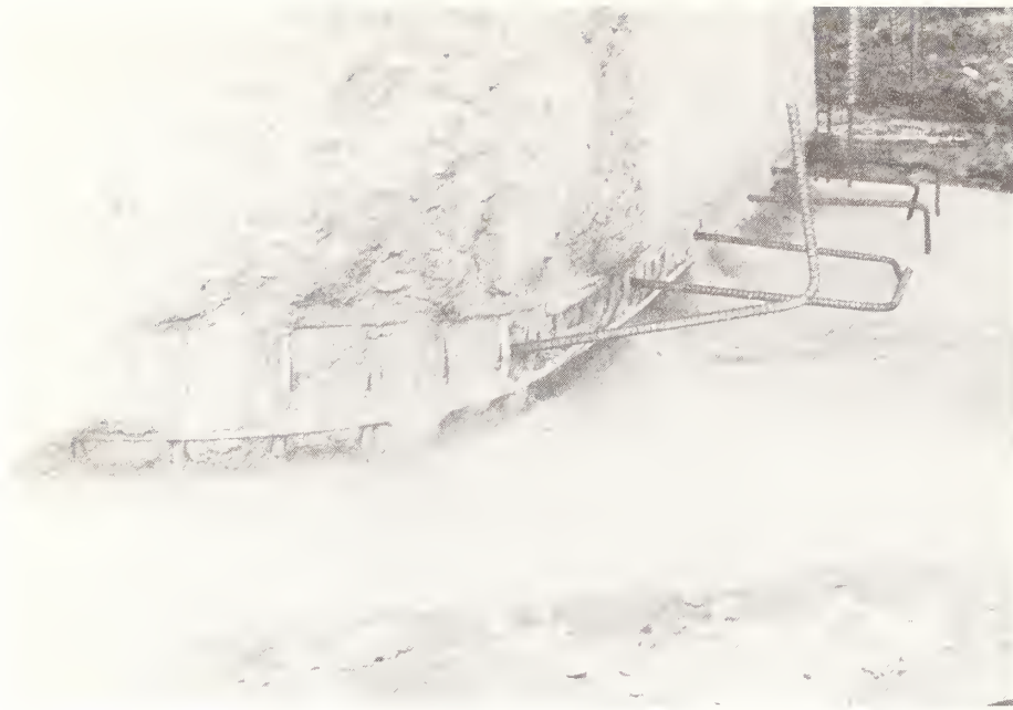
Figure 7.25 Sendai Ohashi Bridge. Typical damage being repaired at the base of the pier. Note the outward buckling of the underformed vertical rebar. The concrete cover had been roughened, the footing strengthened, and additional rebar placed to strengthen the pier.
