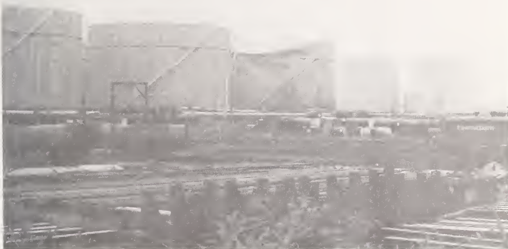
Figure 6.43 Sendai Refinery, Tohoku Oil Company, Ltd. Two other failed TC oil storage tanks.
