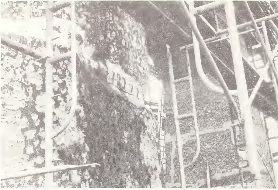
Figure 7.29 Abukuma Bridge. Outward buckling of vertical rebar at one of the damaged piers.
