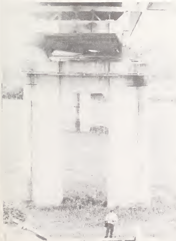
Figure 7.3 Kin-noh Bridge. View of the collapsed suspended plate girder span. Similar damage occurred to bridges in the 1971 San Fernando and 1976 Guatemala earthquakes because of lack of superstructure restraint and small bearing seats. Suspended spans are no longer used in seismically active areas. (Courtesy J.M.O.C.)
