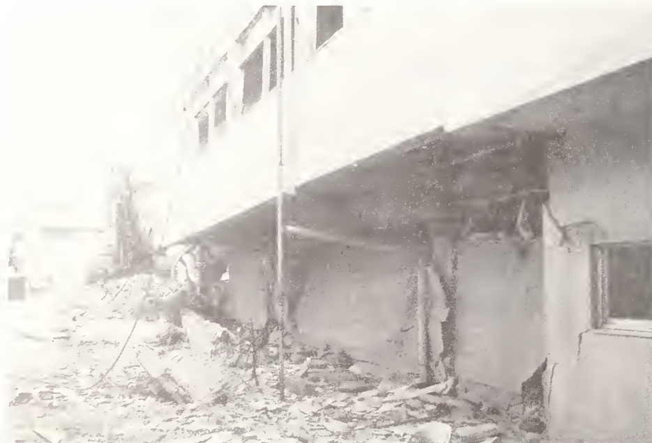
Figure 5.23 Maruyoshi Building, view from the northwest. This three story reinforced concrete frame, one span by three, suffered almost total collapse of the first floor.
