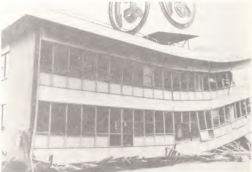
Figure 5.51 Taiyo Fisheries Plant, viewed from the west. The first story columns in the center portion of the building failed, leaving the ends of the building standing. (Japan National Land Agency photograph)
