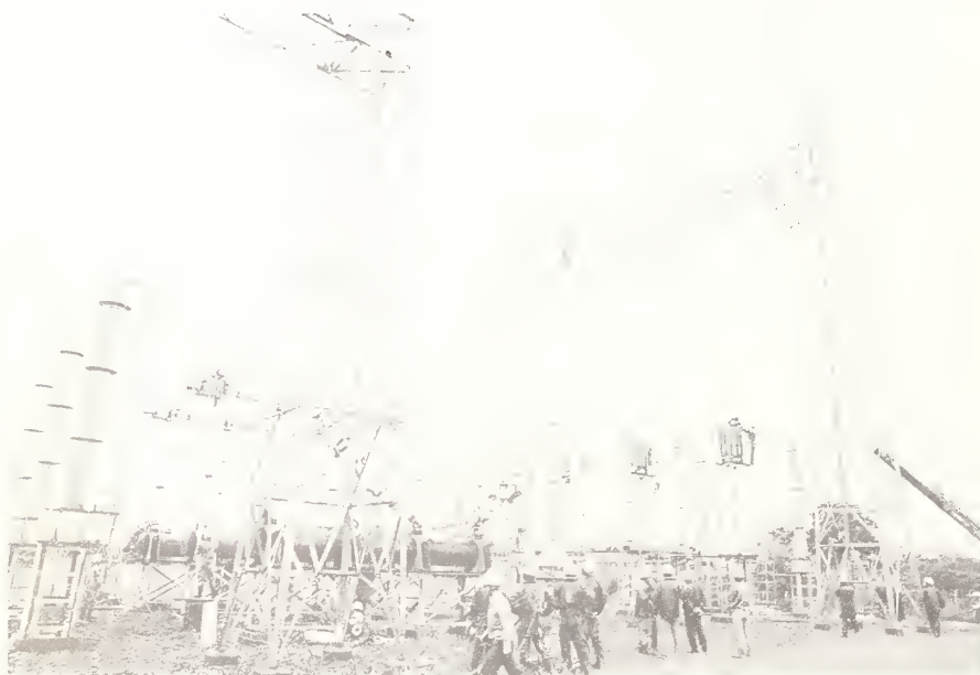
Figure 6.26 Sendai Substation, Izumi: Severe damage to circuit breakers (center of photograph - note the failed columns of live tank design, probably with gas reservoirs), current transformers (with the tapered bushings - some of the stems are also damaged), and reactors (to the left) with presumably broken connections. (Tohoku Electric Power Co. photograph)
