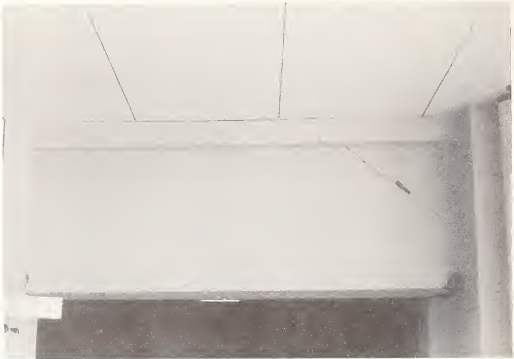
Figure 5.71 Tohoku Institute of Technology, Building 5. The tie beam over a sixth floor corridor connecting two shear walls shows diagonal cracks at both ends.
