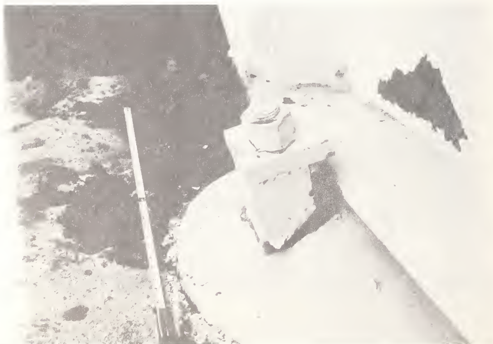
Figure 7.6 Kin-noh Bridge. Evidence of minor transverse displacement of the main girder with broken keeper. This reportedly occurred at the time of the February 20 earthquake.
