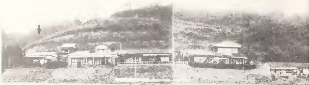
Figure 9.10 Panorama of cut slope near Kitashiona in Miocene tuff which produced rock falls during earthquake damaging nearby houses. Arrow points to damaged house shown in closer view in figure 9.11. (Photograph courtesy of Y. Tsuruya)
