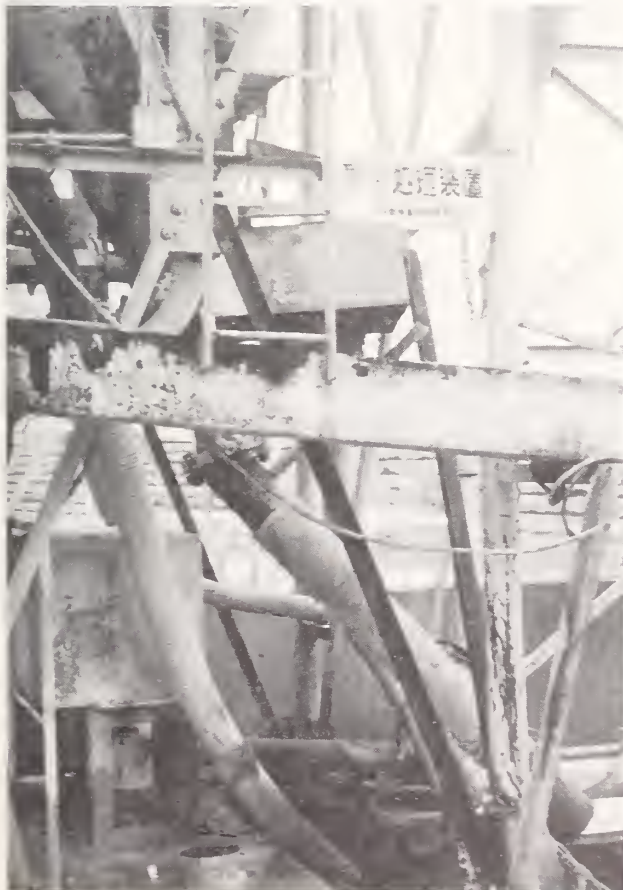
Figure 6.50 Concrete Batch Plant, Sendai: view of the repaired supporting substructure of a cement bin and related equipment. The sheared bolts at the brace connections have been removed and the braces have been welded to the gusset plates. Some of the buckled braces have been replaced entirely.
