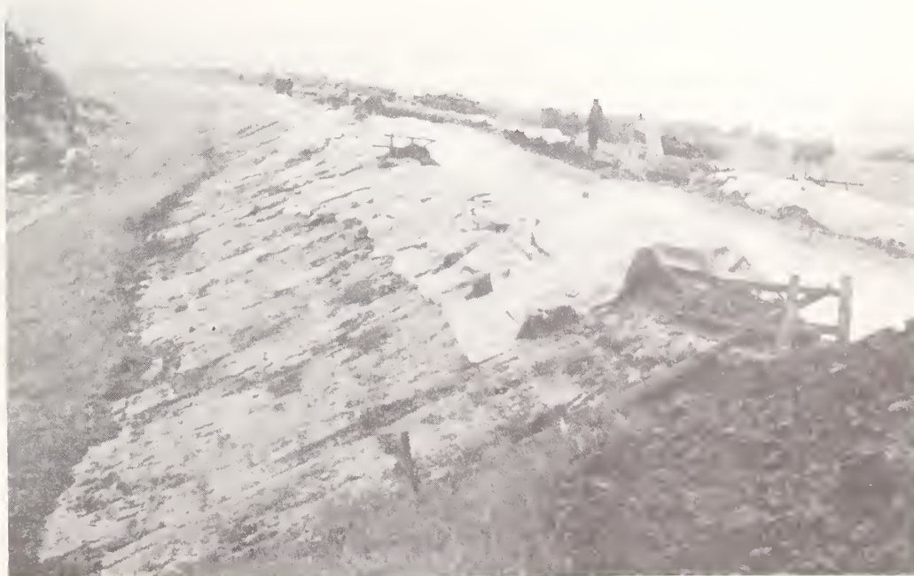
Figure 8.17 Site 6, New Kitakami River. View east along crest of dike and highway that are being repaired. Uneven nature of highway surface is due to liquefaction-induced differential settlement. Settlements of up to 1.5 m occurred along a distance of 4 km.
