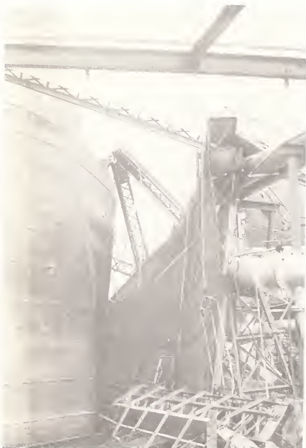
Figure 6.33 Haranomachi Plant, Sendai City Gas Bureau: damage to piping and other equipment and supports caused by impact from the collapsed gas holder and the adjacent pipeway. The newly erected pipeway is to the right.
