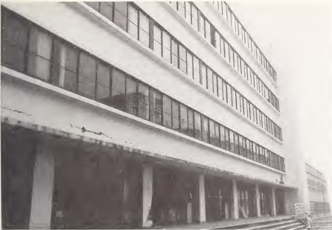
Figure 5.65 Tohoku Institute of Technology. Partial view of the entrance and north facade of building 5. Most serious damage to columns occurred on this side of the building.
