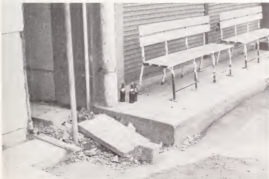
Figure 5.21 Oroshicho area. Sidewalk damage caused by ground settlement.
