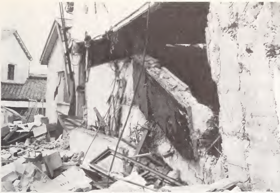
Figure 5.48 Paloma Building. Detail of first story, east end, showing inferior quality concrete.
