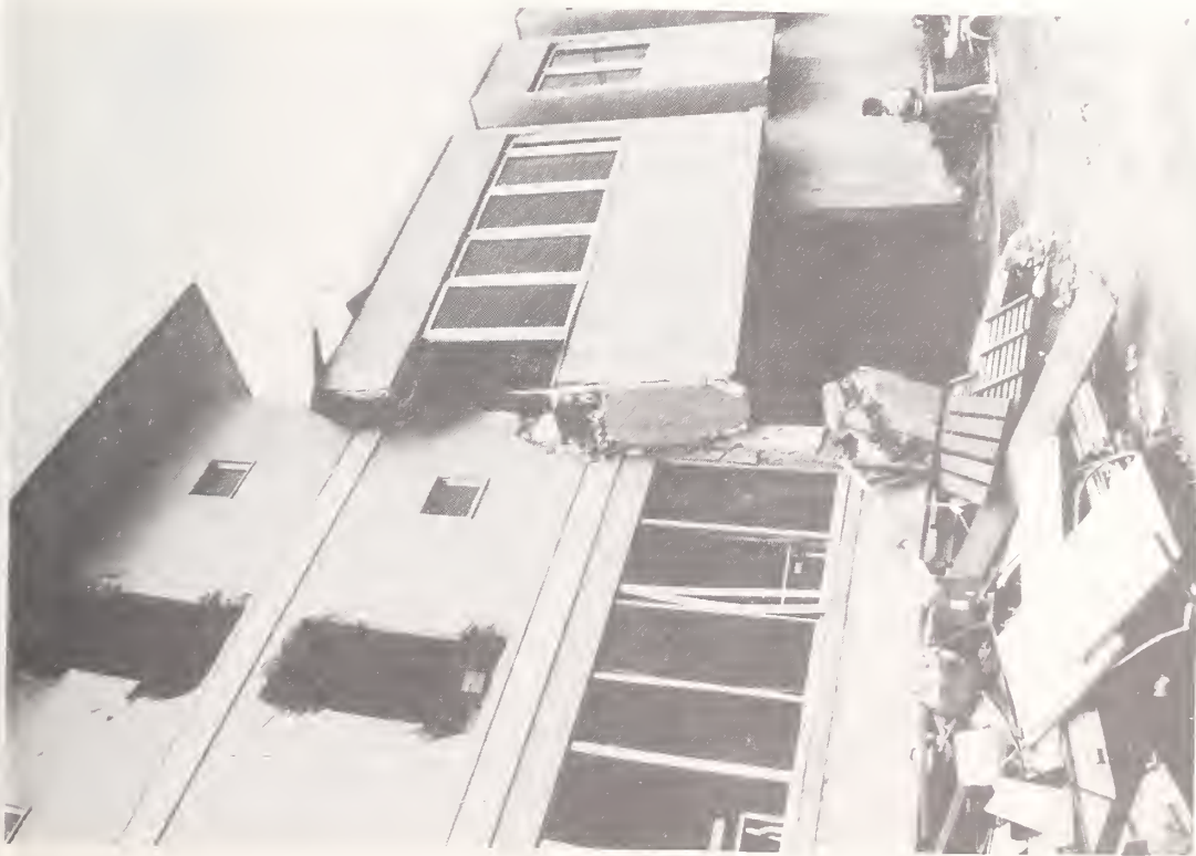
Figure 5.40 Yazaki Industries, showing area of impact between steel and reinforced concrete frames.
