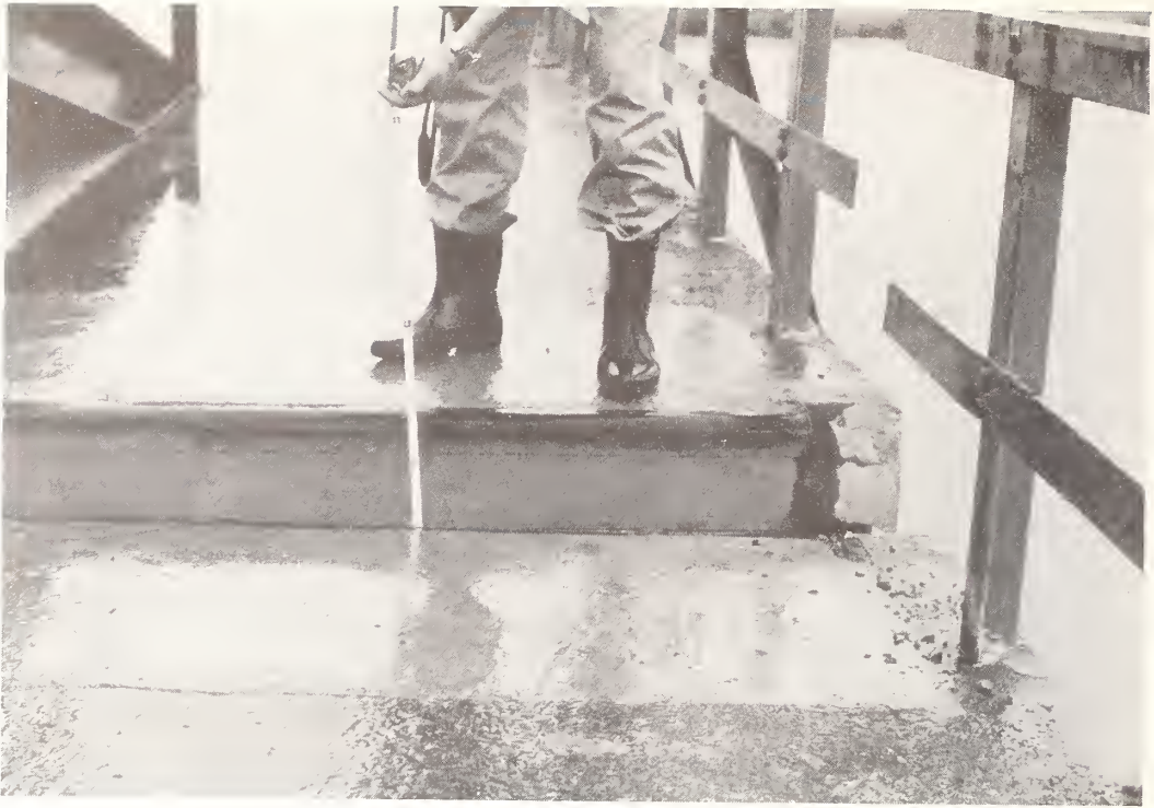
Figure 7.39 Vertical displacement of dislodged span.
