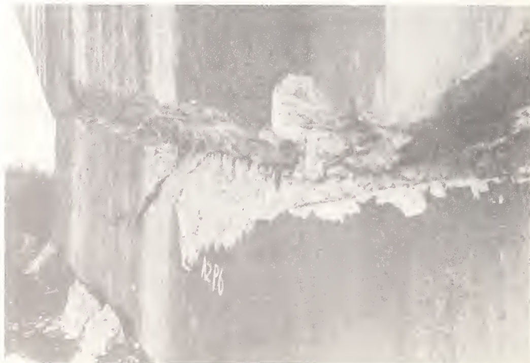
Figure 7.22 Sendai Ohashi Bridge. Typical pier damage at the construction joint between pier and cap. The vertical rebars are buckled across the joint. Significant concrete spalling is evident. Horizontal cracking around the pier was discovered upon excavation of soil around the piers. (Courtesy J.M.O.C.)
