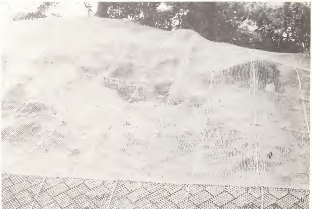
Figure 7.46 Wire mesh screening used to contain land and rockslides along highways.
