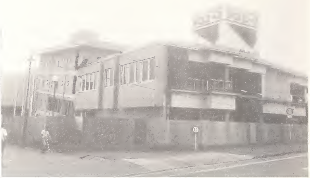
Figure 5.38 Yazaki Industries Buildings, viewed from the northeast, Oroshicho area. Portions of three Yazaki buildings are shown. Failure of the reinforced concrete middle building caused it to rack forward against the front steel structure.
