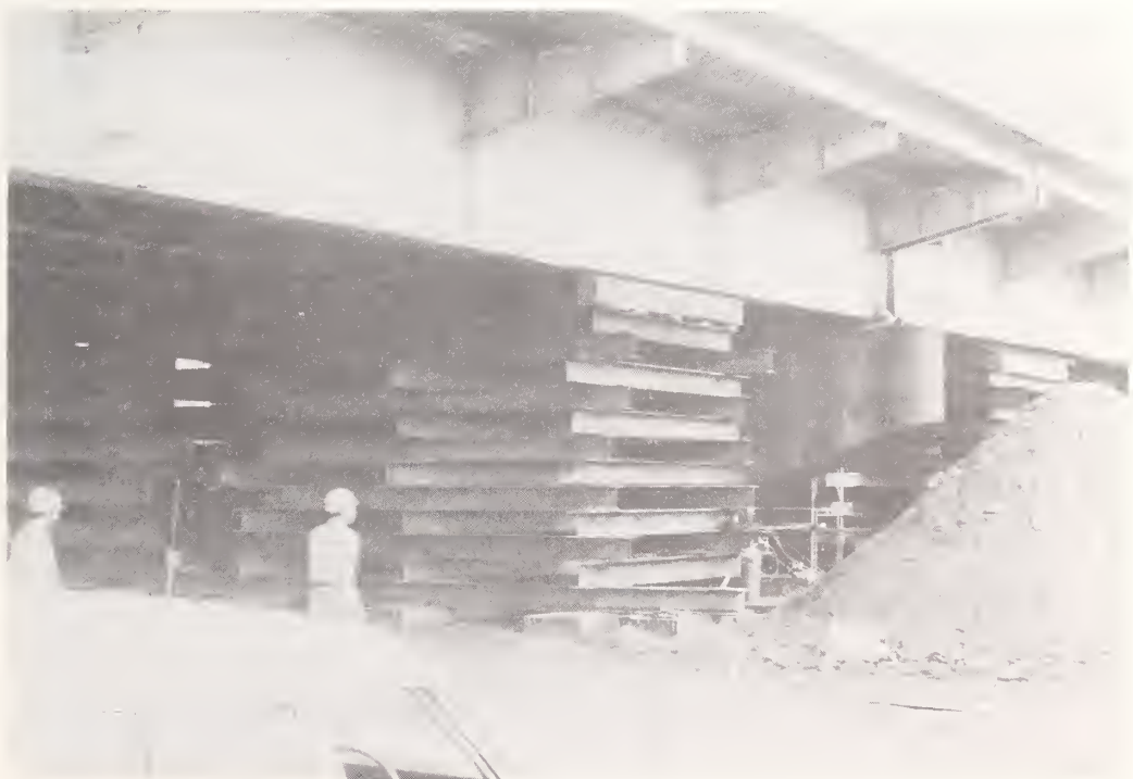
Figure 7.20 Sendai Ohashi Bridge. Temporary cribbing used to support the steel plate girders.
