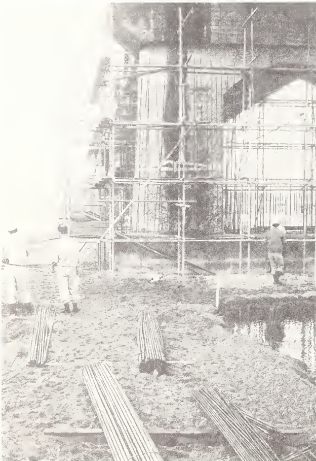
Figure 7.30 Abukuma Bridge. Typical repair of a damaged pier includes epoxy injection of cracks, epoxy covering of buckled rebar, preparation of existing concrete surface to accept fresh concrete, emplacement of vertical rebar into the footing and horizontal rebar into the pier, and an increase of the gross cross sectional area of the pier with new concrete. The technique is similar to that used on the Yuriage and Sendai Ohashi bridges.
