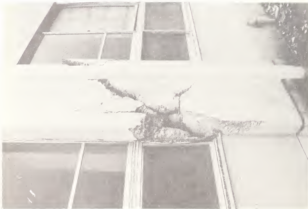
Figure 5.55 Tonan High School. Detail of shear cracking in exterior column above partial infill panels on east face
