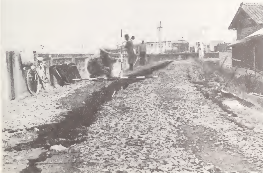
Figure 8.7 Site 2, Natori River. Settlement, lateral spreading, and longitudinal cracking of dike. View is east. (Photo courtesy Tohoku Regional Construction Bureau)
