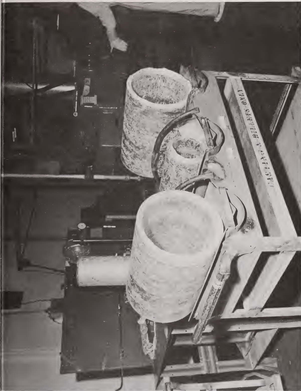
Fig. 6. Uranium-Aluminum Castings of Various Sizes.
