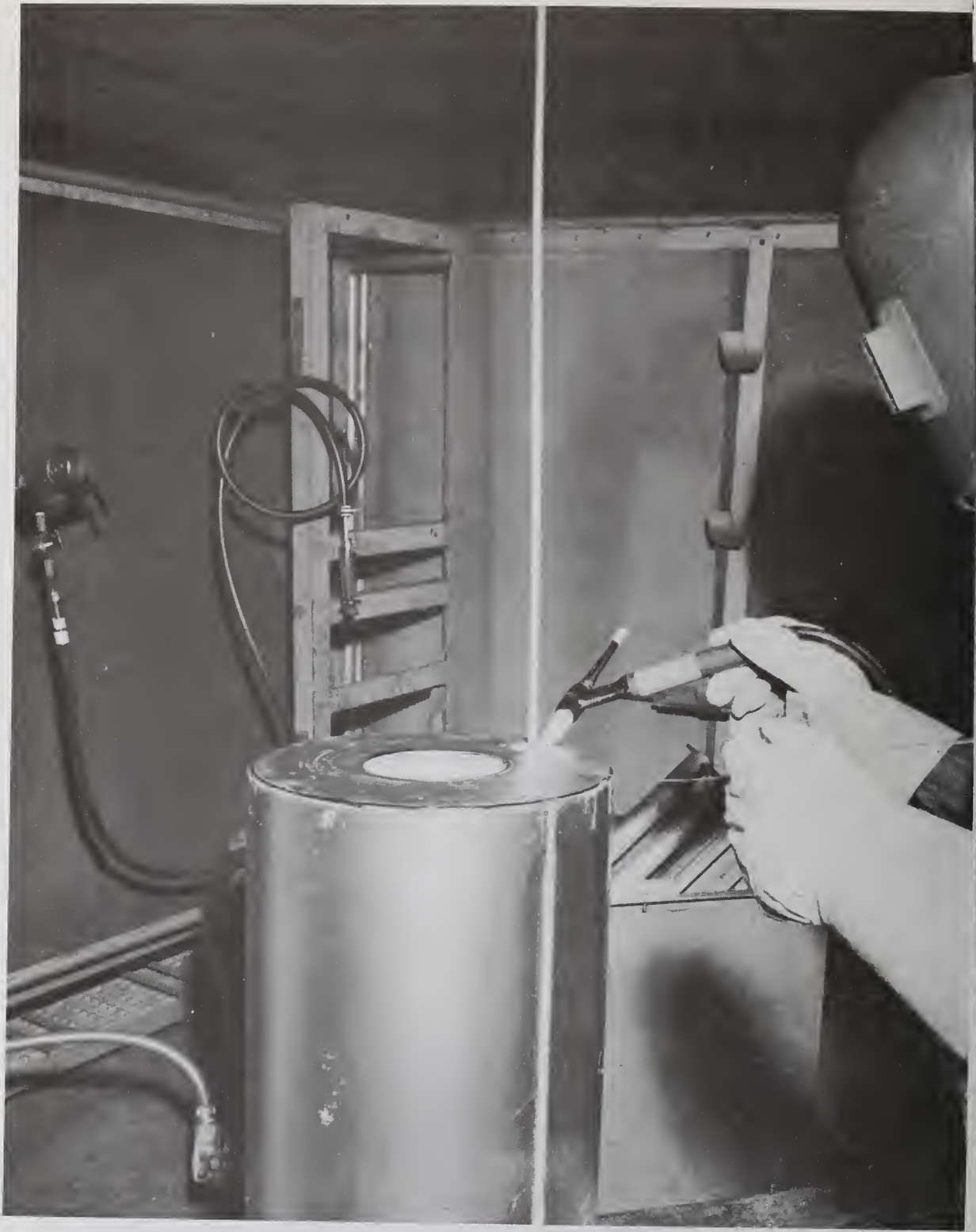
Fig. 9. Welding Pre-extrusion Billet.
