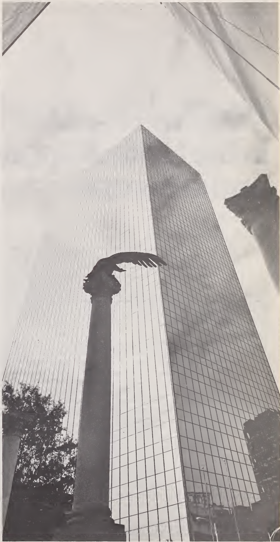
Figure 8. Marietta Tower, Atlanta. This building has more spandrel area than vision area (only 38 per cent of facade)
