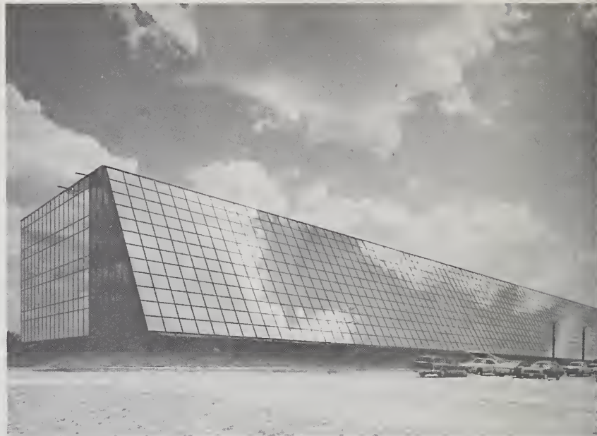
Figure 3. Century Center, San Antonio. Gold reflective glass on the sloping wall makes it possible to provide a people-occupied four-story garden
