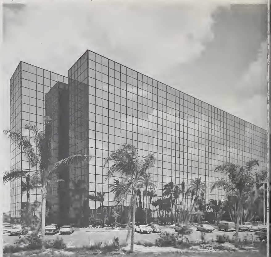
Figure 6. Lincoln Center, Tampa. Though this looks like a 100 per cent glass building, 50 per cent of the facade is spandrel area
