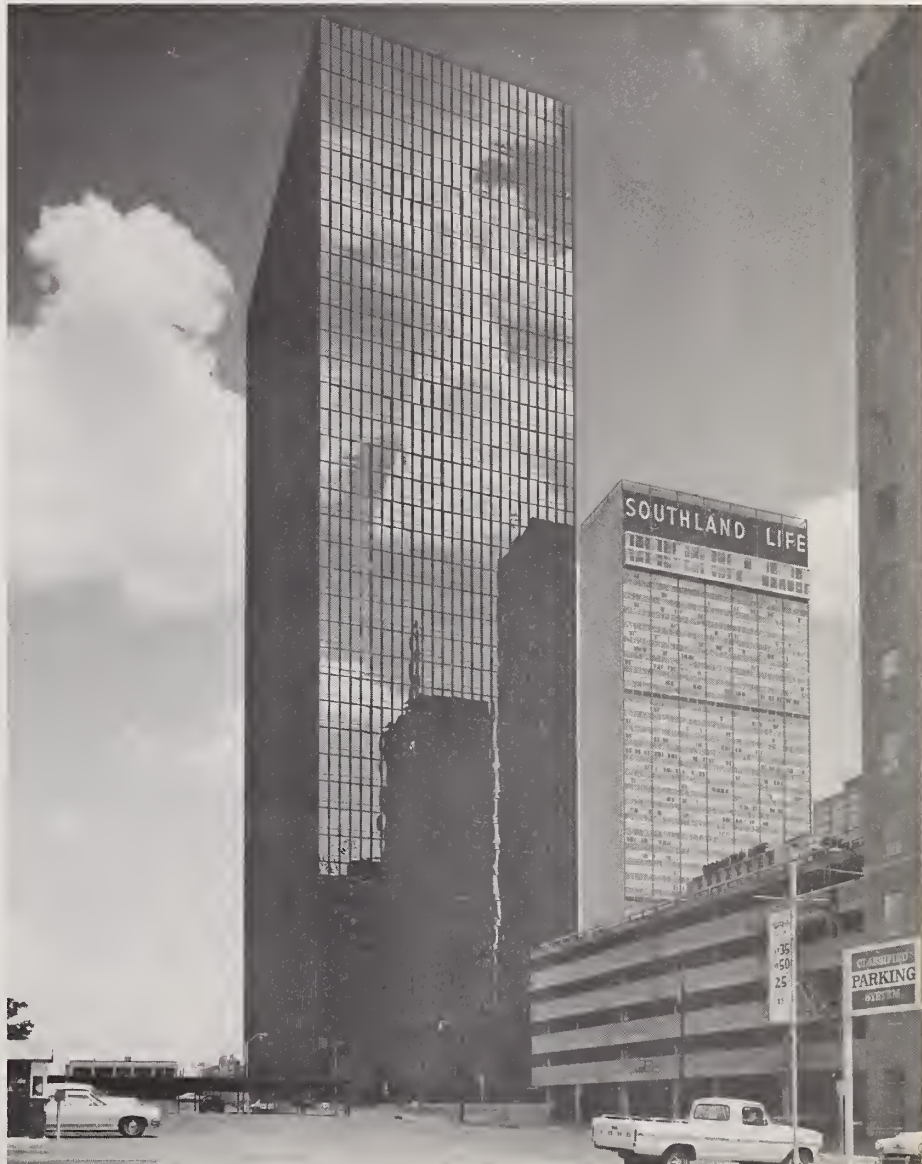
Figure 2. Bryan Tower, Dallas. A 100 per cent vision-glass facade (drapery pocket at spandrel)
