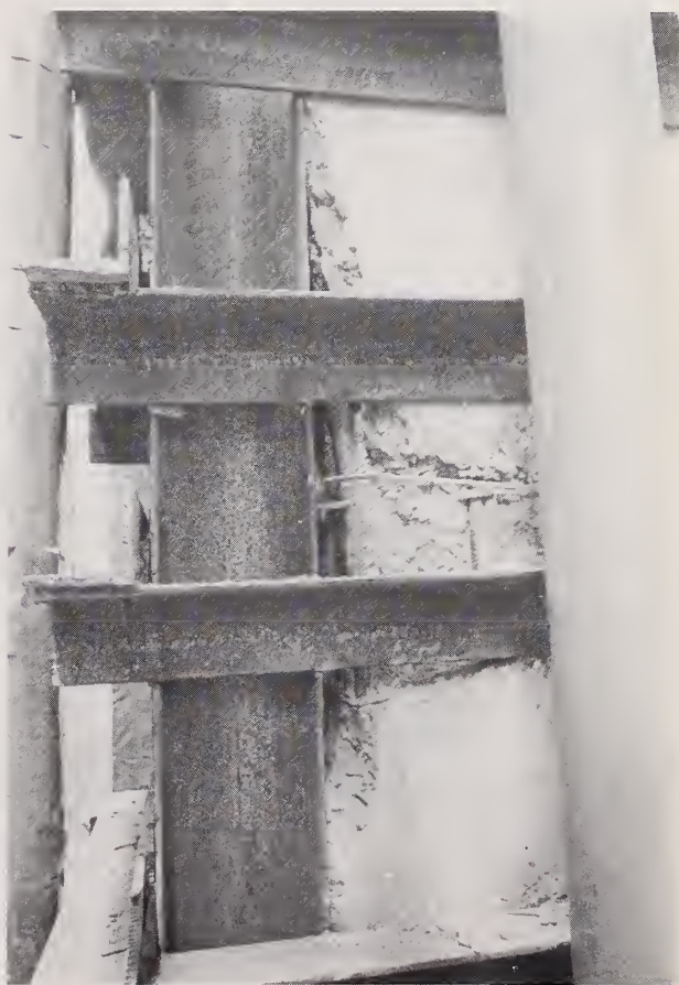
Figure 3.65. Close-up view of steel framing used for confinement of ruptured column.
