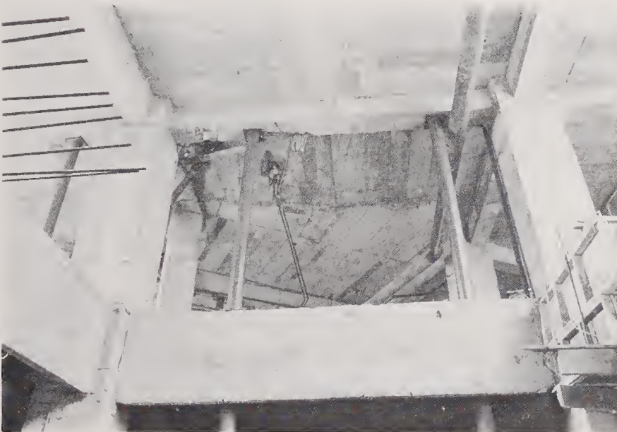
Figure 3.69. Metal pipes used in shoring damaged transverse beams.
