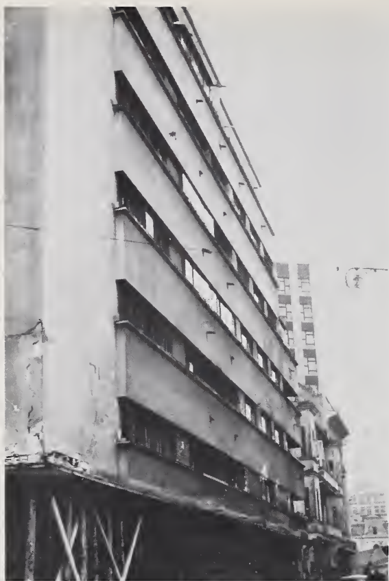
Figure 3.30. West view of Turist building showing substantial facade and masonry damage.
