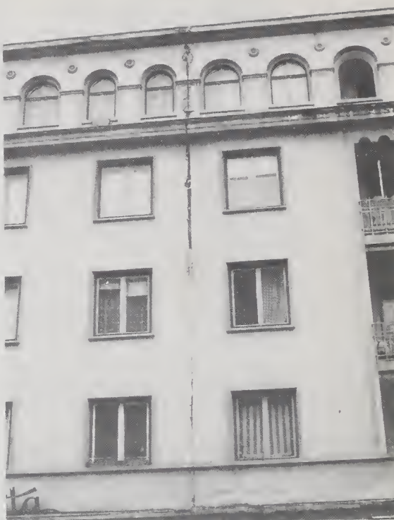
Figure 3.109. Pounding damage between adjacent buildings.
