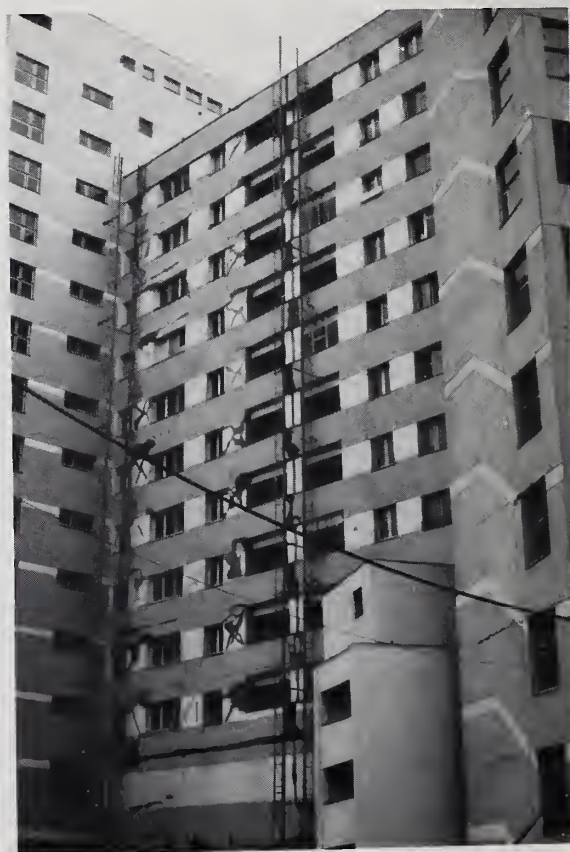
Figure 3.79. Cracking of exterior piers in multistory building.
