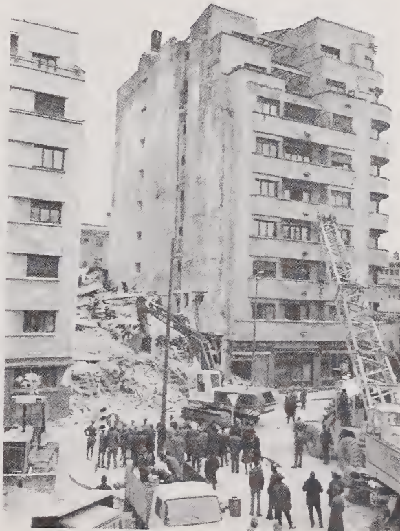
Figure 3.5. Multistory apartment on Sahia Street near corner of Piata Rosetti totally destroyed by the earthquake.
