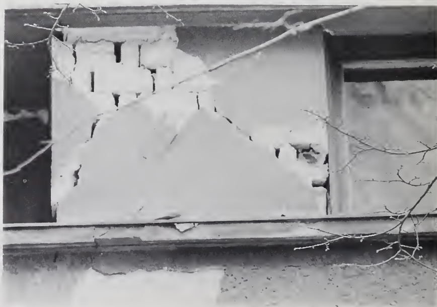
Figure 3.31. Close-up of damaged masonry pier beneath spalled plaster.
