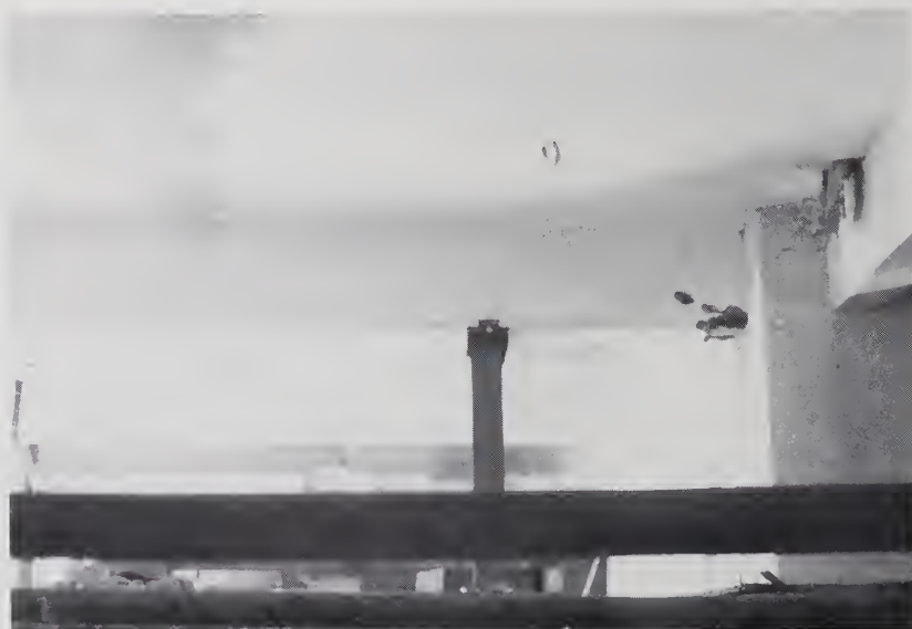
Figure 3.71. Shoring of damaged first story beam in multistory concrete frame building. (Building No. 18)
