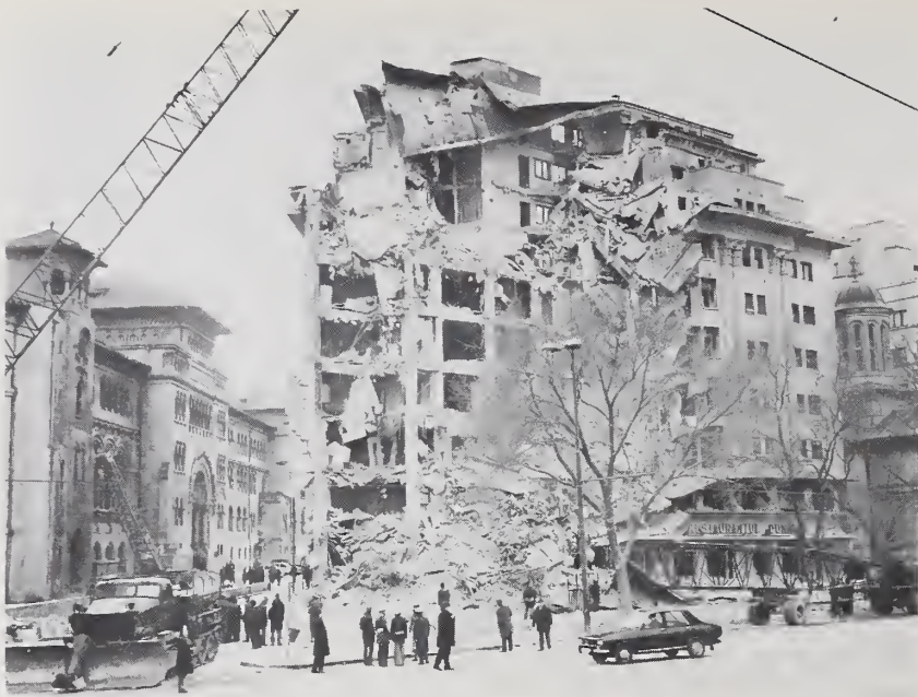
Figure 3.14. View of partially collapsed Dunres building before removal of debris.
