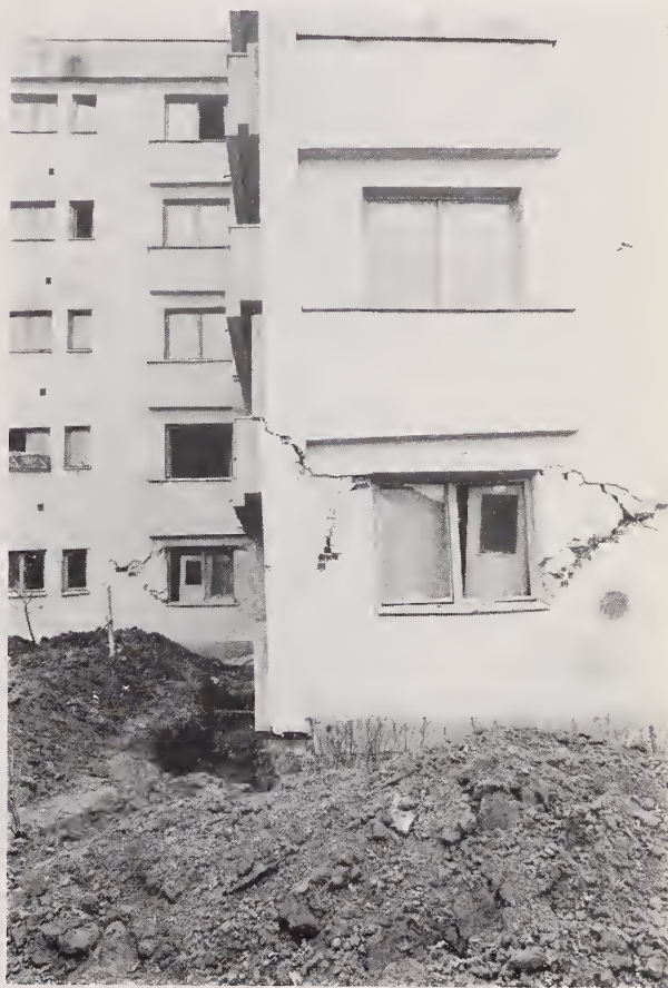
Figure 3.105. Damage of first-story exterior bearing walls.
