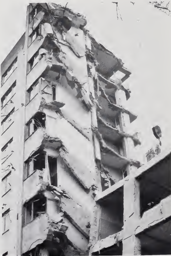
Figure 3.43. Close-up view of region collapsed stairs.
