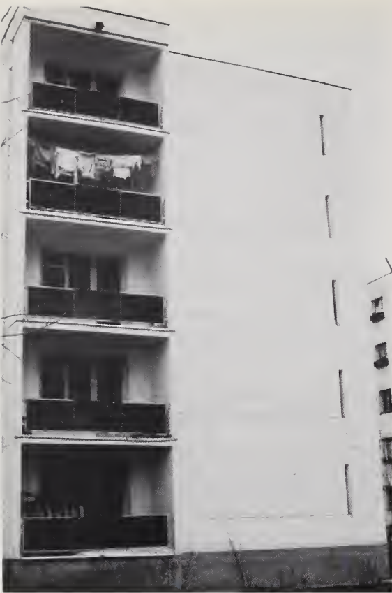
Figure 3.86. End view of 5-story panel building.
