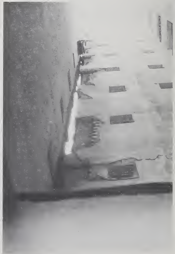
Figure 3.83. Heavy pounding damage to buildings with adjacent corners.
