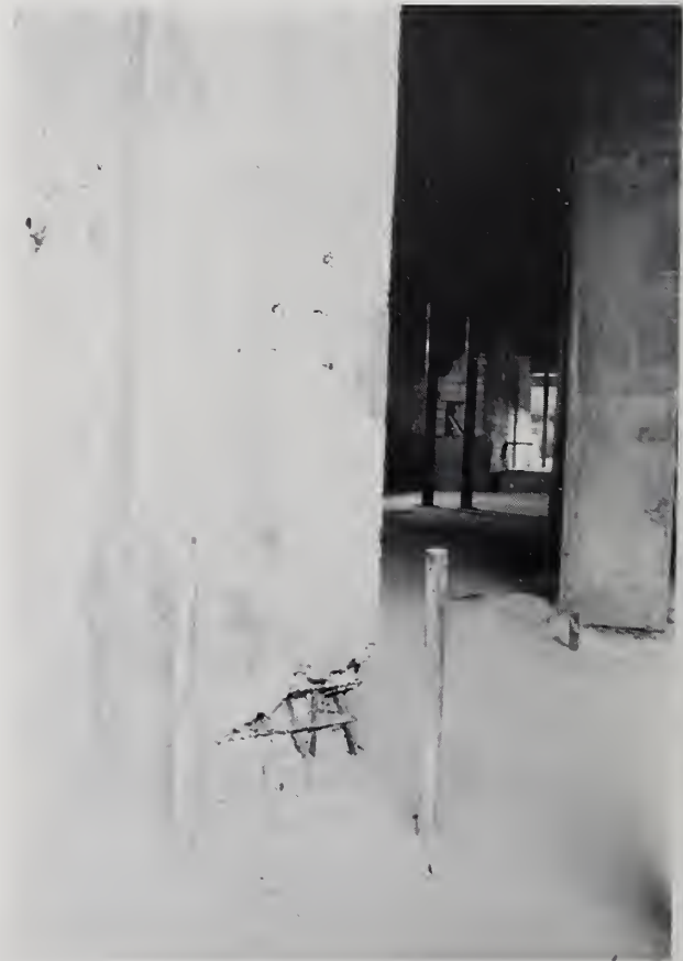
Figure 3.67. Damage at the base of first story interior column.
