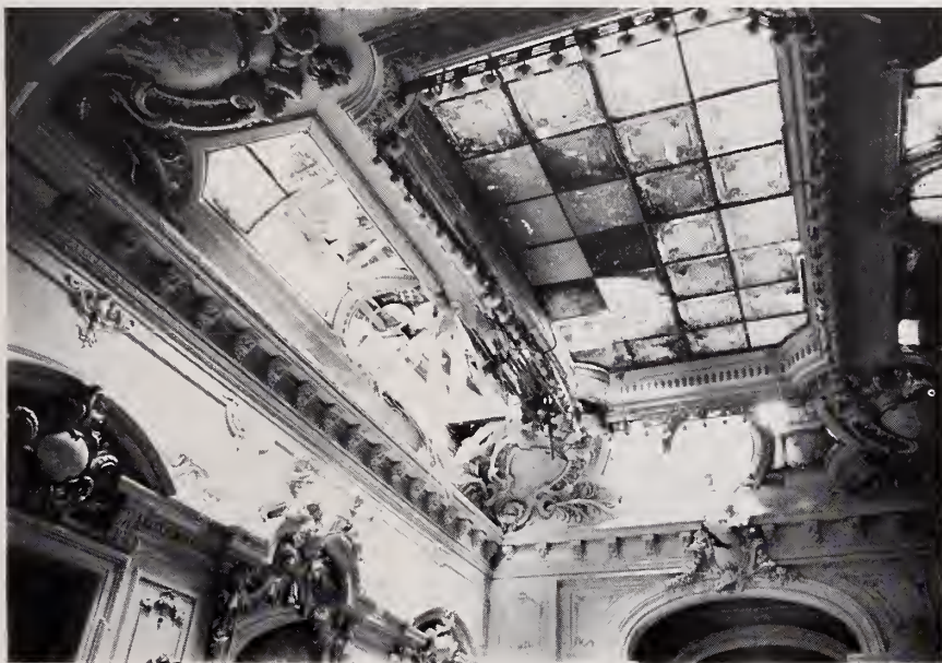
Figure 3.101. Damage of decorative skylight within the first story of the museum.
