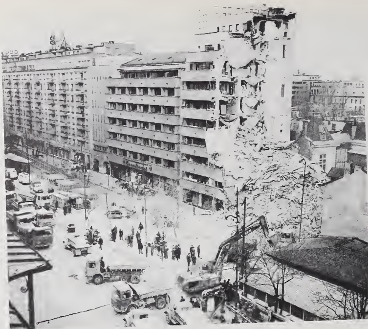
Figure 3.22. General view of the collapse of the end bays of Casata building.
