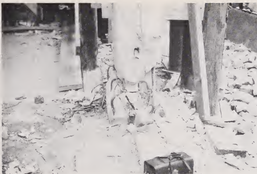
Figure 3.20. Failure of interior first story column at the base indicating lateral displacement.
