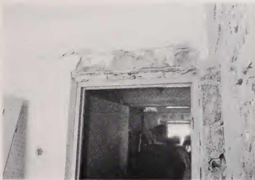
Figure 3.108. Damage of lintel wall in first story.
