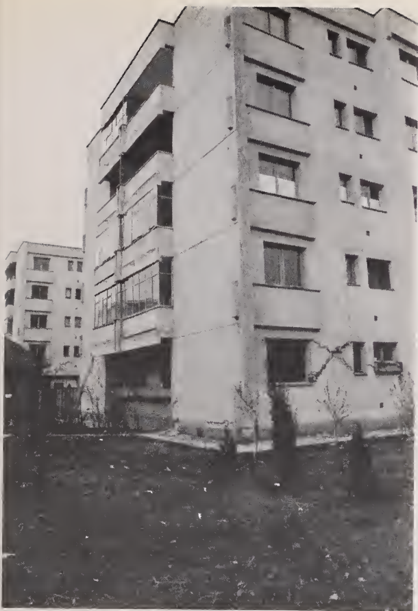
Figure 3.104. General view of load-bearing masonry apartment building.
