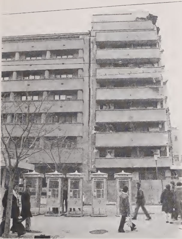
Figure 3.24. Damage due to pounding of the Casata building with the next structure.
