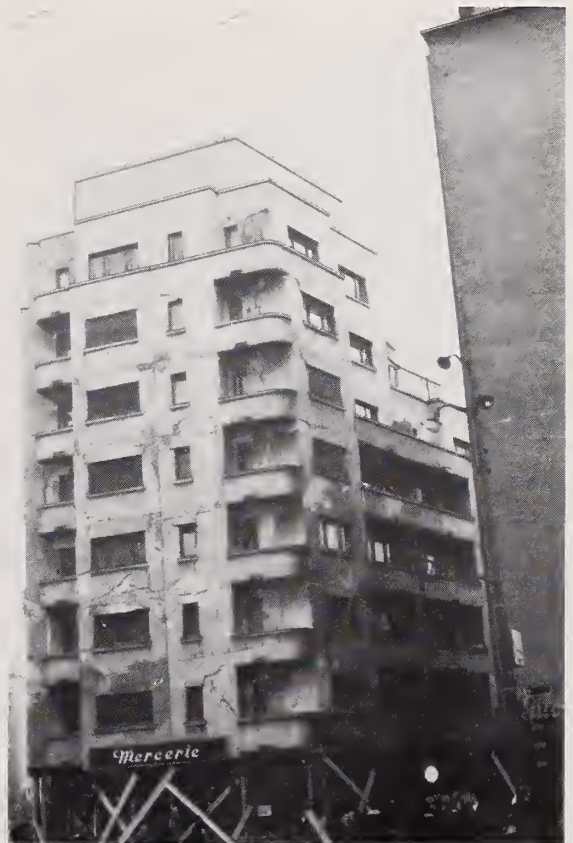
Figure 3.37. Another view of Mercerie building showing configuration of upper story setbacks.
