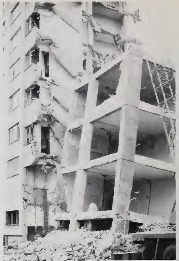
Figure 3.42. Rear corner view of collapsed end bays after tearing down of walls by wrecking crew.
