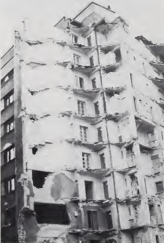
Figure 3.35. Left view of the collapse Metalimport building.
