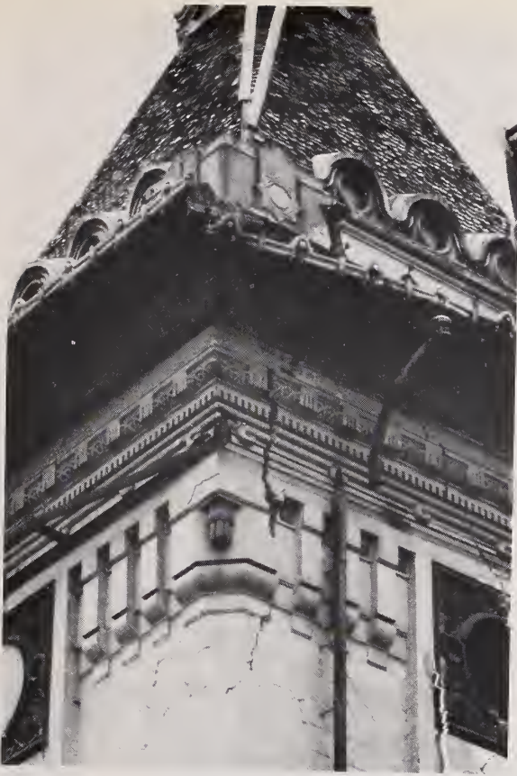
Figure 3.96. Close-up view of damaged tower of city administration building.
