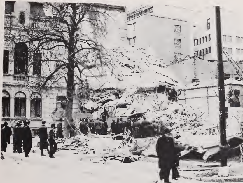
Figure 3.9. Partial collapse of three-story residential building on Snagov Street.
