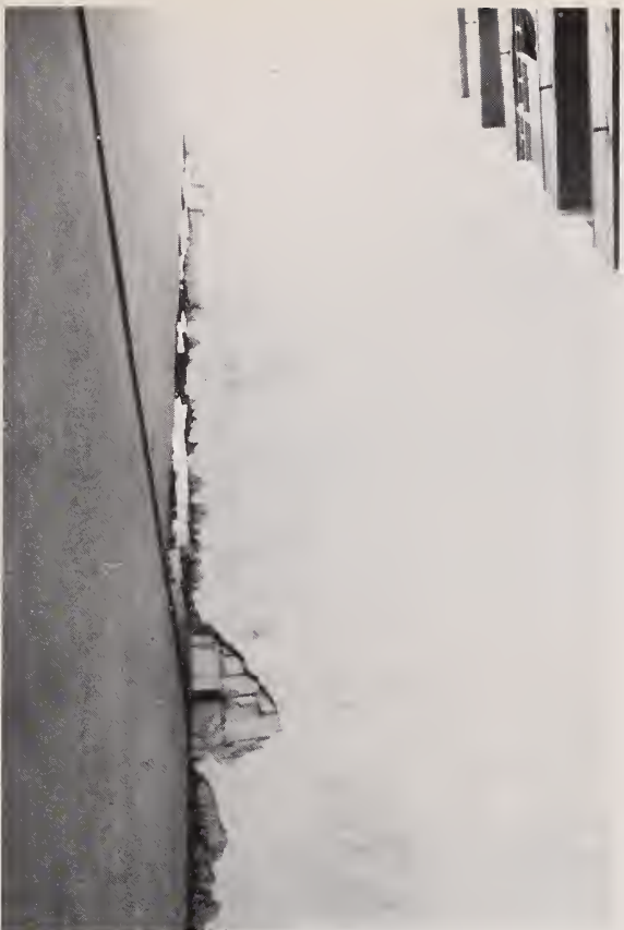
Figure 3.84. Same pounding damage viewed from the opposite side.
