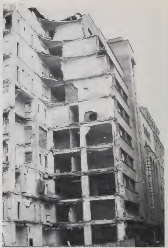
Figure 3.34. Partial collapse of 10-story Metalimport building.
