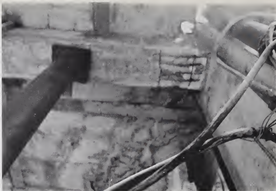
Figure 3.70. Failure of transverse beam at the support.
