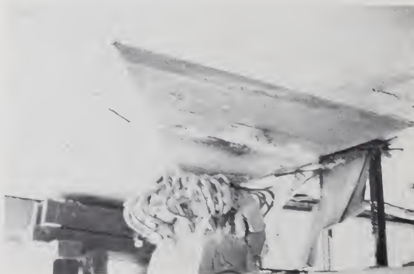
Figure 3.55. Failure at the top of the northwest column in the first story.
