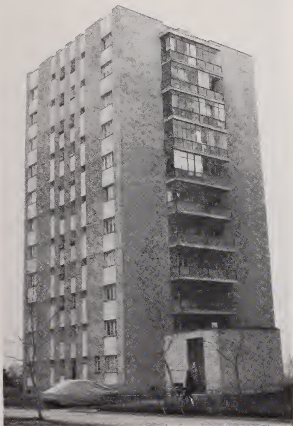
Figure 3.89. Eleven-story slip-formed shear wall building.
