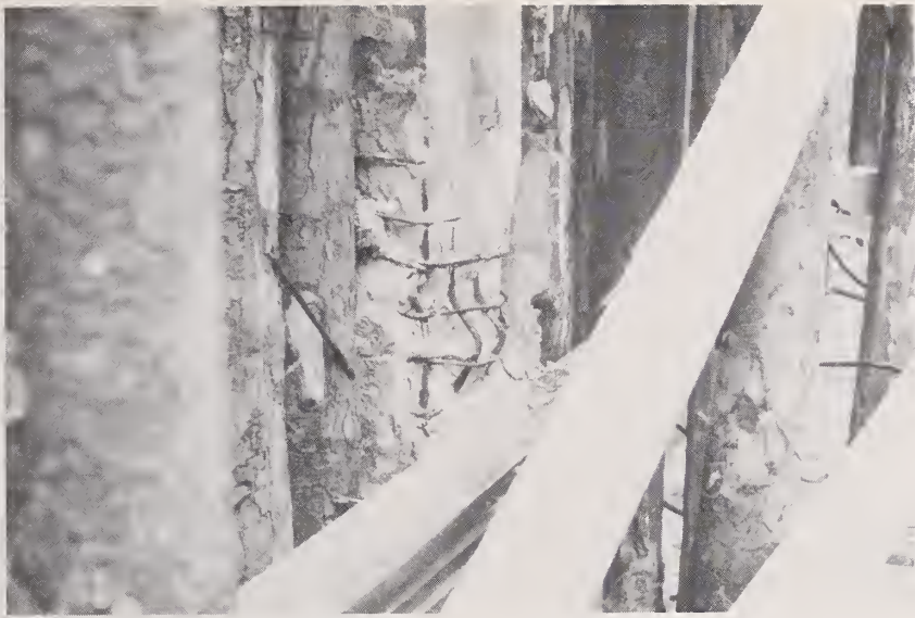
Figure 3.32. Interior view showing failure of first story column at the base.
