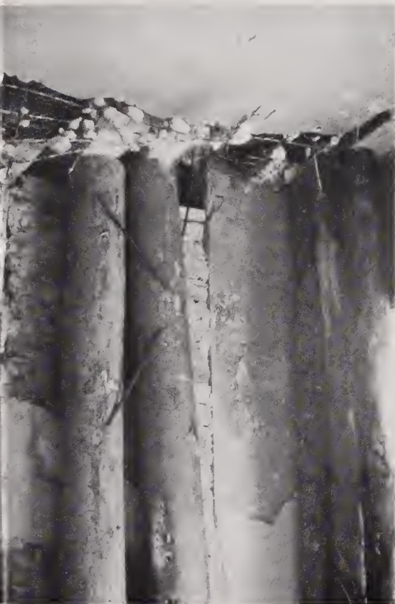
Figure 3.32. Interior view showing failure of first story column at the base.
