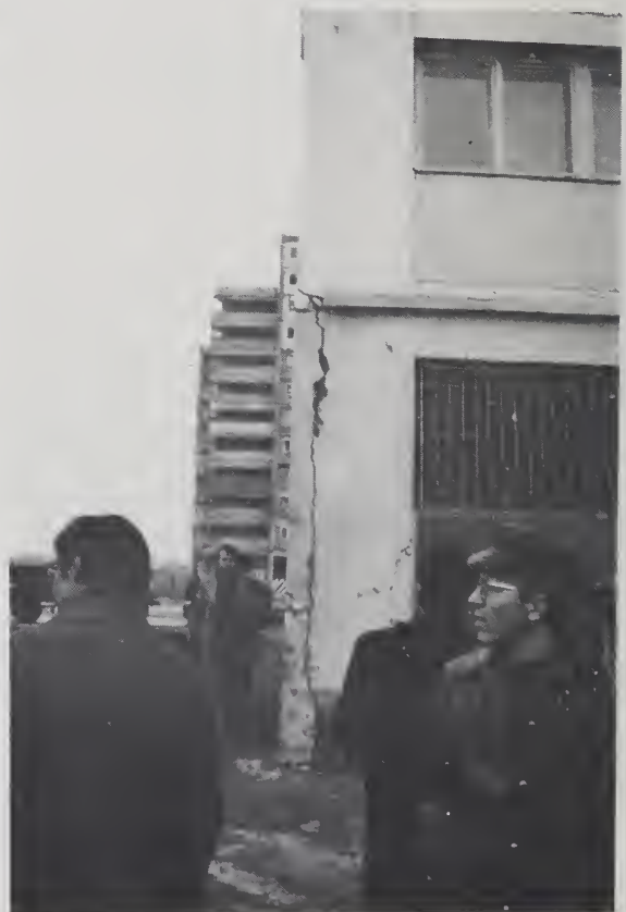
Figure 3.59. View of rear corner of Building 16 showing detached insulation wall.
