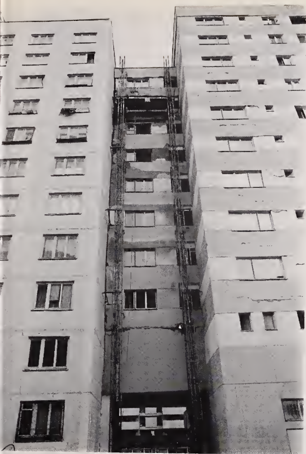
Figure 3.80. General view of superficial damage in concrete frame building next to shear wall building on the left.
