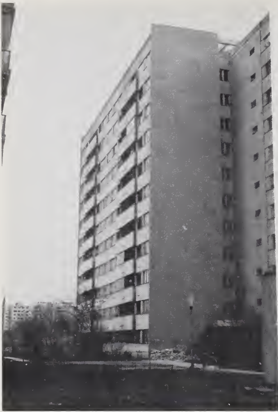
Figure 3.90. Another 11-story slip-form shear wall building.
