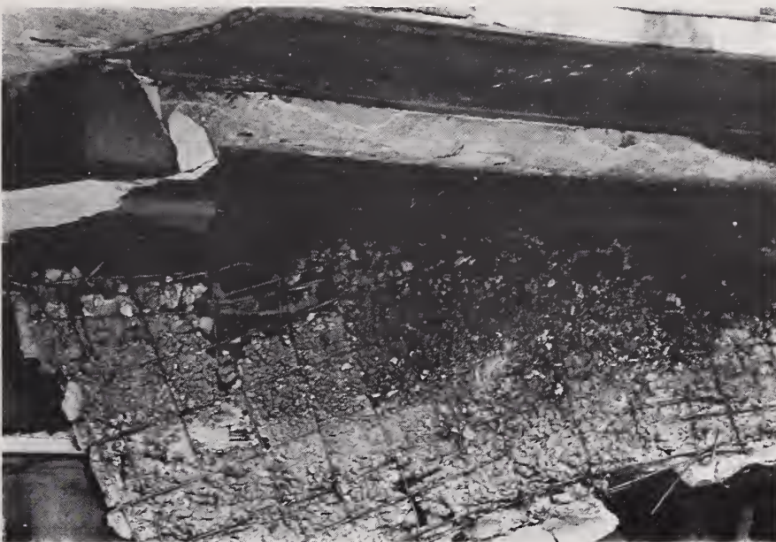
Figure 3.29. Close-up view of detached soffit of the canopy over the sidewalk.
