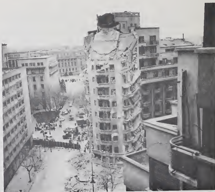
Figure 3.7. General view of failure of Wilson apartment building.
