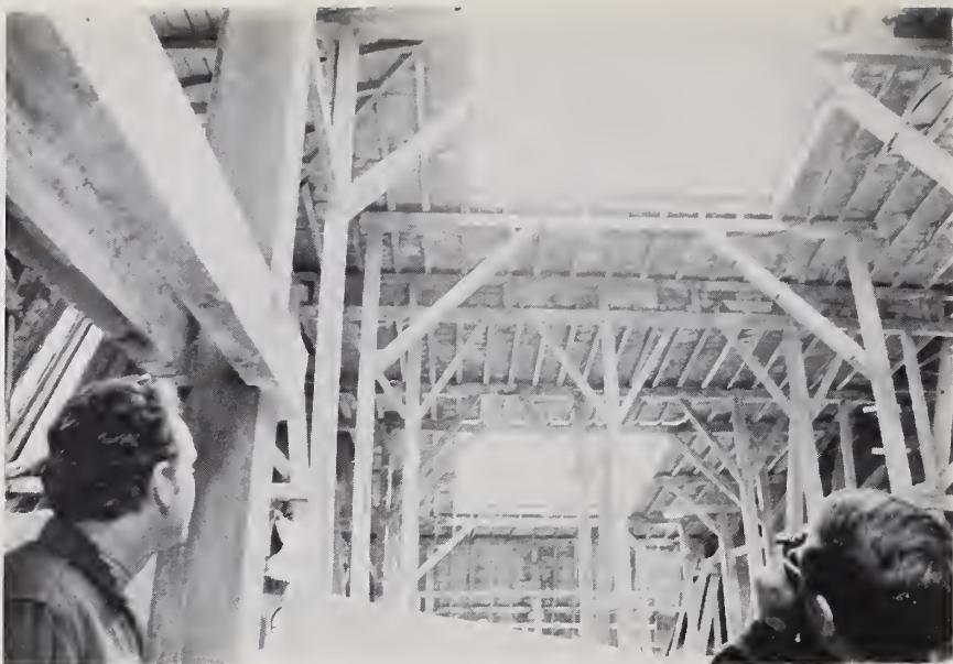
Figure 3.102. Timber framing of the roof within the museum attic.
