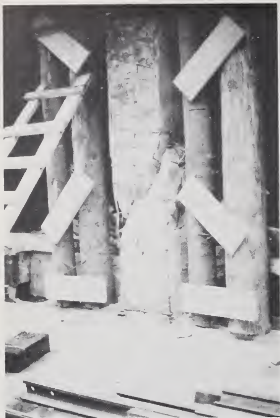
Figure 3.26. Damage to interior column in the first floor.
