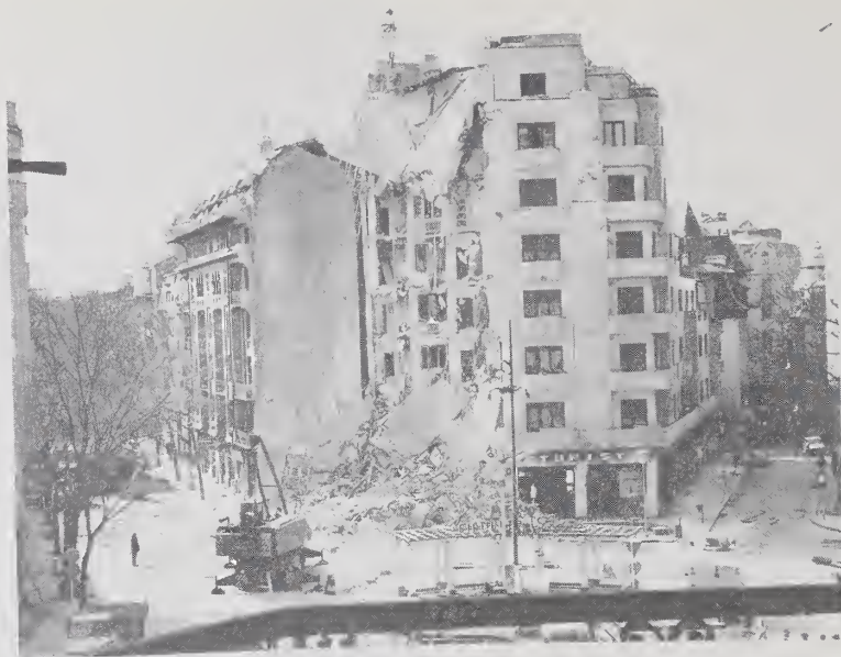
Figure 3.18. Partial collapse of Lido building.
