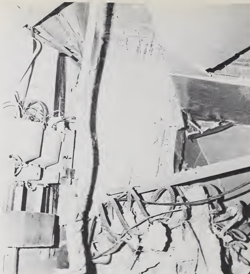
Figure 3.54. Failure of second story column located in the air conditioning room.
