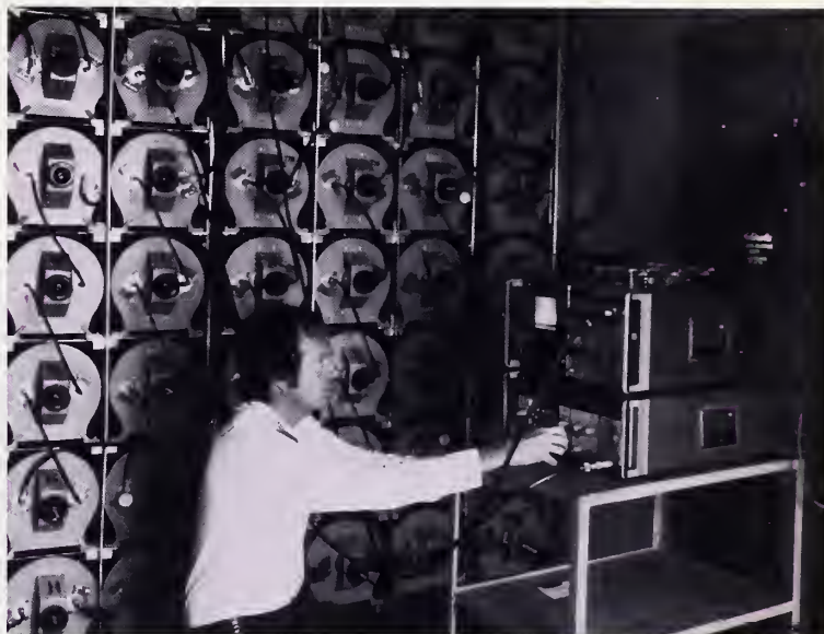
Figure 17. A cavity resonator installation for 39 MHz. (Photograph courtesy of Los Angeles County Communications Department.)
