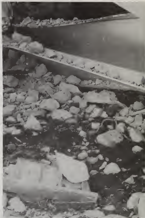
Figure 8 Agua Caliente Fallen Expansion Rocker, Base of Pier 3
