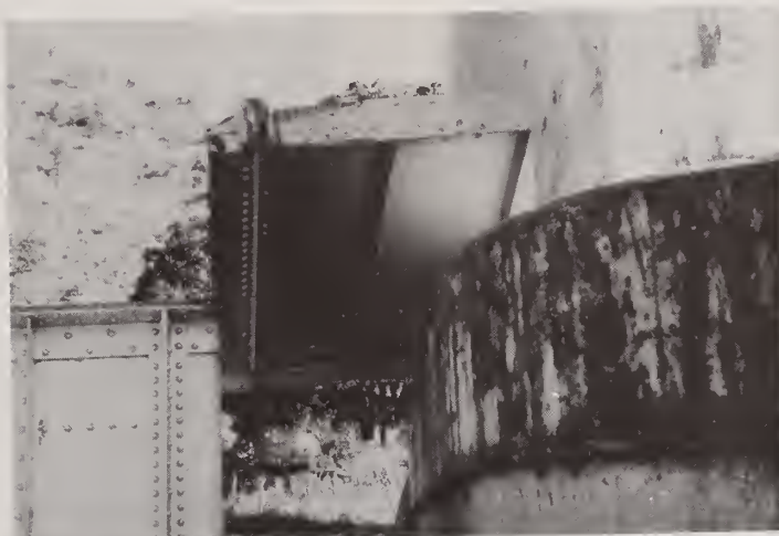
Figure 4 Agua Caliente - Longitudinal Girder Displacement, Base of Pier 2
