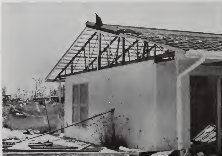
Fig. 16. Prefabricated house with asbestos cement-polyurethane sandwich panels and steel wall and roof frames
