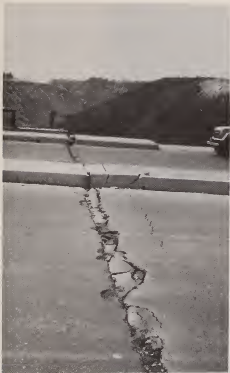
Figure 25 Incienso - Pavement Cracking at West Abutment
