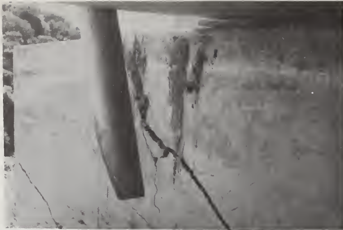
Figure 16 LaAsuncion - West Abutment Wall Damage
