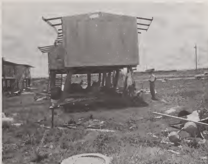
Fig. 6. Failure of concrete block shear walls and racking of concrete piers
