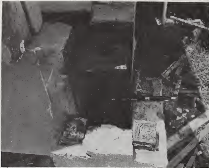
Fig. 15. Beam to column connection - precast concrete high-set
