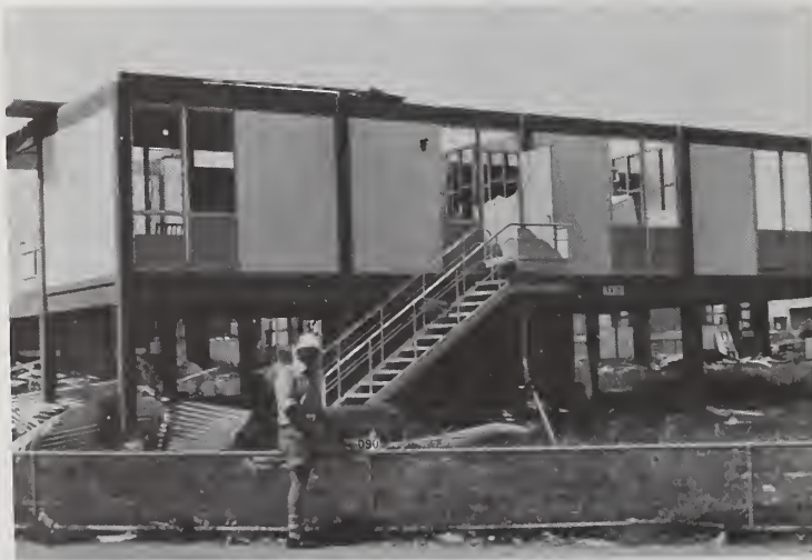
Fig. 12. High-set house with precast concrete frame and interlocking precast concrete panels.
