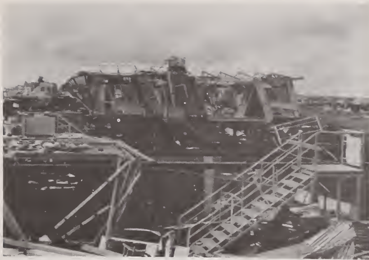
Fig. 5. Severe racking and loss of timber deck
