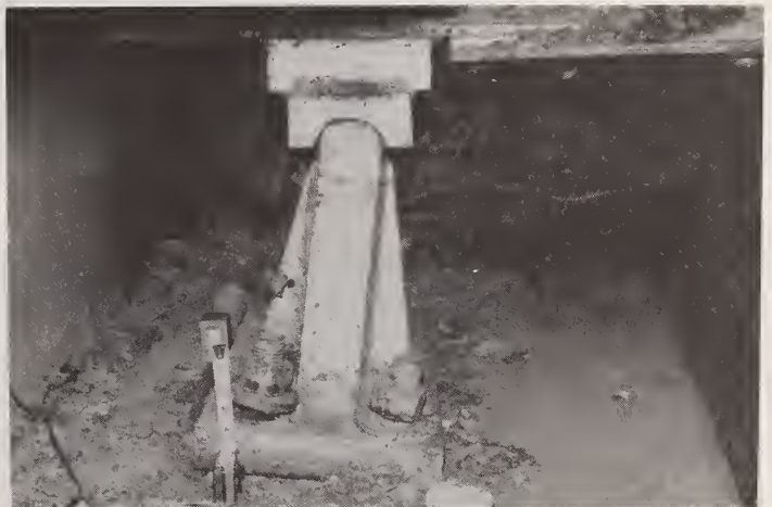
Figure 11 Agua Caliente Bearing Detail, West Abutment, North Girder
