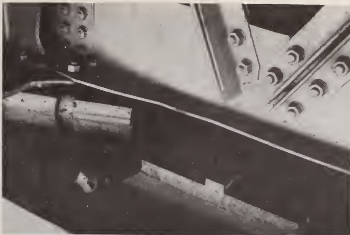
Figure 19 LaAsuncion - Displaced Rocker Bar at West Abutment
