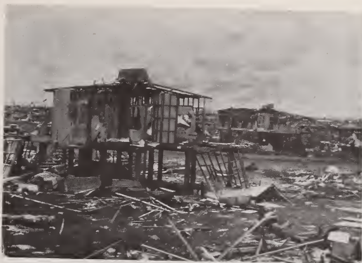
Fig. 9. Failure of endwall
