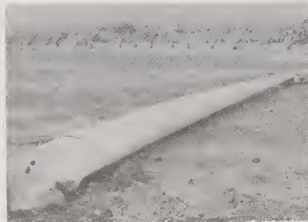
Photo-15. Damage to arc lamp standard (Hachijo High School)
