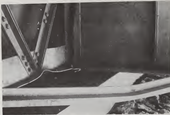
Figure 22 LaAsuncion - Bottom Lateral Bracing and End Diaphragm Damage
