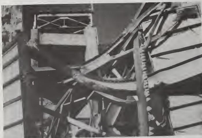
Figure 7 Agua Caliente - Detail of Collapsed Span at Base of Pier 3
