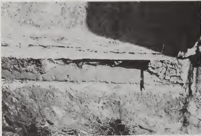
Figure 17 LaAsuncion - West Abutment Foundation Damage
