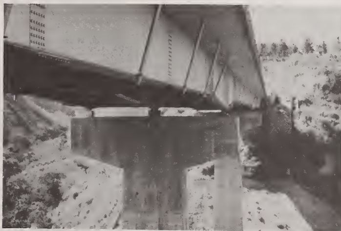
Figure 21 LaAsuncion - Missing Bearing, East Pier
