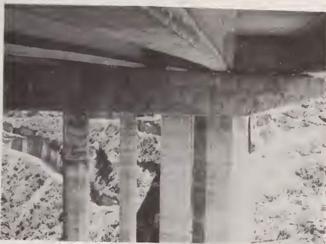
Figure 27 Incienso - Hinge Restraint, West Pier Bent
