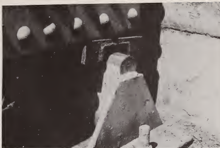
Figure 34 CA9-Typical Damaged Fixed Bearing Detail
