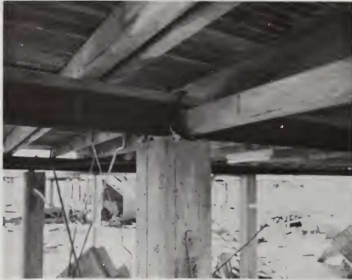
Fig. 7. Typical floor systems and pier anchorage
