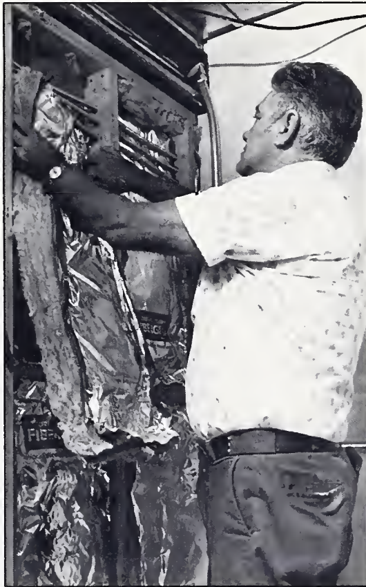
Adding insulation to check energy savings.
