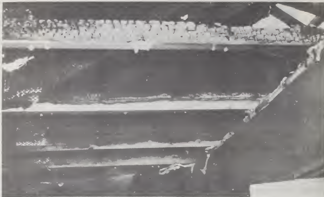
Figure 4. Penetration of the attic void permits fire to attack the top floor ceiling from the upper side - note the burning on the bottom chords of the roof trusses. Water required to extinguish the fire causes the ceiling to drop. Water damage down through the building is often severe.
