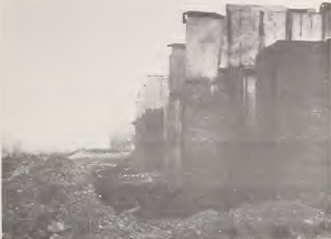
Figure 6. The firewalls were all that was left.
