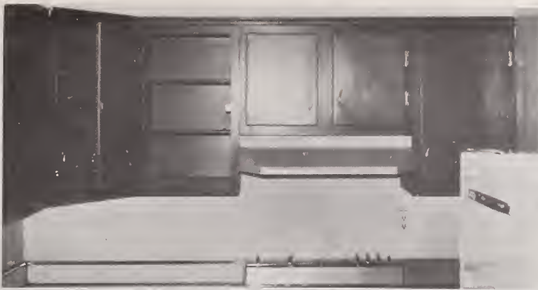
Figure 3. Kitchen cabinets. These "built-in" cabinets are attractive in appearance, but the only barrier between a kitchen fire and the inner voids of the building may be 1/8 inch of hardboard forming the top of the cabinet.
