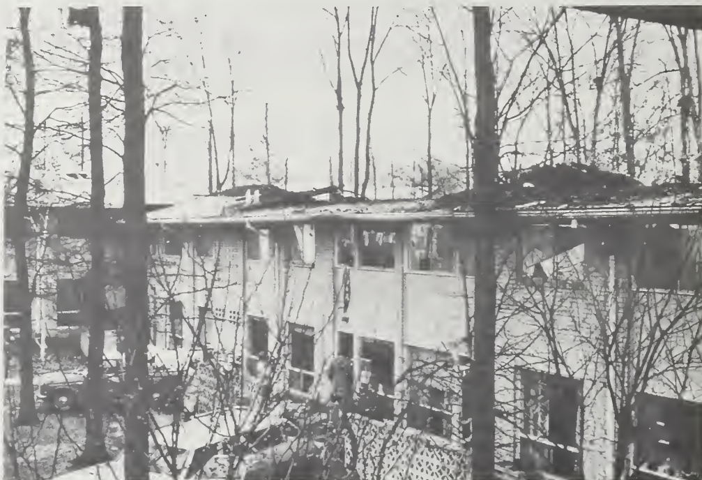
Figure 8. The combustible attic forms a vast horizontal flue.
