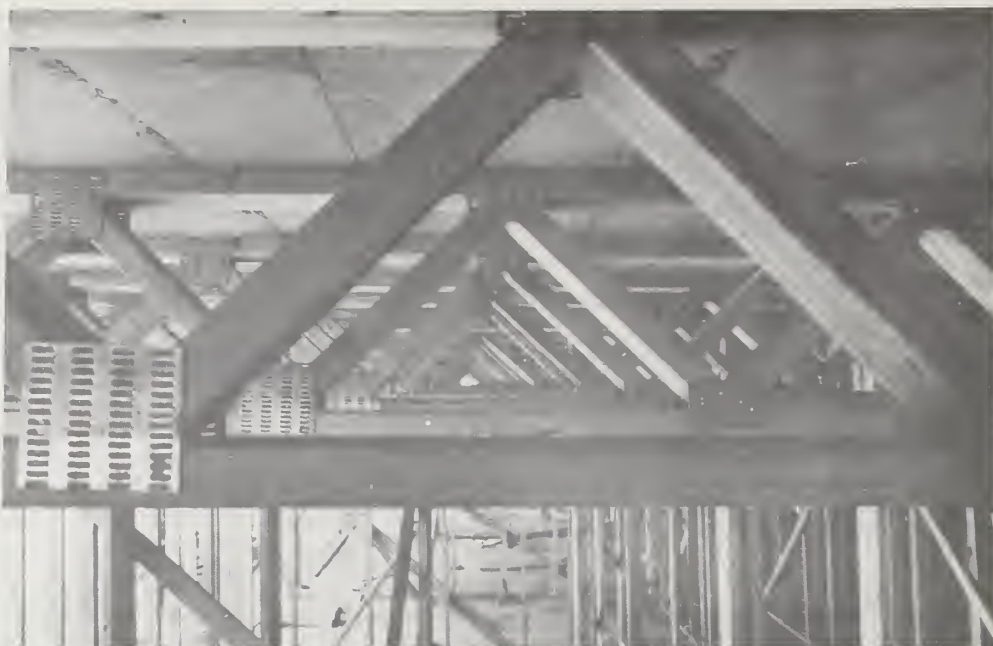
Figure 7. These trussed floors permit a combustible void over and under the four apartments on a floor. Vertical channels may interconnect the several voids. In such a structure it is possible to envision collapse not long after fire penetrates the void.
