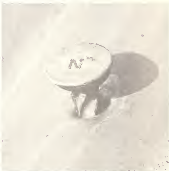
Fig. 3 Protrusion of helically threaded nail from sheet-metal roof of V.P.I. Animal Husbandry Barn.
