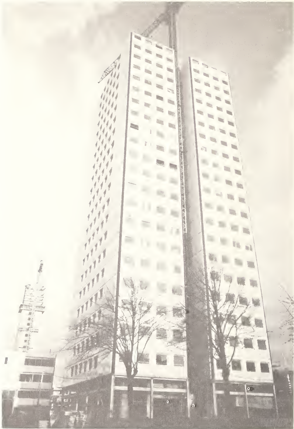
Fig. 1 High-rise Flats for Greater London Council. Wall Panels are Sandwich Composites Combining Several Materials to Meet Performance Requirements.
