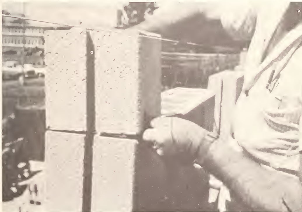
Fig. 3 A ground block being laid in the adhesive mortar
