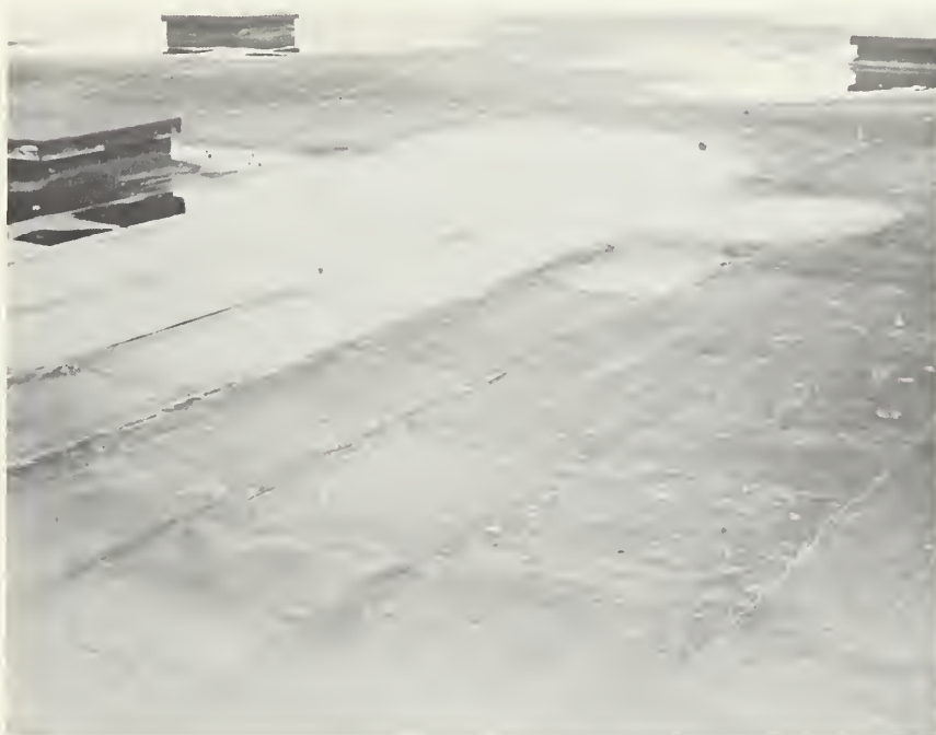
FIGURE 7. Eleven year old asbestos roof membrane providing leak-free service despite extreme deck and insulation movements.
