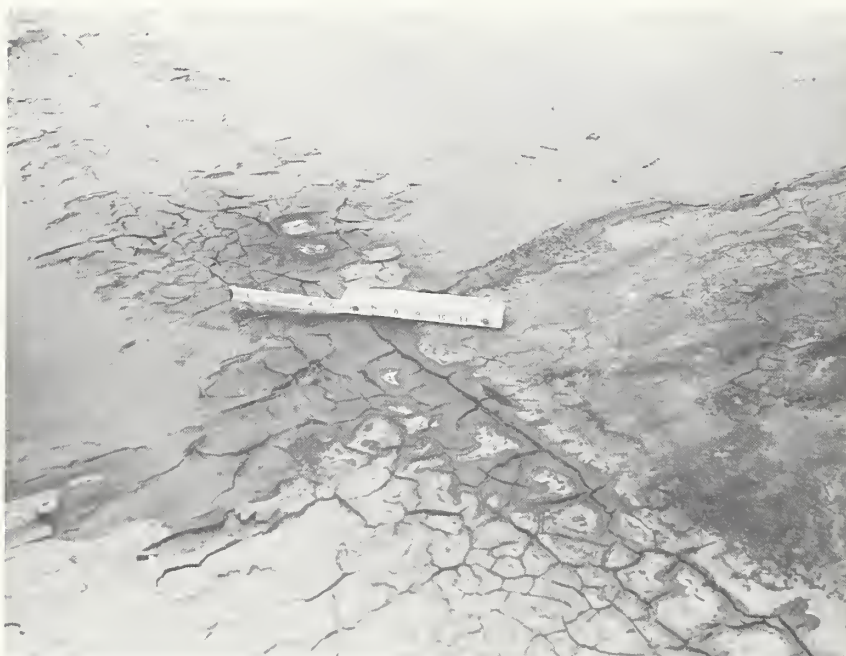
FIGURE 5. Cracking of top coating on smooth surface asbestos built-up roof.
