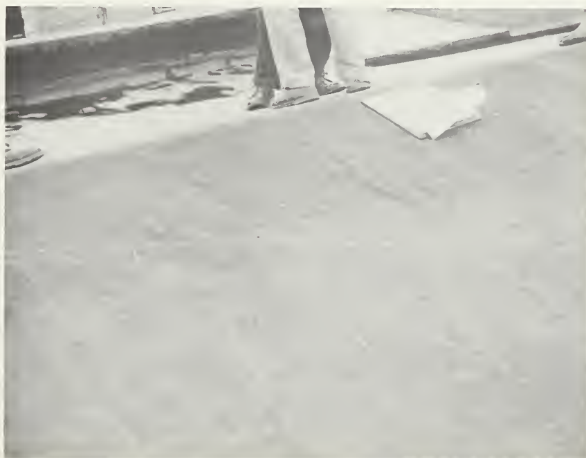
FIGURE 3. Blister caused by poor interply adhesion.
