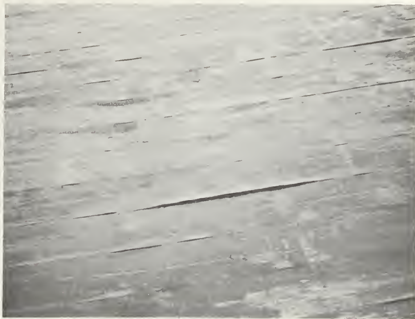
FIGURE 2. Delamination of asbestos felt on smooth built-up roof.
