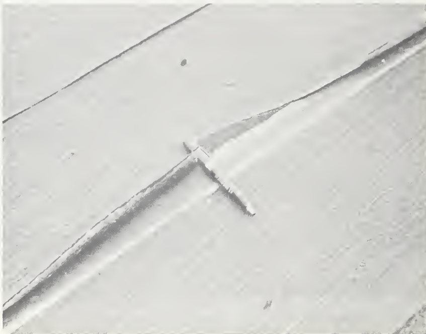
Figure 8. Asbestos felts delaminated and torn. This roof was subjected to several hurricanes.
