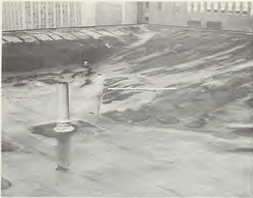
FIGURE 6. Large blister caused by incompatibility of top asphalt built-up roof with that of bottom coal-tar roof.
