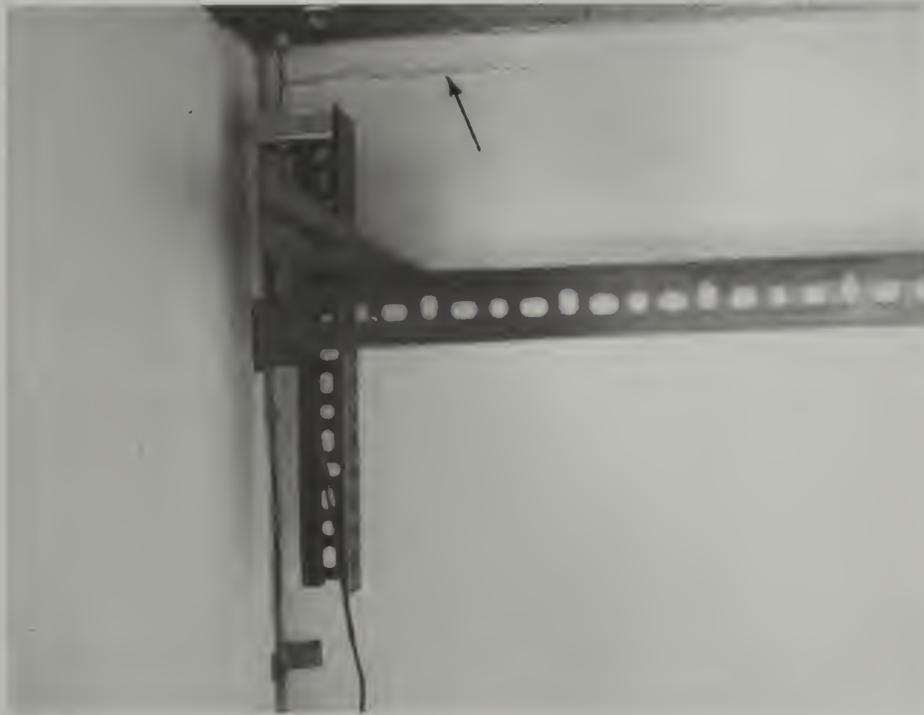
Fig. 9.22 Drywall crack near ceiling on interior side of east wall
