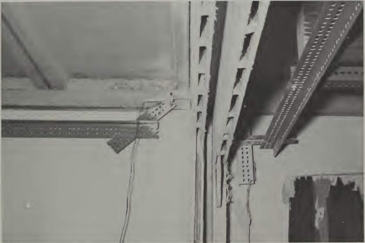
Fig. 5.16 Interior "structicore" wall (partially dismantled)
