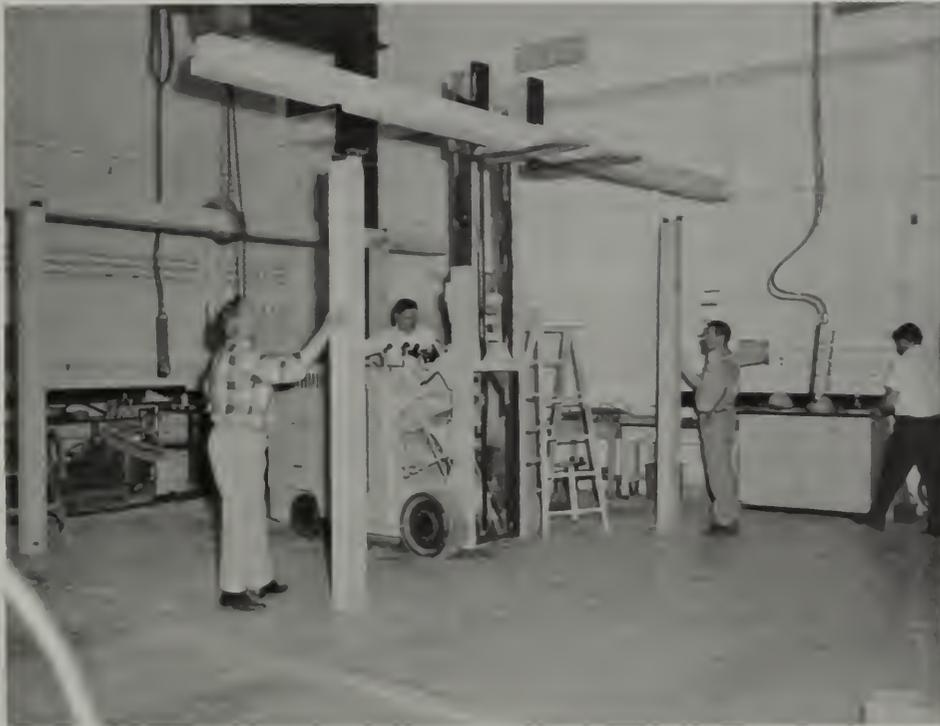
Fig. 5.3 Assembling of structural frame components
