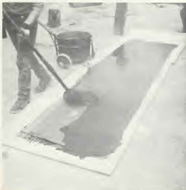
FIGURE 2. Application of hot asphalt to felt.
