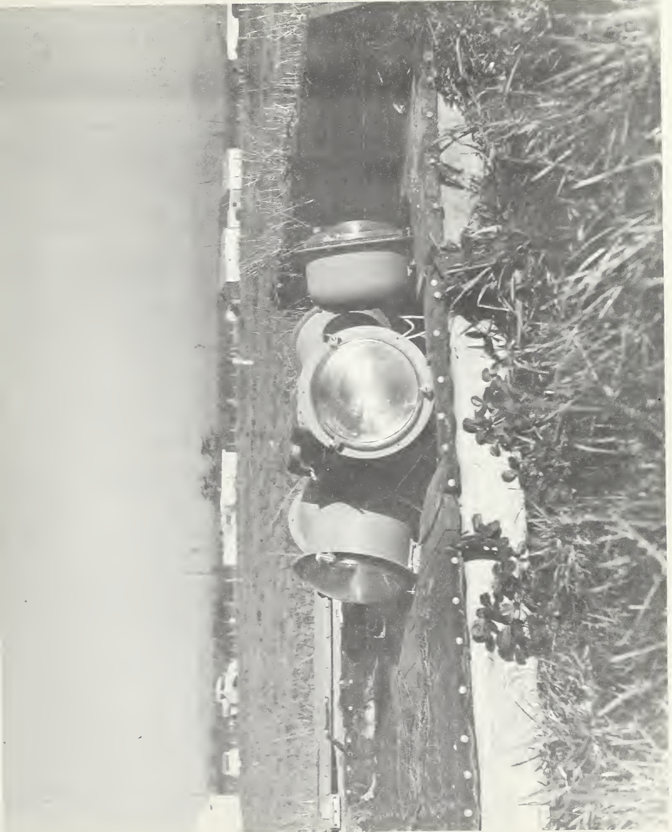
Figure 1. The stub approach beacon and shield.
